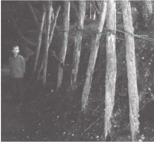
ILLUS 11 A well-preserved section of the anti-tank barrier near its western end, with surviving upright timbers held in place at the top of the bank by loops of galvanized wire
