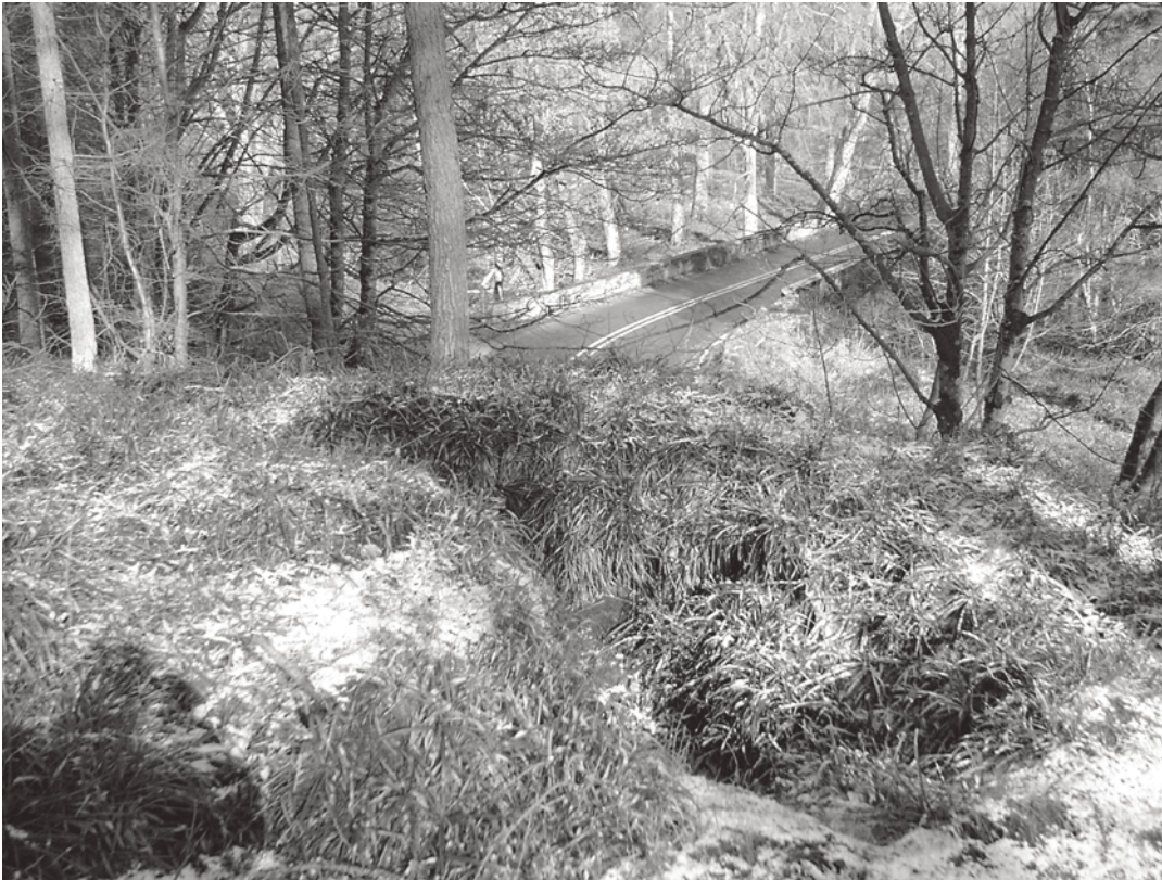
ILLUS 22 One of the slit trenches at Findlaystone, from the east
