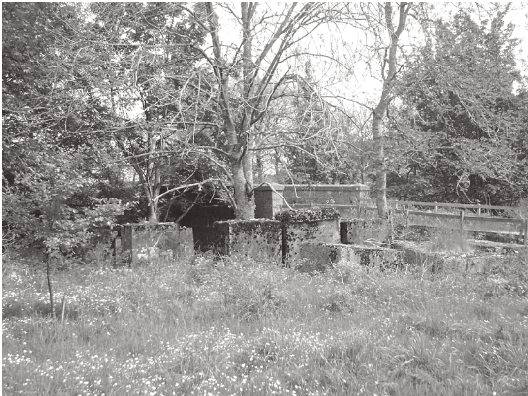
ILLUS 14 Haugh Head Bridge showing cubes
