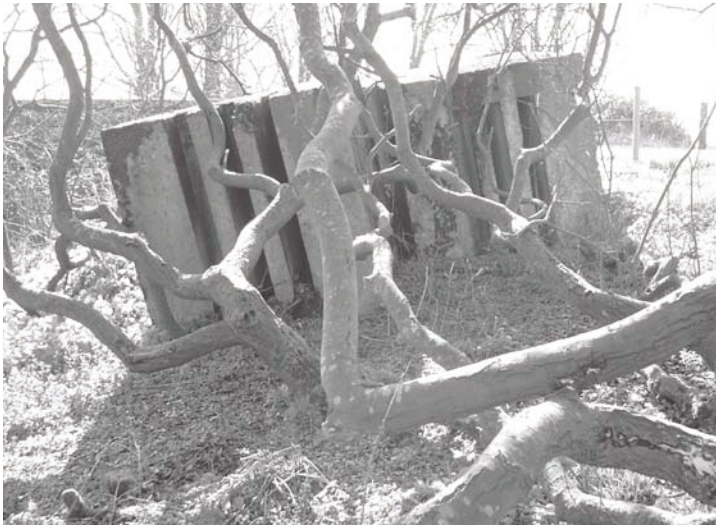
ILLUS 25 Socketed concrete blocks originally forming roadblock on the Glen Ury viaduct
