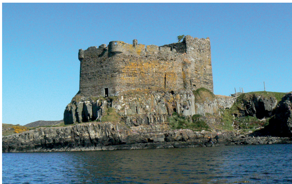
ILLUS 2 The castle on its rock, showing the sea gate and battlements with their two bartizans at the seaward angles of the curtain wall (photo: Jonathan Haylett)
