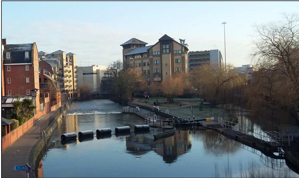
Figure 50. A pound lock (County Lock) on the River Kennet in Reading town centre
