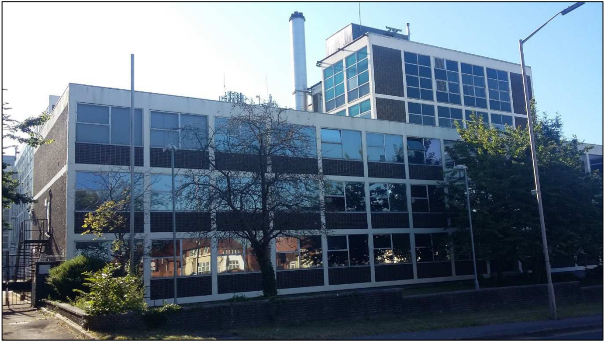
Figure 77. Telephone Exchange, Basingstoke Road, Reading
