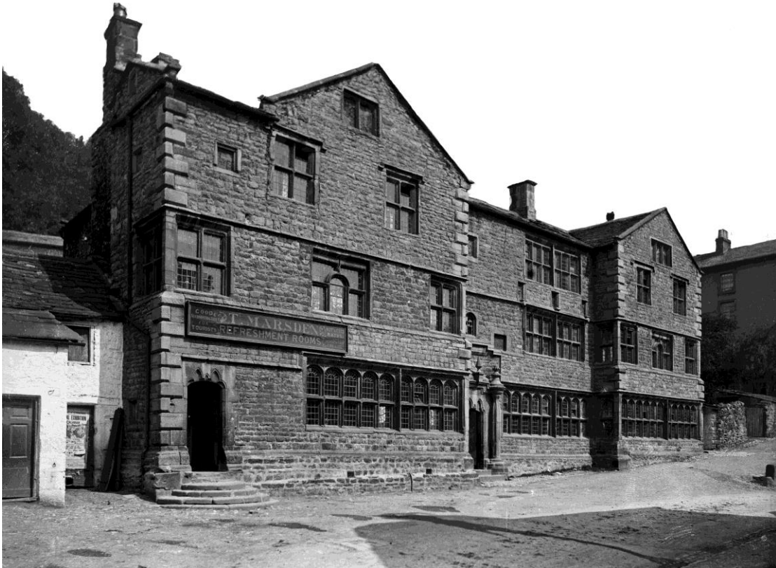
Figure 31 The Folly, Settle, photographed in 1897. Historic England Archive
