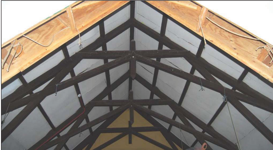
Plate 5: Roof Trusses of Nave
