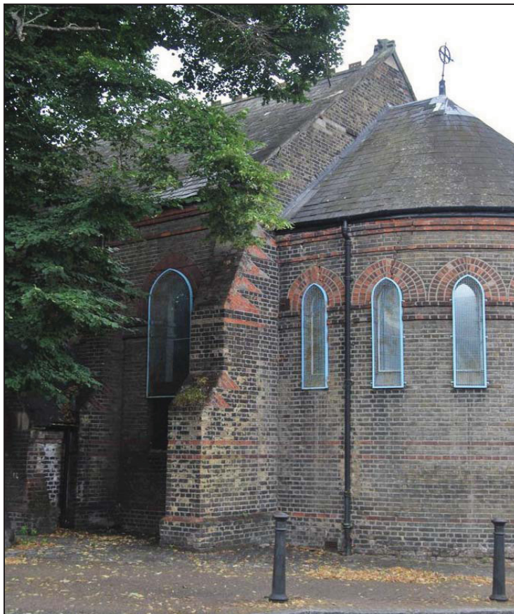
Plate 3: External View of Church
