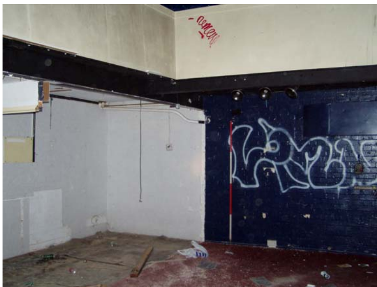
Plate 2: The Operations Block
