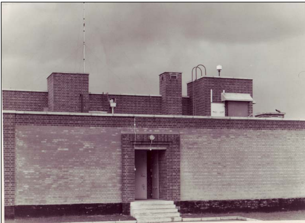
Plate 15: P1034. 1963. Exterior of protected control. Includes doorway and radio mast
