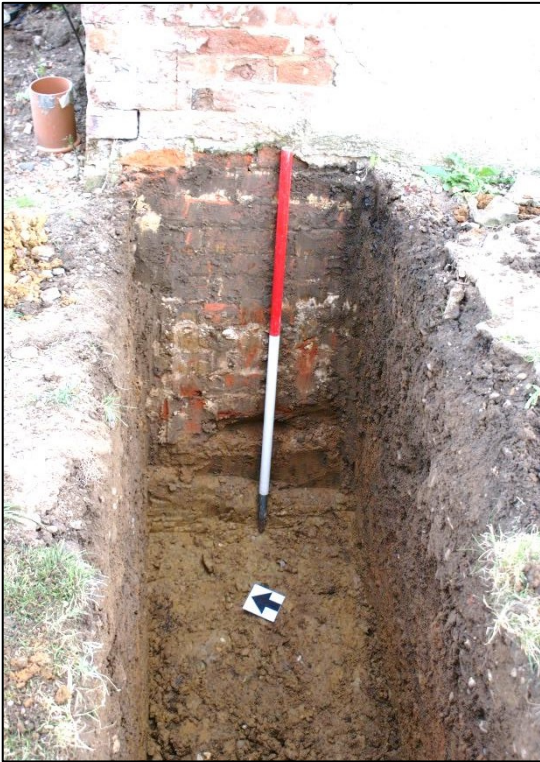
Figure 9 (left). View of the wall foundation of the southern wing of the present building, looking north-east
