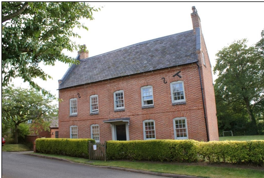
Figure 4. The main wing of Manor Farm, showing the symmetrical frontage and brick key blocks to the windows, features of this 18th century building.
