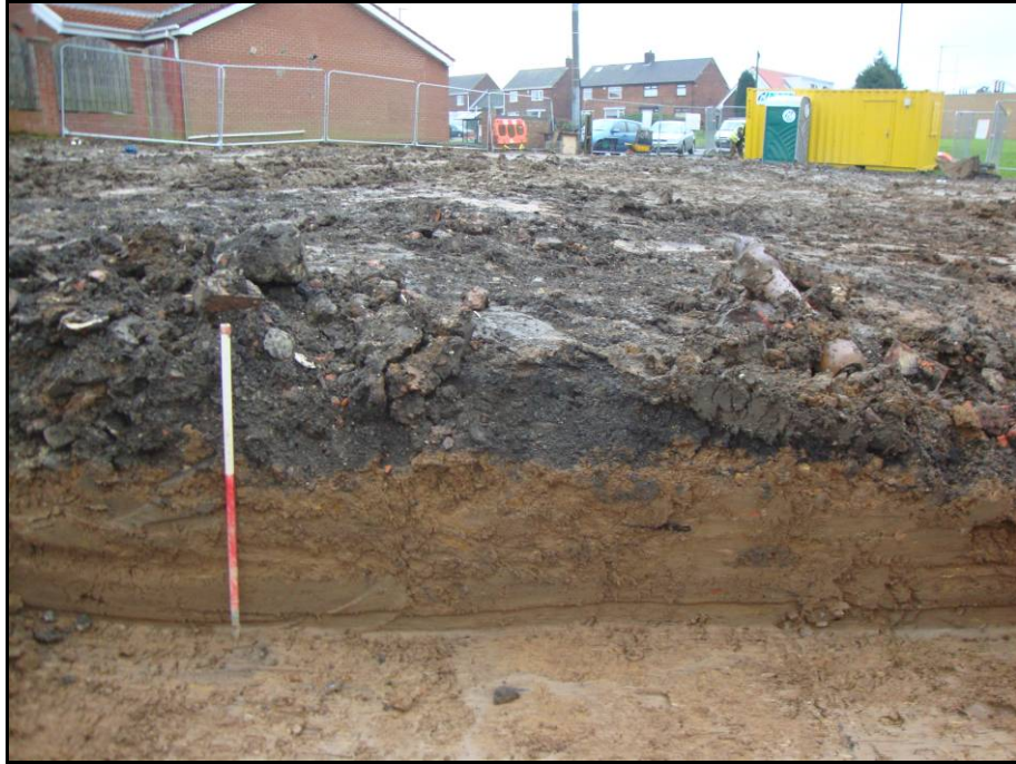
Figure 3. WNW facing section through made ground deposits (101), (102) and natural clay deposit (103). Scale 1 x 1m.
