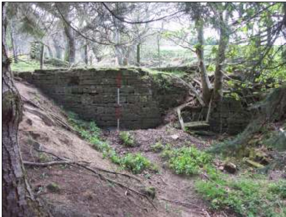
Fig. 28 Feature 028 flat topped culver: scale = 2m
