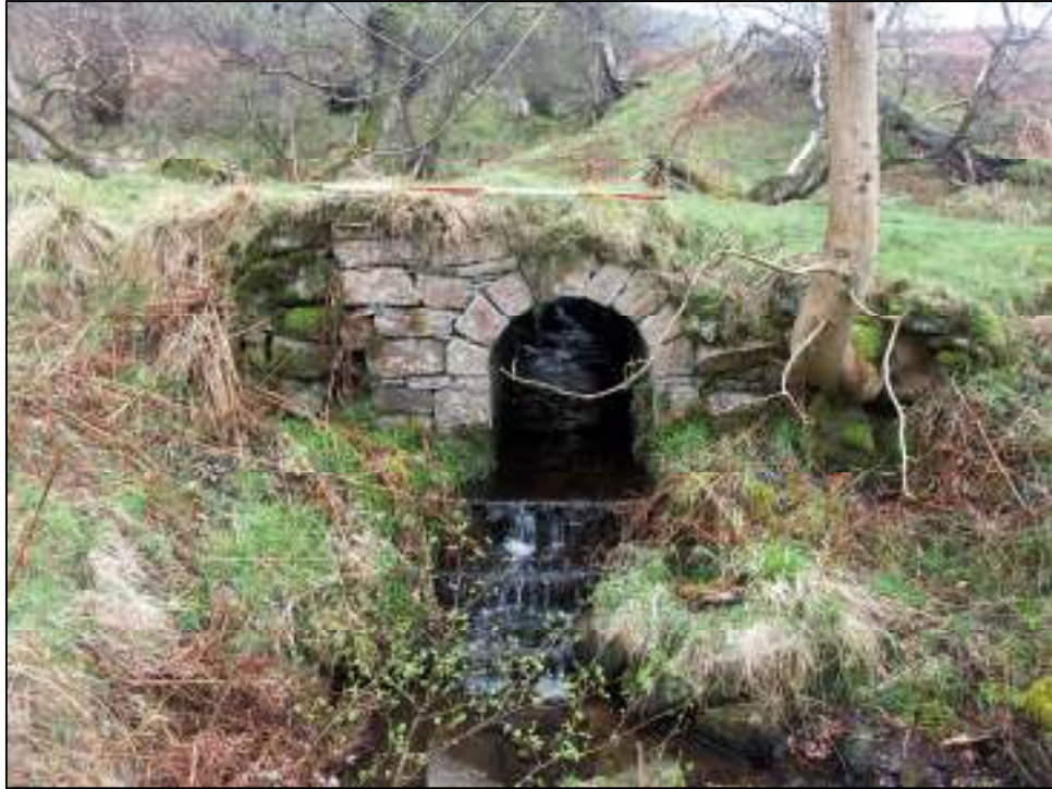
Fig 22. Feature 031 arched culvert: scale = 2m
