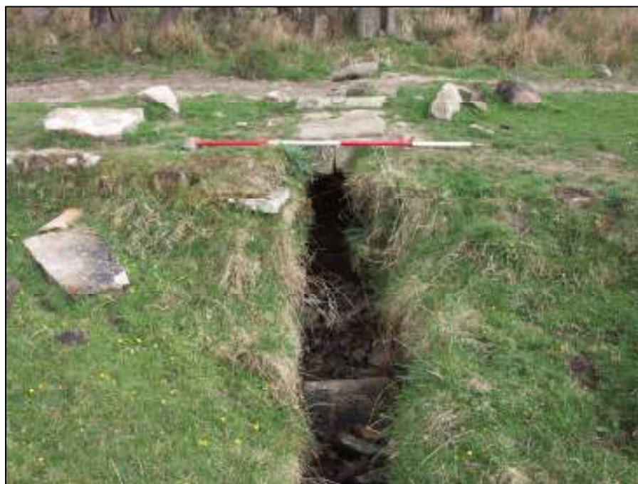
Fig. 27 Feature 019 flat topped culvert: scale = 2m
