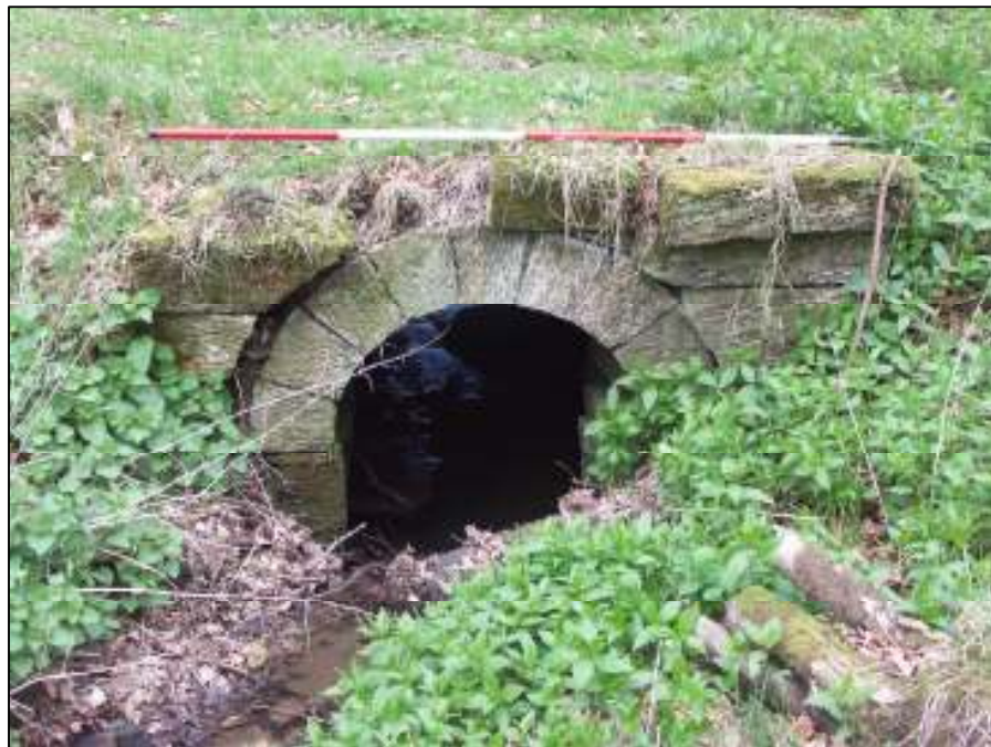
Fig. 26 Feature 029 arched culvert: scale = 2m
