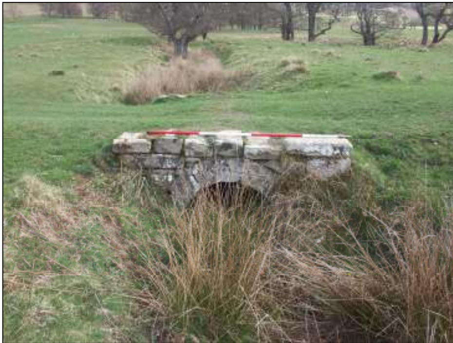
Fig. 25 Feature 020 arched culvert: scale = 2m
