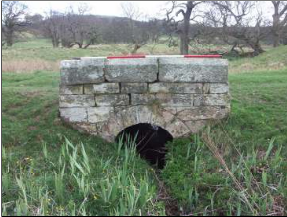
Fig. 24 Feature 021 arched culvert: scale = 2m
