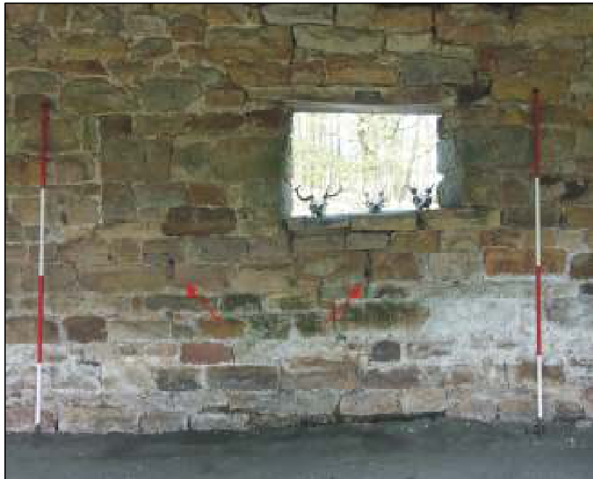
Fig. 36 Interior of Deer Hemmel, with blocked off window and slots to accommodate manger shown by arrows: scale = 2m
