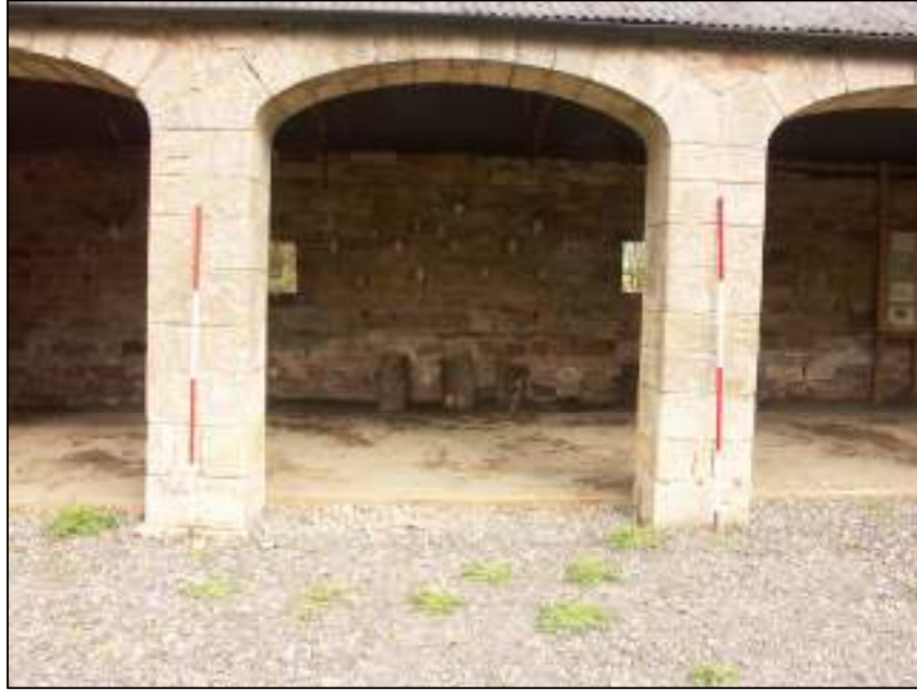
Fig. 35 Arched entrance of ashlar blocks situated on south of Deer Hemmel: scale = 2m
