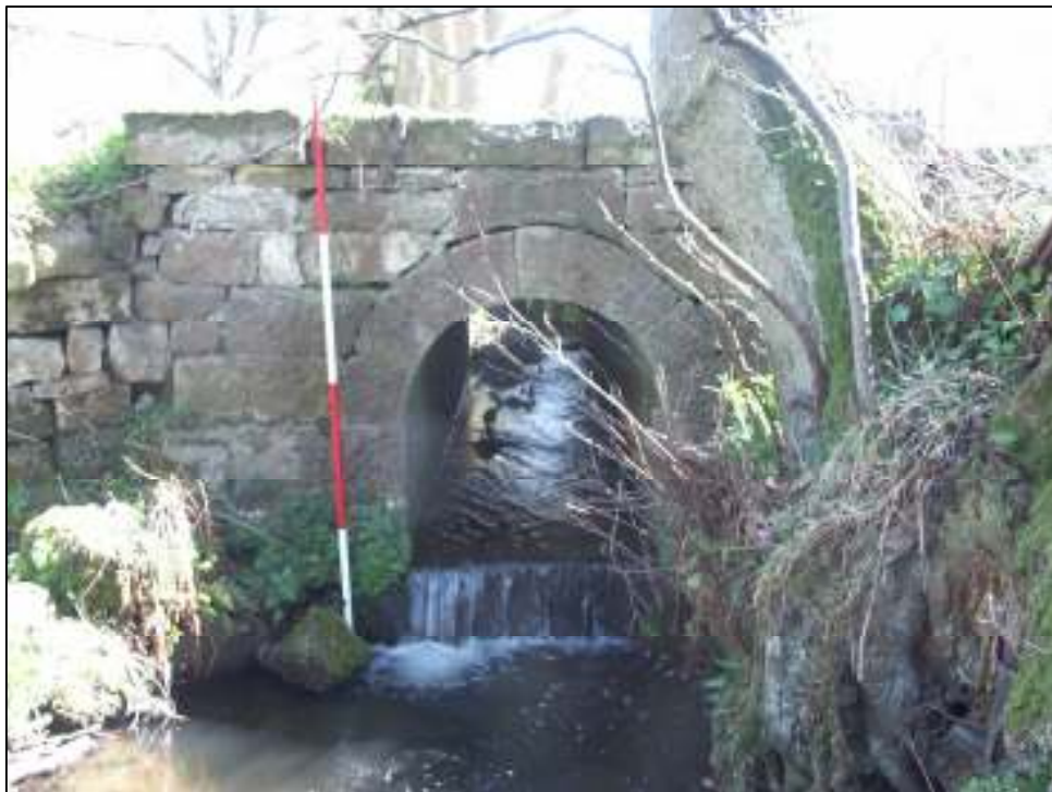
Fig. 23 Feature 017 arched culvert: scale = 2m
