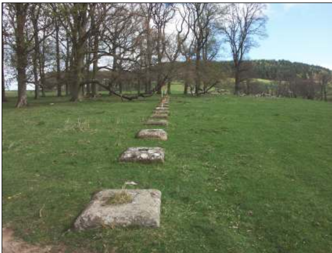
Fig. 31 Sandstone supports looking north-east: scale = 2m
