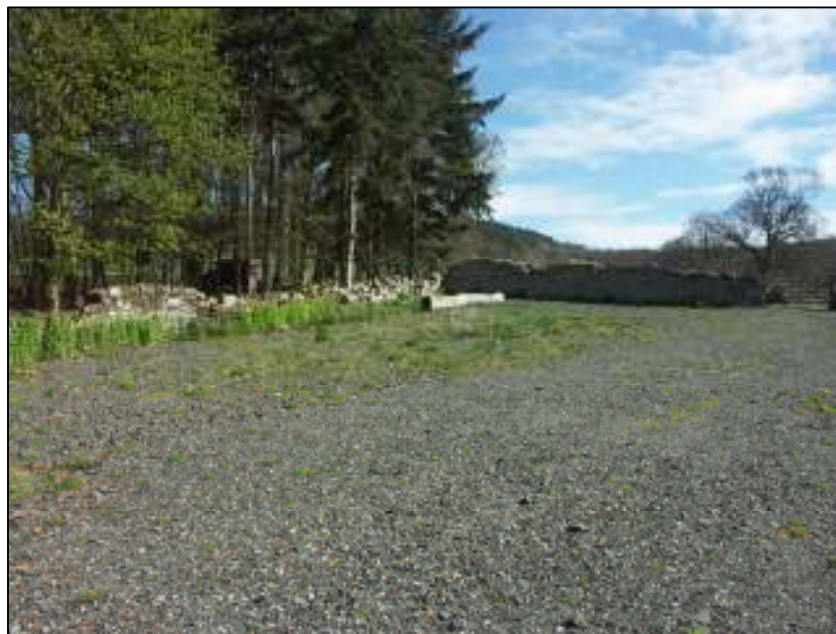
Fig. 37 Old Boundary Wall (F016) situated on right adjoining gate: scale = 2m
