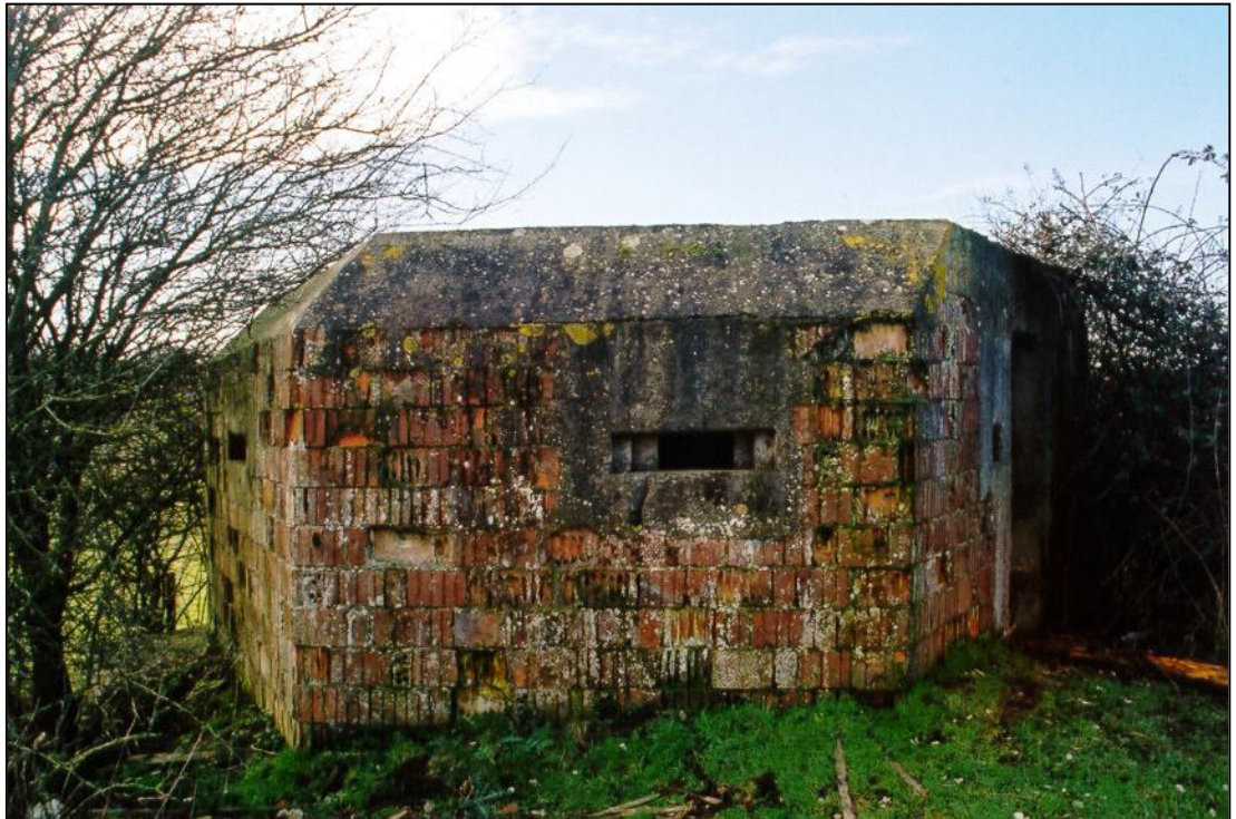
Fig. 8 - UORN 200: brick-shuttered type 24 infantry pillbox built by the tracks of the former railway line. It faced south towards Whaddon and the junction of the two branches (Green and Blue) of the GHQ Line.
