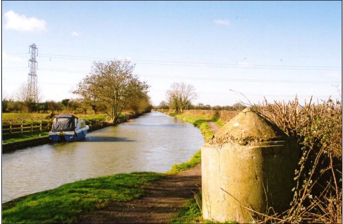
Fig. 10 - UORN 8683: conical-topped cylinder, made from a section of concrete drain pipe, by the Kennet and Avon Canal.
