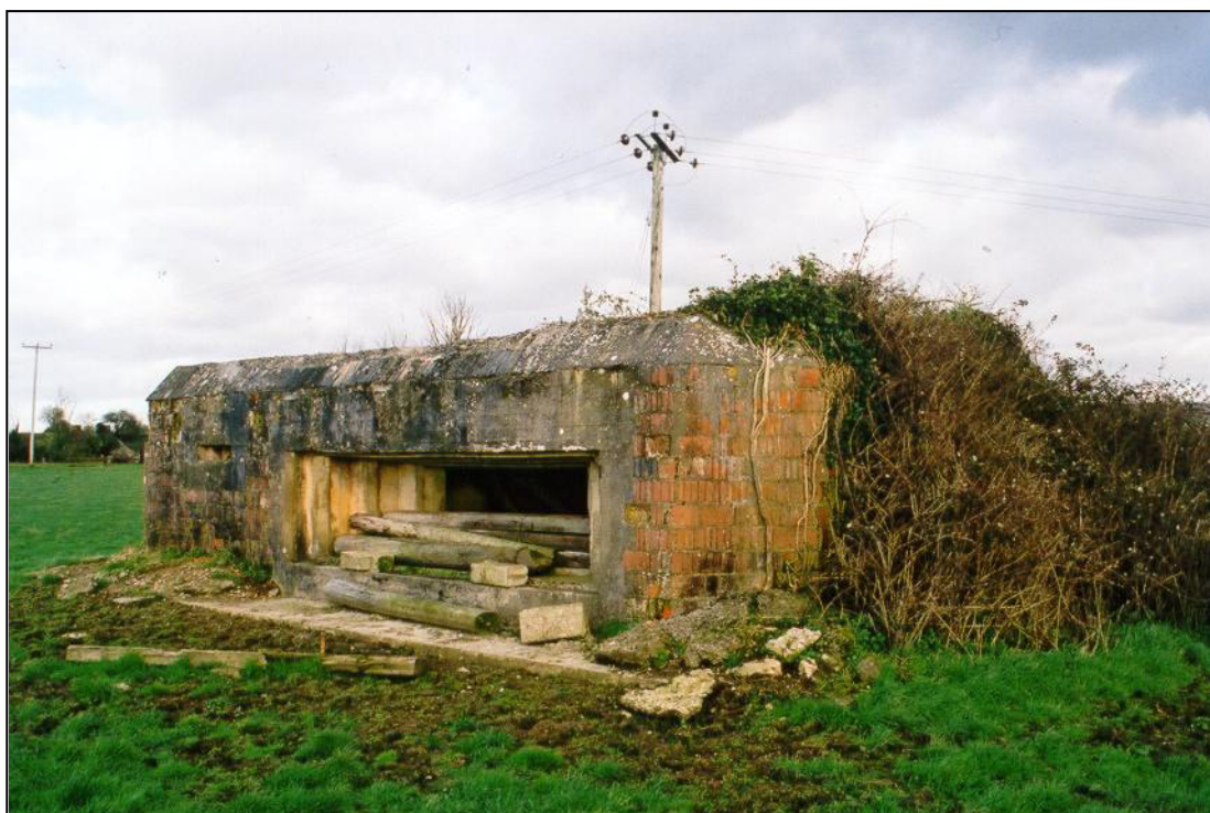
Fig. 6 - UORN 8679: massive two-chamber type 28a anti-tank gun emplacement, one of seven surviving examples in the defence area.
