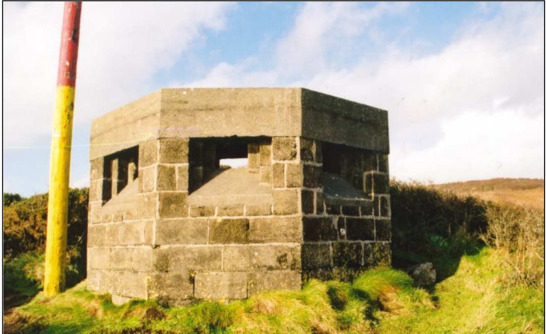
Fig. 8 - UORN 3191: pillbox made of concrete blocks, with an open rear chamber for anti-aircraft fire.
