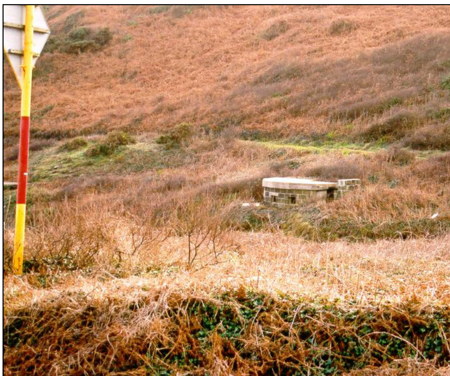
Fig. 6 - UORN 3272: looking at the east facing embrasures of this unusually shaped pillbox, built of concrete blocks. It stands at the edge of a slope. [see as well Fig. 7].
