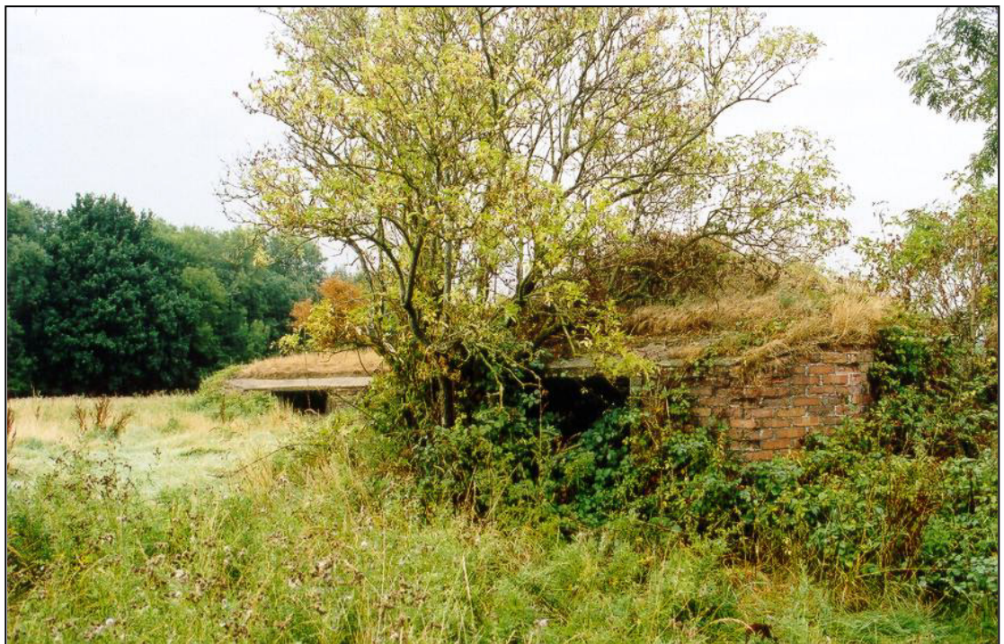
Fig. 7 - UORNs 16741 [left] and 16742. These Vickers machine gun emplacements were angled to each other so that their fire converged.
