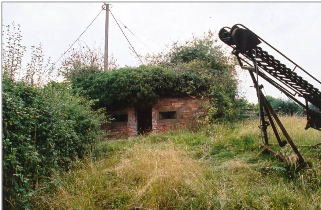
Fig. 13 - UORN 9827: the doorway and rear-facing embrasures of the type 24 pillbox next to Homecroft Farm in Ewshot village.
