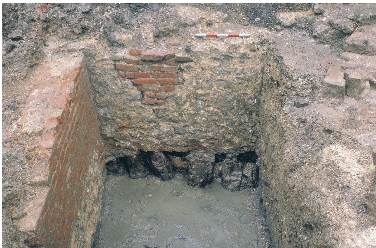
Fig. 3: medieval wall supported on timber piles
