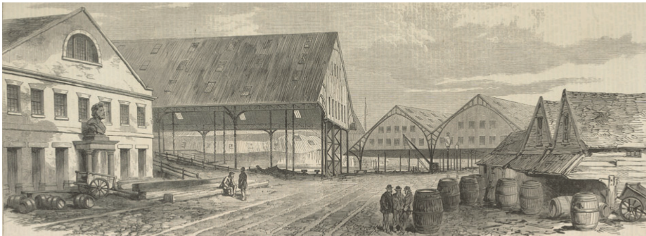
Fig. 19: Baker’s iron roofs over Slipways Nos 1, 2 and 3 engraving of 1869 (© British Library Board ADD MS 32360)
