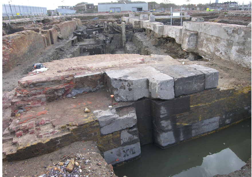
Fig. 15: Stone Basin entrance of c. 1814 with depth gauge (© MOLA)
