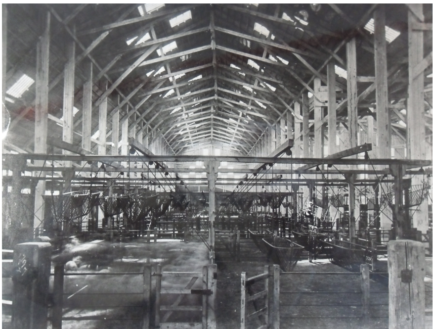
Fig. 23: interior of wooden cover building over slipway No 5, c. 1880 (© Courtesy of Lewisham Local History and Archives Centre Thankfull Sturdee Collection PH 71-4158 LS34)
