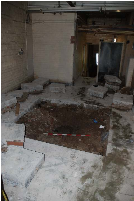
Fig 17 General view of Trench C looking southeast towards the rear of the site. The upper concrete slab has been removed and the trench measures 2.04m x 2.10m in plan. The compacted rubble layer can be seen. (Scale:1m).
