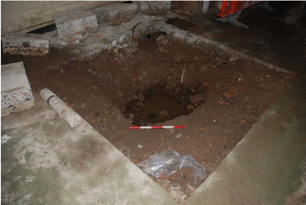
Fig 20 Trench C after diamond drilling through the rubble and lower slab.
