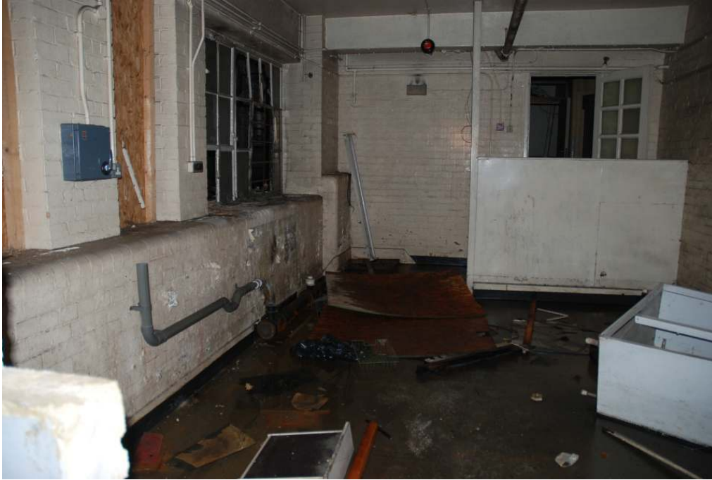
Fig 16 General location of Trench C in the centre of the site, looking west towards the York Road frontage.
