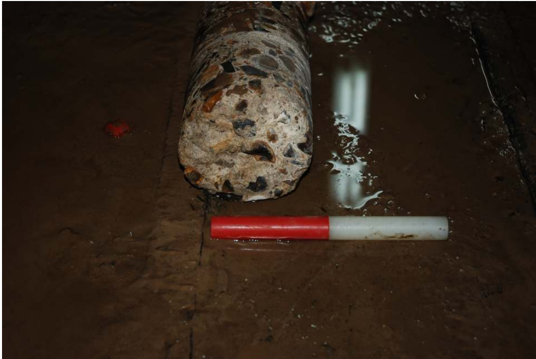
Fig 26 The broken end of the core from Trench D (Scale 20 cm)
