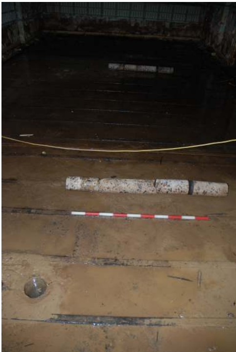
Fig 25 Core for Trench D looking south. The core for this Trench measured 1.3m in length and was reinforced from a depth of 1.24. However, on extraction the base of the core broke (200mm) and fell back into the hole. The actual depth of the concrete slabs in this area of the site, included the loose concrete rubble below, was actually probably about 1.7m. This would still give an underside of concrete level of between -1.066m OD.
