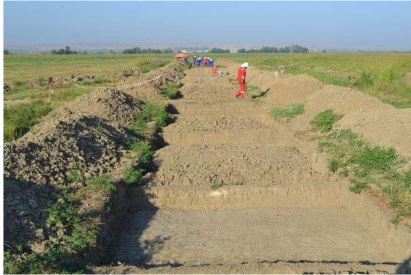
Figure 2. General view of excavation, view to west
