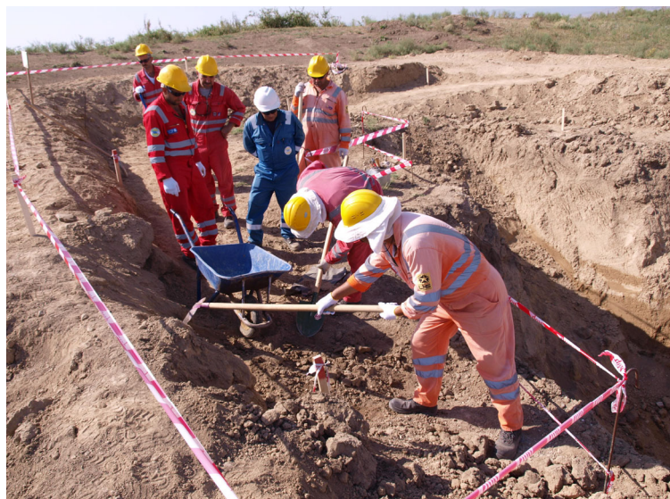
Figure 3. View of excavation area. View to west.
