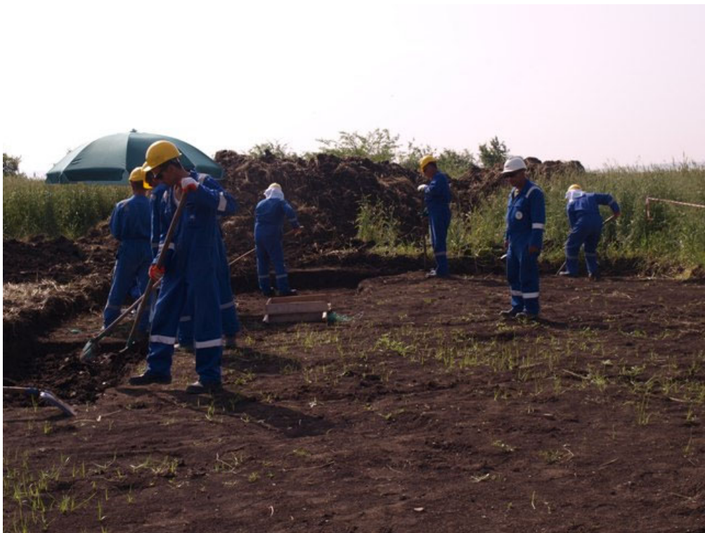
Photo 2. View of excavation area.
