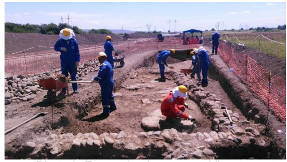
Photo 8. Excavation in process. View to east
