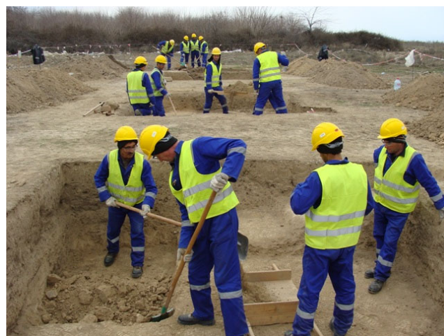
Photo 5. Area 2 excavation process in Unit 22, view to west.
