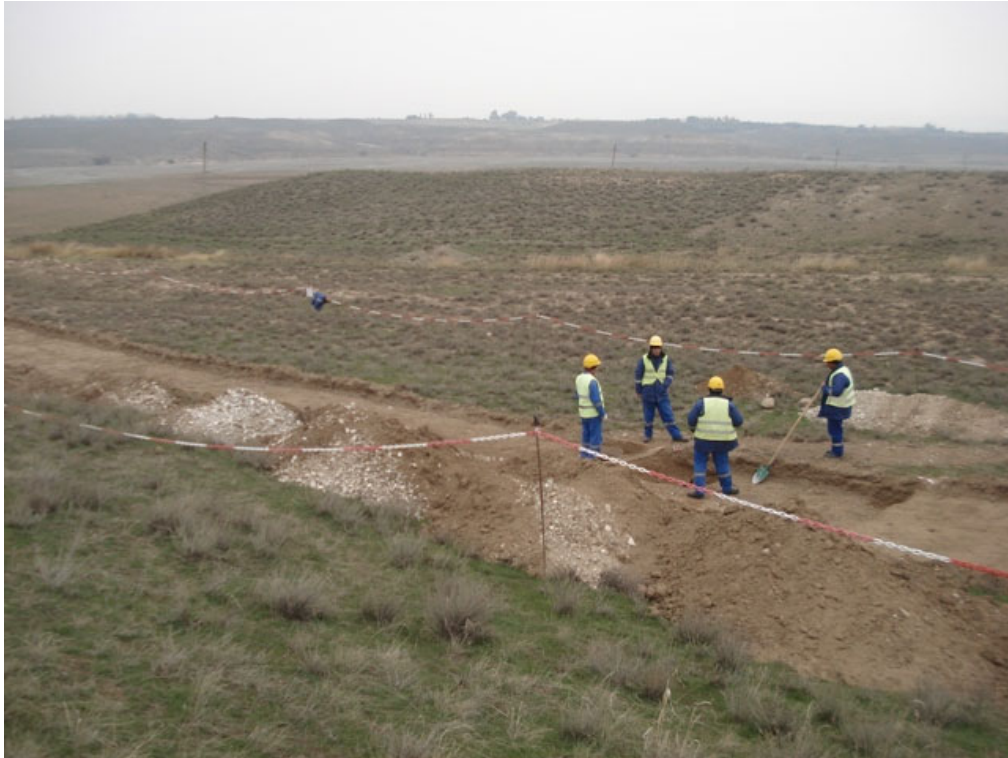
Photo 2. View of excavation. View to north. The prehistoric cemetery excavated in 2003 lies to the right on the low ridge in the foreground.
