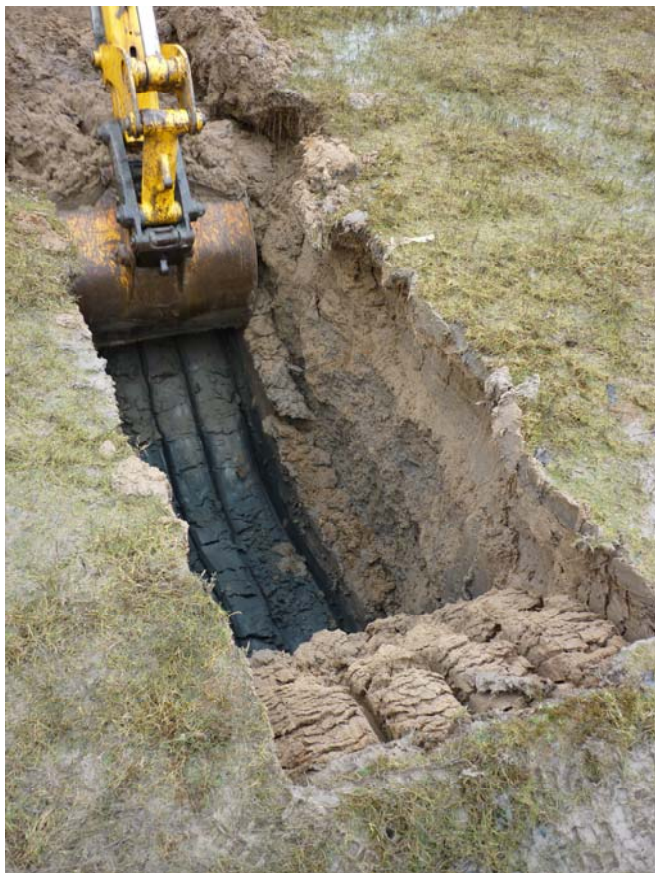
Plate 3 (left): Dark grey silts present in trial pit/borehole 03
