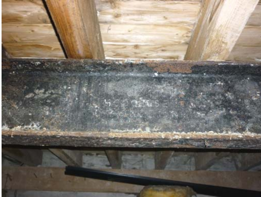
Plate 19: Iron girder supporting ceiling of Room 2
