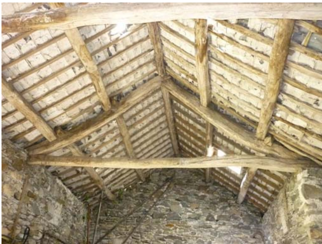
Plate 13 (left): General view of southern roof truss
