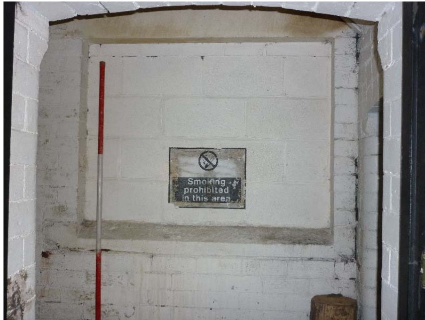
Plate 36: Blocked window in the east elevation of Basement 8, showing the curvature of the arched doorway from Basement 6
