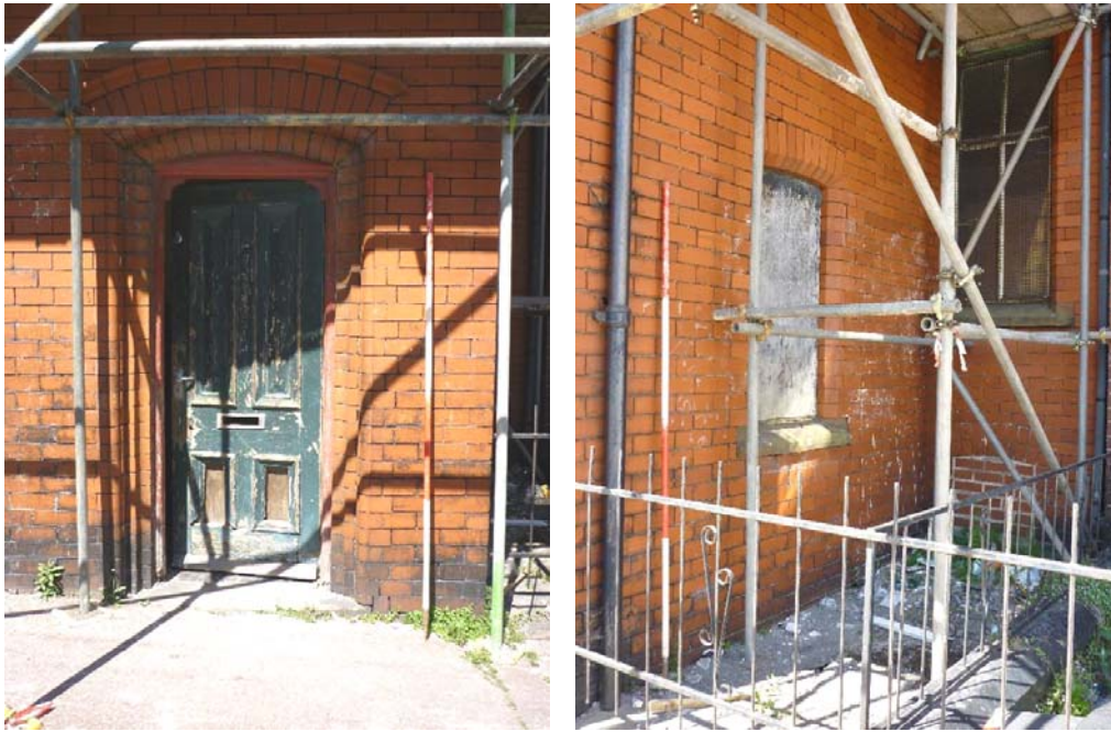
Plate 23 (left): Porch doorway in the south-east elevation
