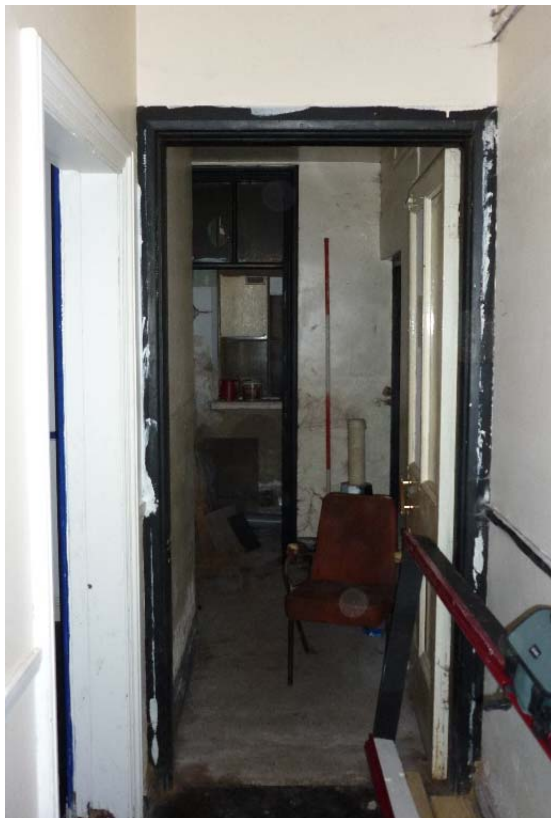
Plate 35: View through to Basement 7 from the main corridor, Basement 2
