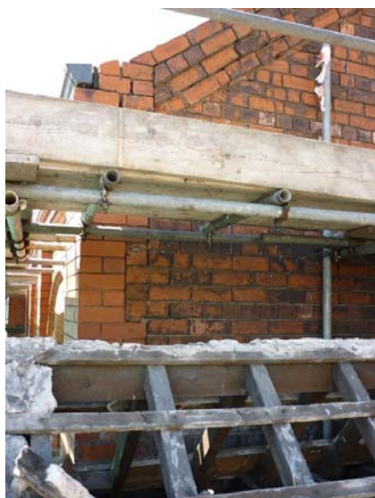
Plate 21 (left): Junction between the machine-made bricks of the south-east elevation and the rougher bricks of the north-east
