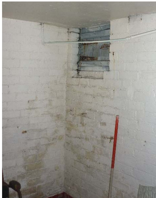
Plate 37: Hatch in the south-east corner of Basement 9
