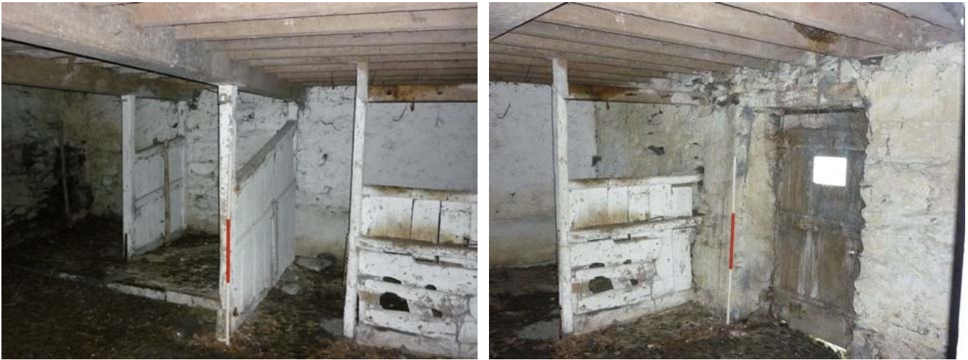
Plate 20 (left): Stalls against the south-west elevation, G3
