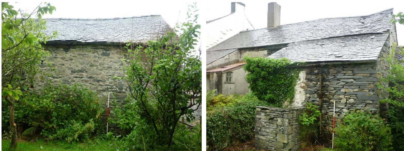
Plate 8 (left): South-east external elevation, north-east end
