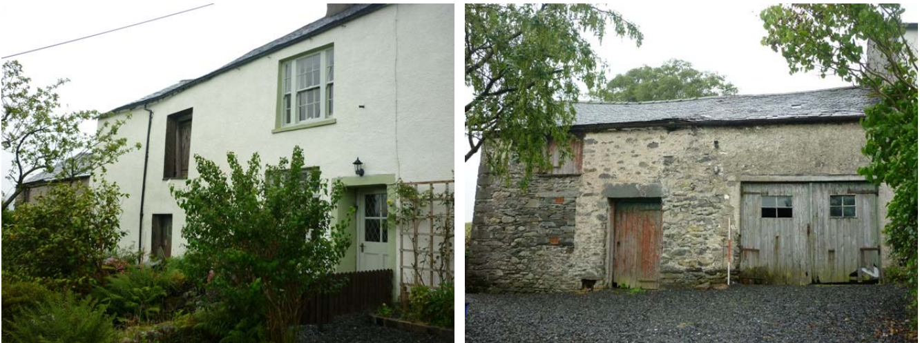
Plate 5 (left): North-west external elevation, south-east side
