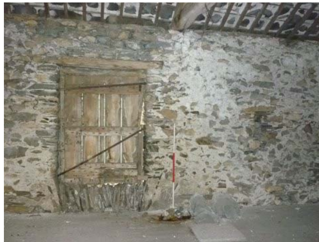
Plate 28: Doorway and ventilation slot in north-west elevation, F2
