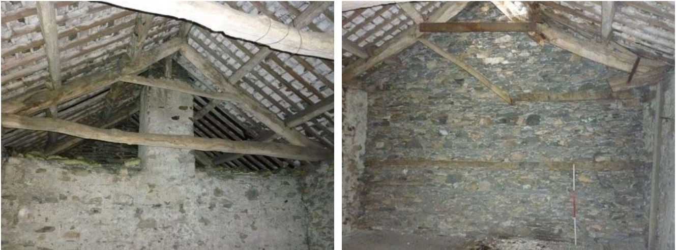
Plate 26 (left): Surviving truss on south-west side of F2
