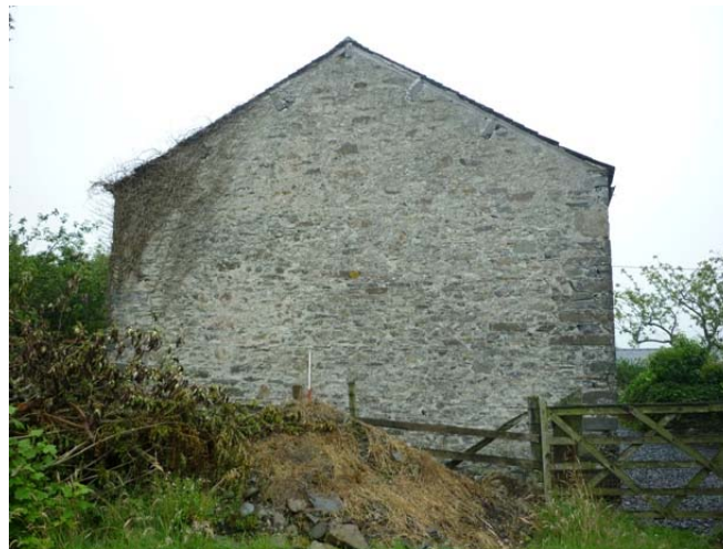
Plate 7: North-east external elevation
