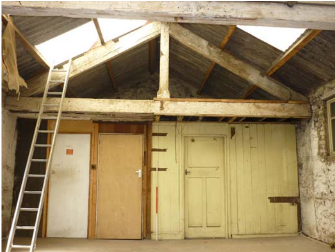
Plate 42 (Left): North truss in F2
