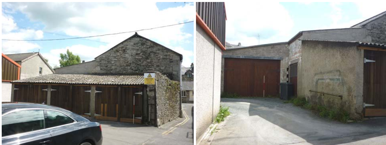
Plate 15 (left): North external elevation
