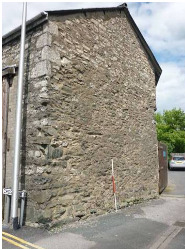
Plate 19: South elevation showing the different build between the lower and upper sections
