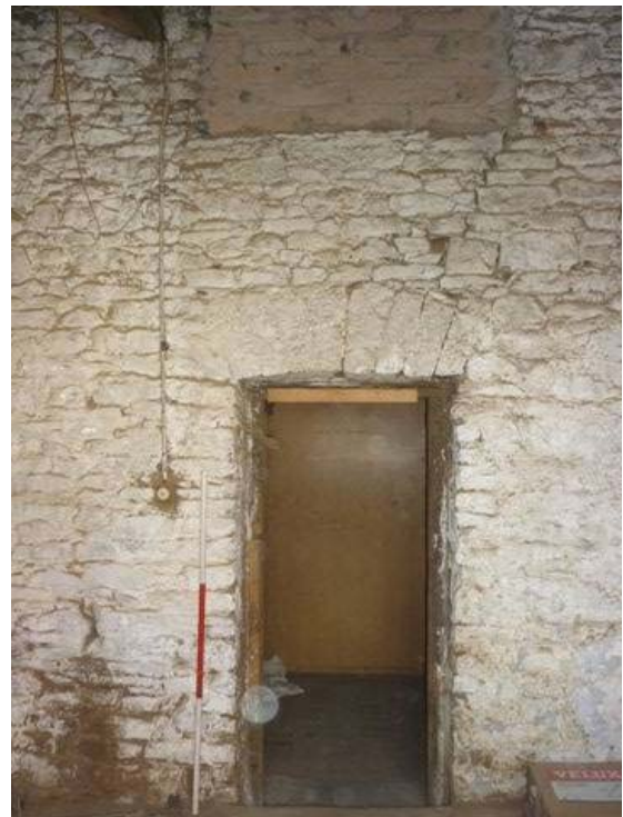
Plate 31 (right): Doorway with blocked window above at north end of west elevation, G2
