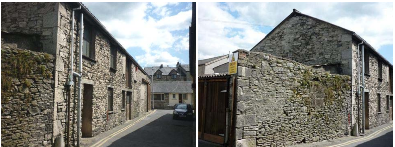
Plate 21 (left): North end of the west elevation
