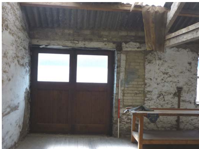
Plate 44 (right): Large doorway, south end of west elevation, F2
