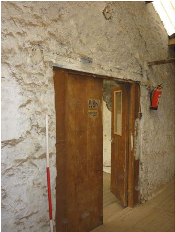
Plate 40 (left): Doorway in north elevation, F1
