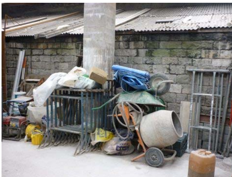
Plate 25: Stone section in centre of west elevation of G1
