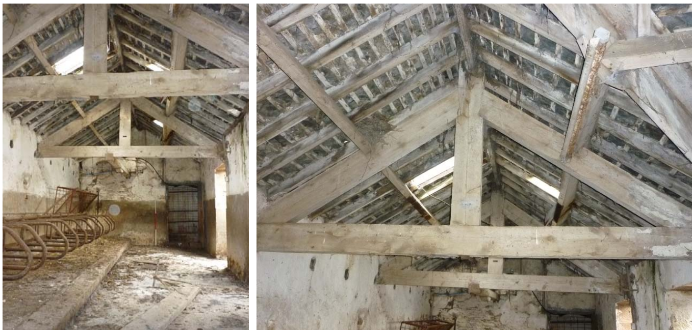
Plate 24 (left): View looking north in the north/south arm of Building 1
