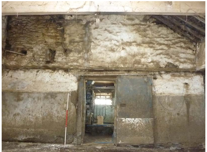
Plate 47 (left): Detail showing quoins from the original limit of the northernmost wall of Building 4
