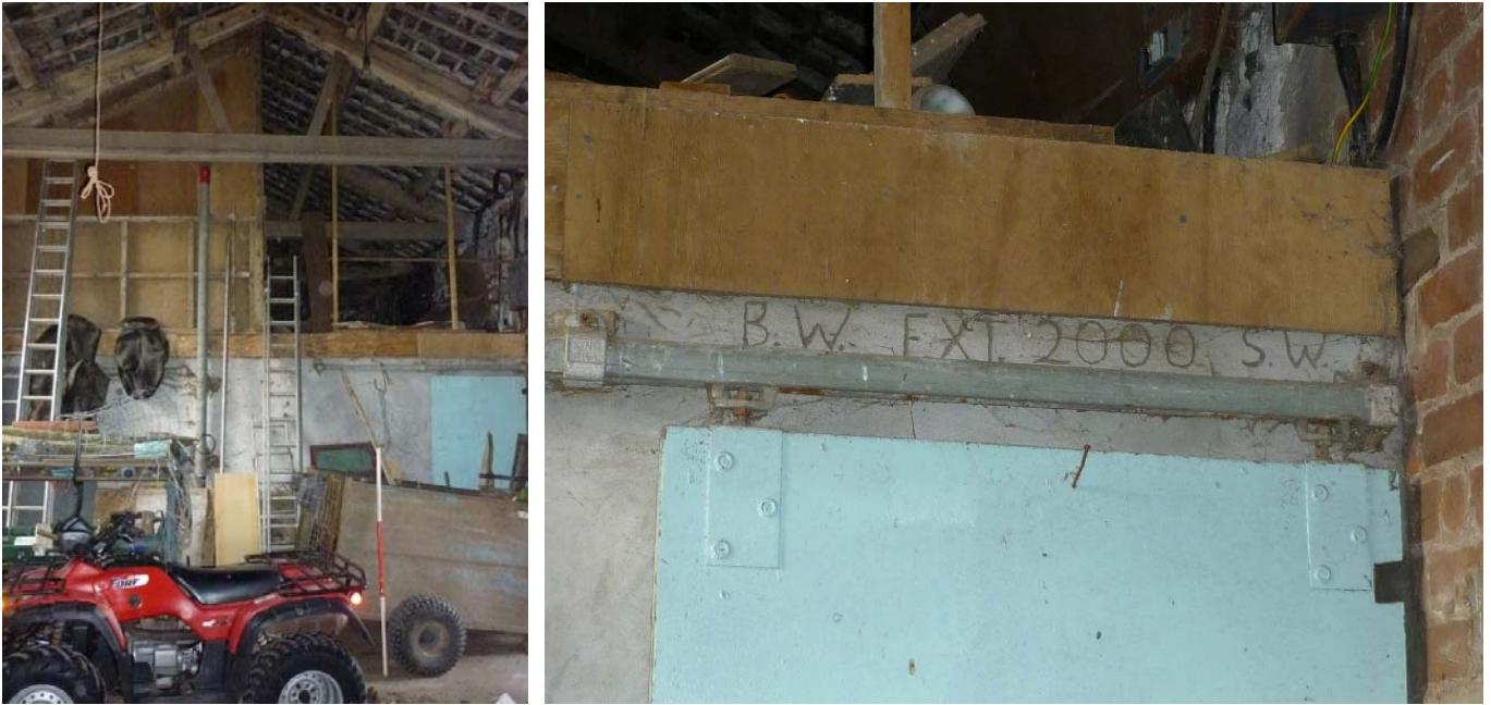
Plate 35 (left): Building 3 viewed from the east, showing the upper floor
