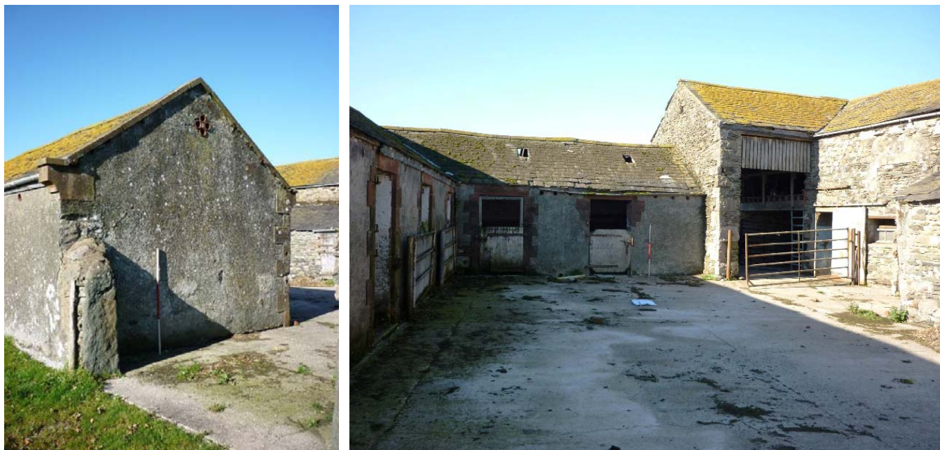
Plate 14 (left): South end of the east elevation of Building 1
