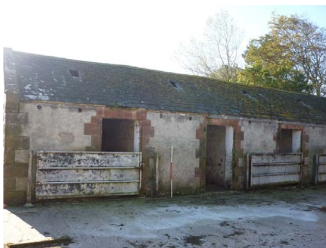
Plate 11: The north elevation of Building 1
