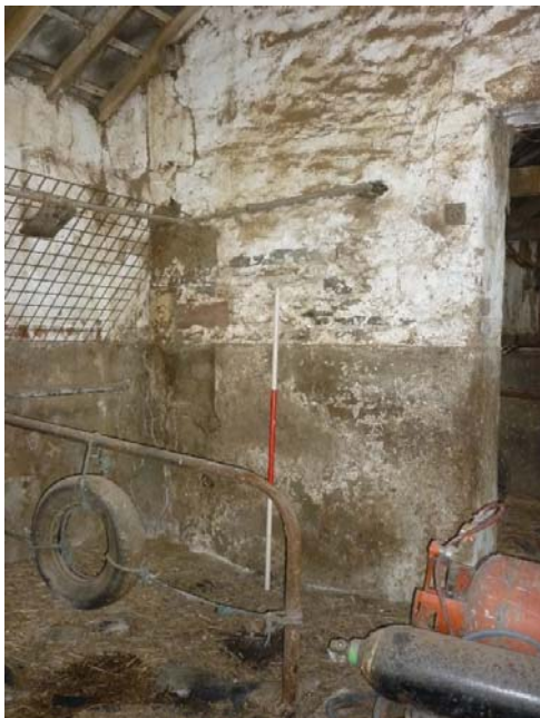
Plate 47 (left): Detail showing quoins from the original limit of the northernmost wall of Building 4
