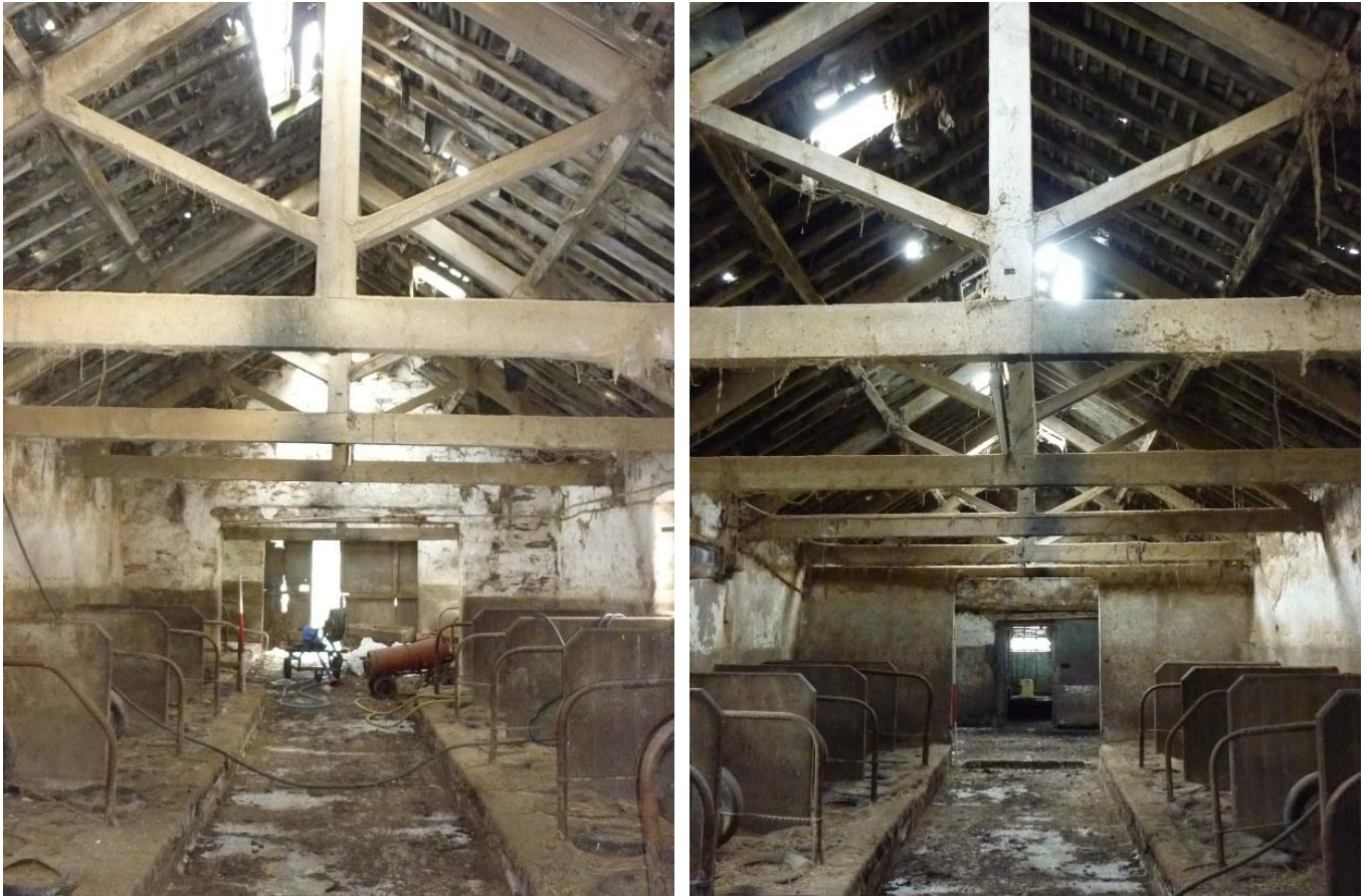
Plate 45 (left): General view of Building 4 from the south
