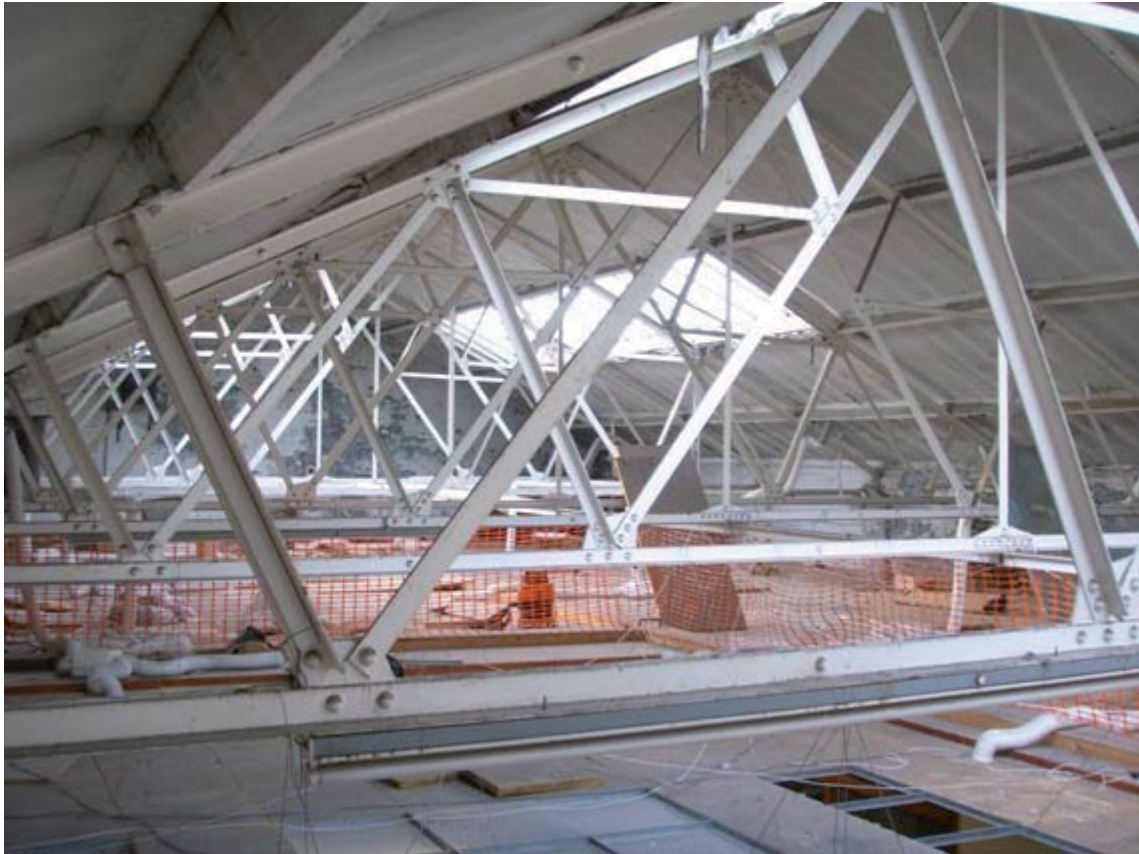
Plate 21: General view of roof trusses in the main roof space
