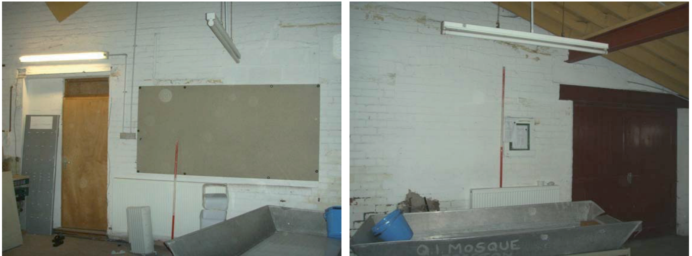
Plate 13 (left): North elevation of Room 2, showing remodelled and blocked window
