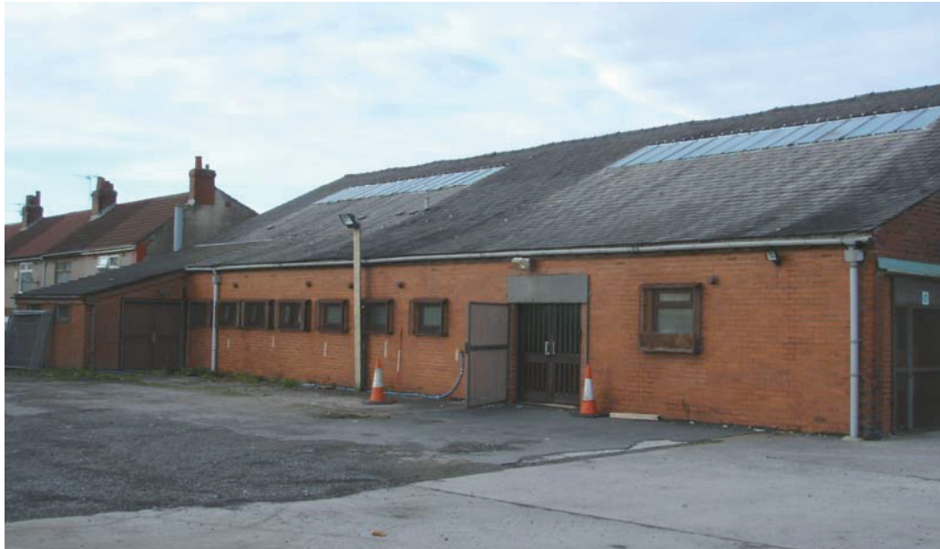
Plate 8: General view of the south external elevation
