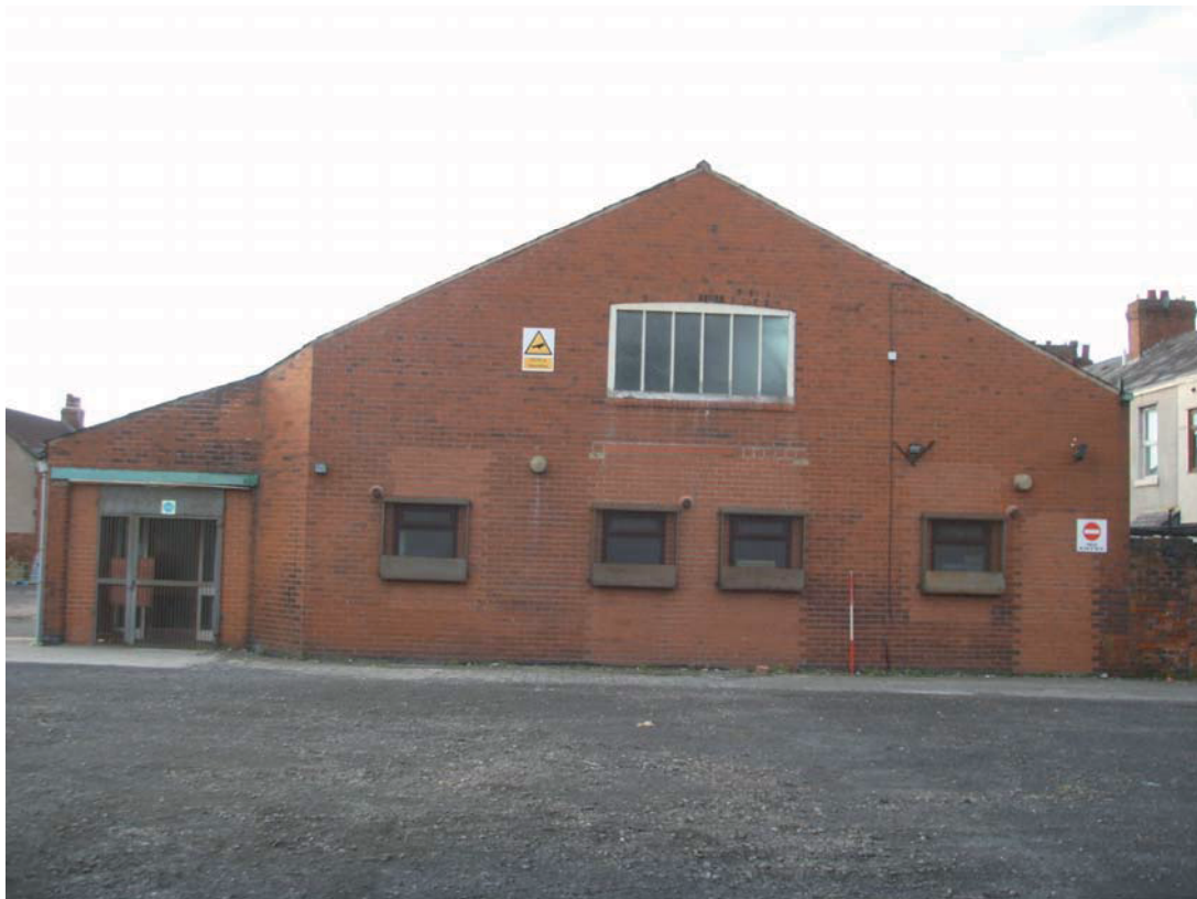
Plate 5: General view of the east external elevation
