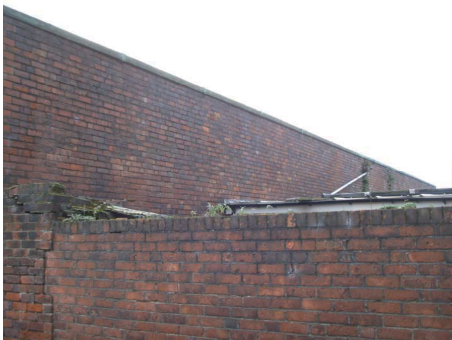
Plate 4: North external elevation from the north-east
