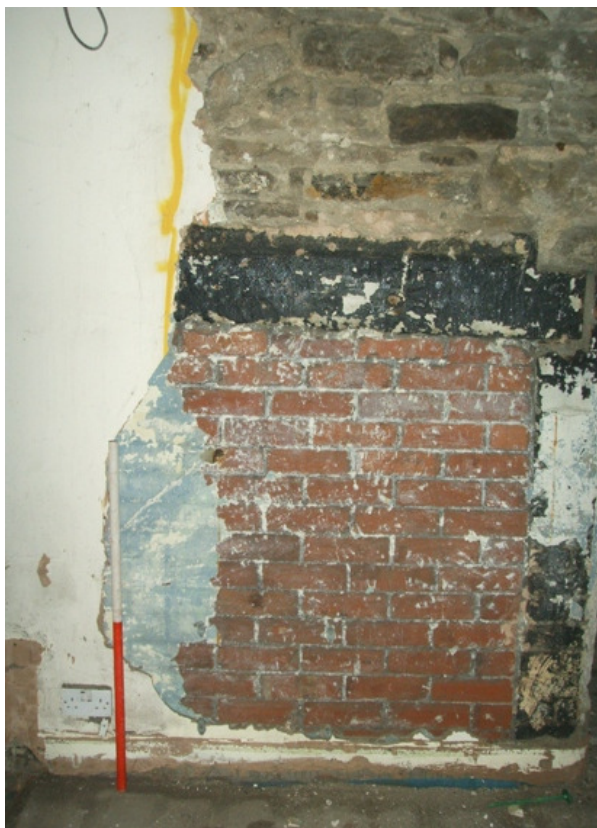
Plate 23 (left): Blocked fireplace in G10c Plate 24 (right): Detailed view of the carved letters, numeral, and symbol in the lintel (turned 90° to the left)
