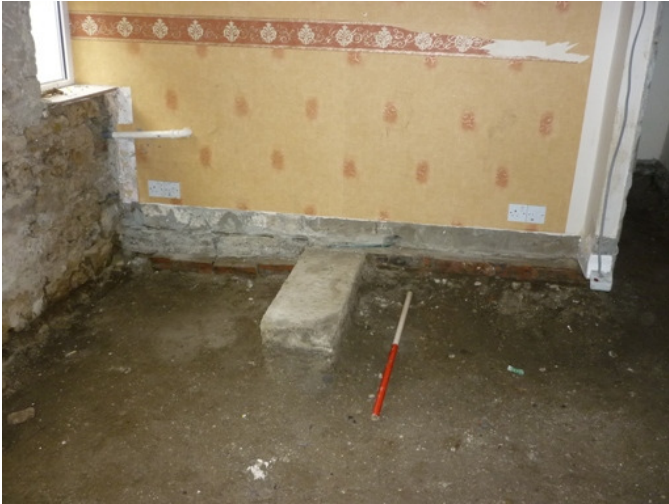
Plate 29 (left): Stone 'plinth' running beneath a partition wall in Room G13
