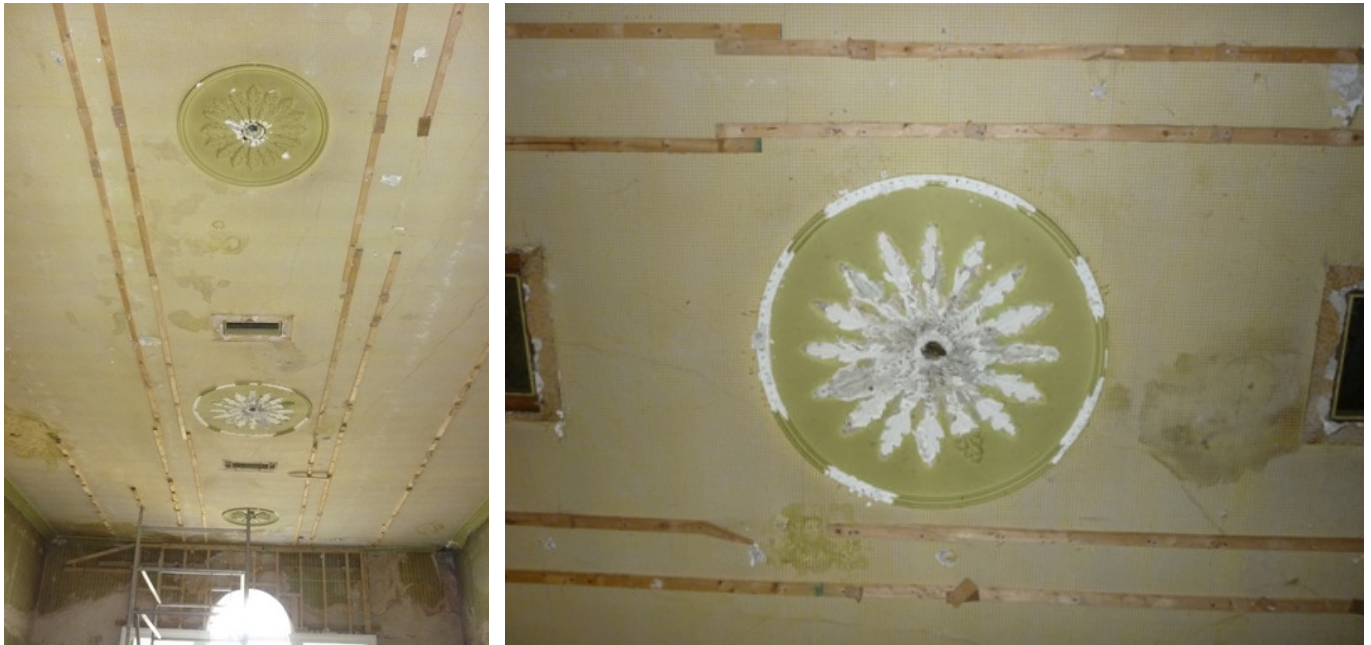
Plate 35 (left): Ceiling roses exposed in Room F6
