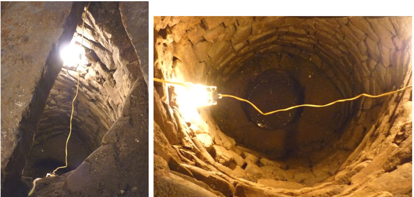
Plate 17 (left): Detail of the wall construction of the well in Room G8
