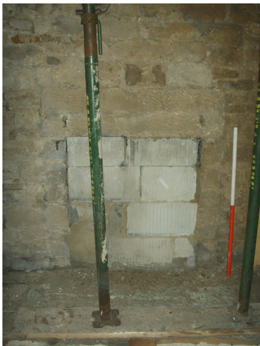
Plate 47: Blocked fireplace in south elevation of S2
