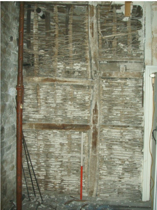
Plate 33 (left): Exposed timber stud wall in Room F3
