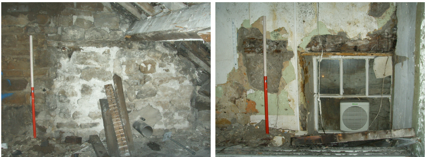
Plate 43 (left): Blocked window at west end of S1
