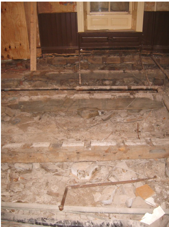
Plate 11 (left): exposed joists beneath the floor of Room G6 (photograph by Stephen Gardner)
