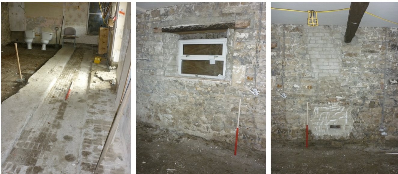
Plate 26 (left): Concrete floor revealed in Room G12
