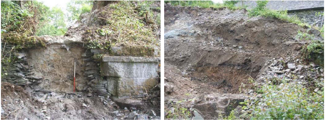
Plate 23 (left): Remains of wall with slag built against it and incorporating limestone built 'gate pier' on re-used edge-runner stone
