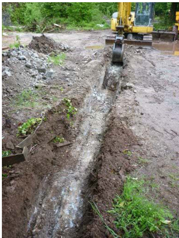
Plate 12 (left): Excavating through slag to create the service trench
