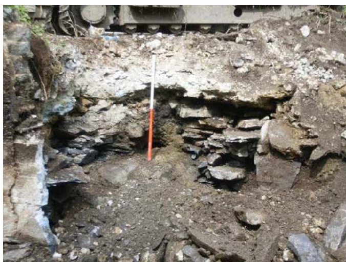
Plate 17 (left): Culvert encountered in the north-west abutment cut
