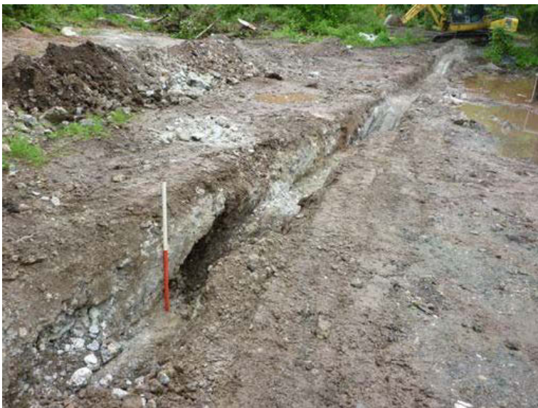
Plate 12 (left): Excavating through slag to create the service trench
