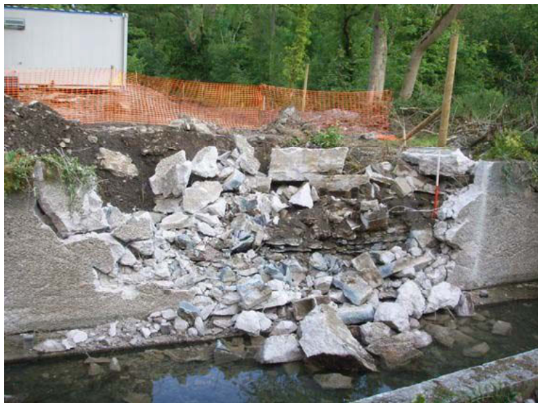
Plate 15 (left): The north-west abutment following the demolition of the leat wall
