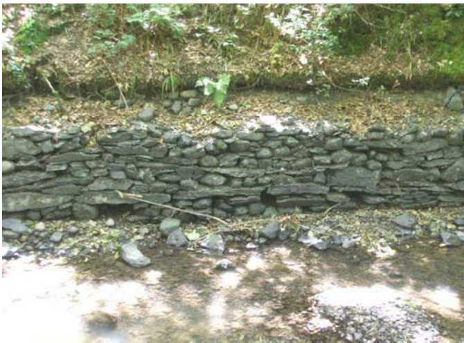
Plate 25 (left): Example of leat wall showing build Style 1
