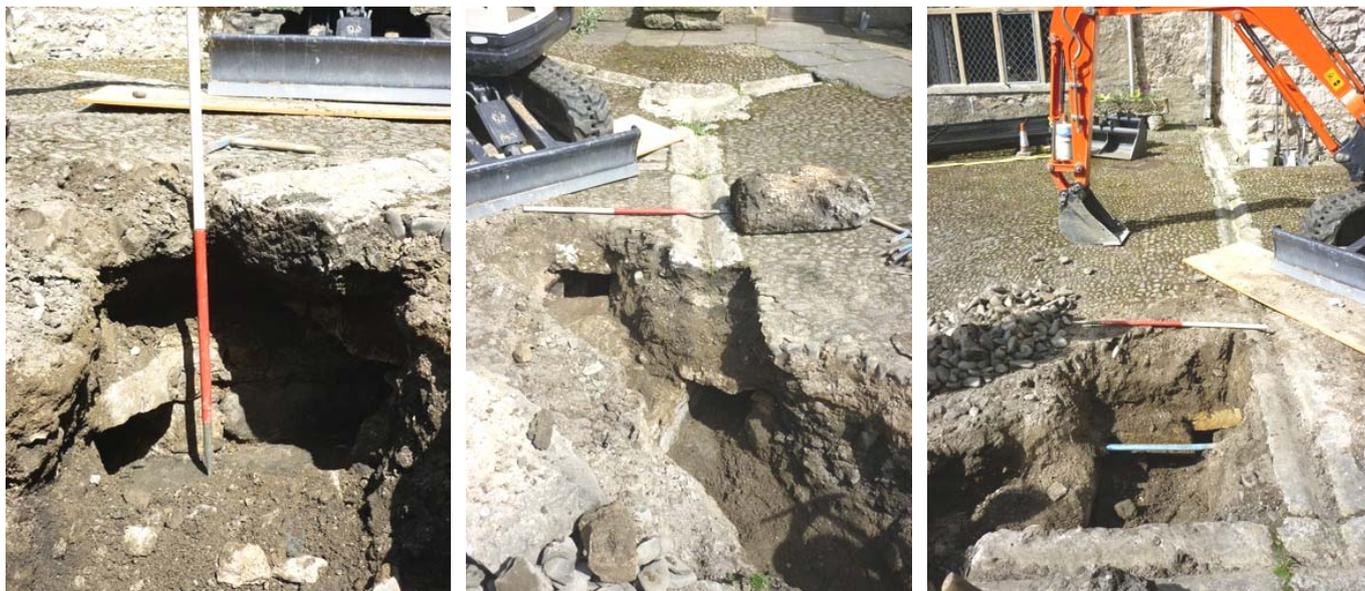
**Plate 15 (left): Stone culvert (the slate base of which is visible at the point of the scale bar)**
