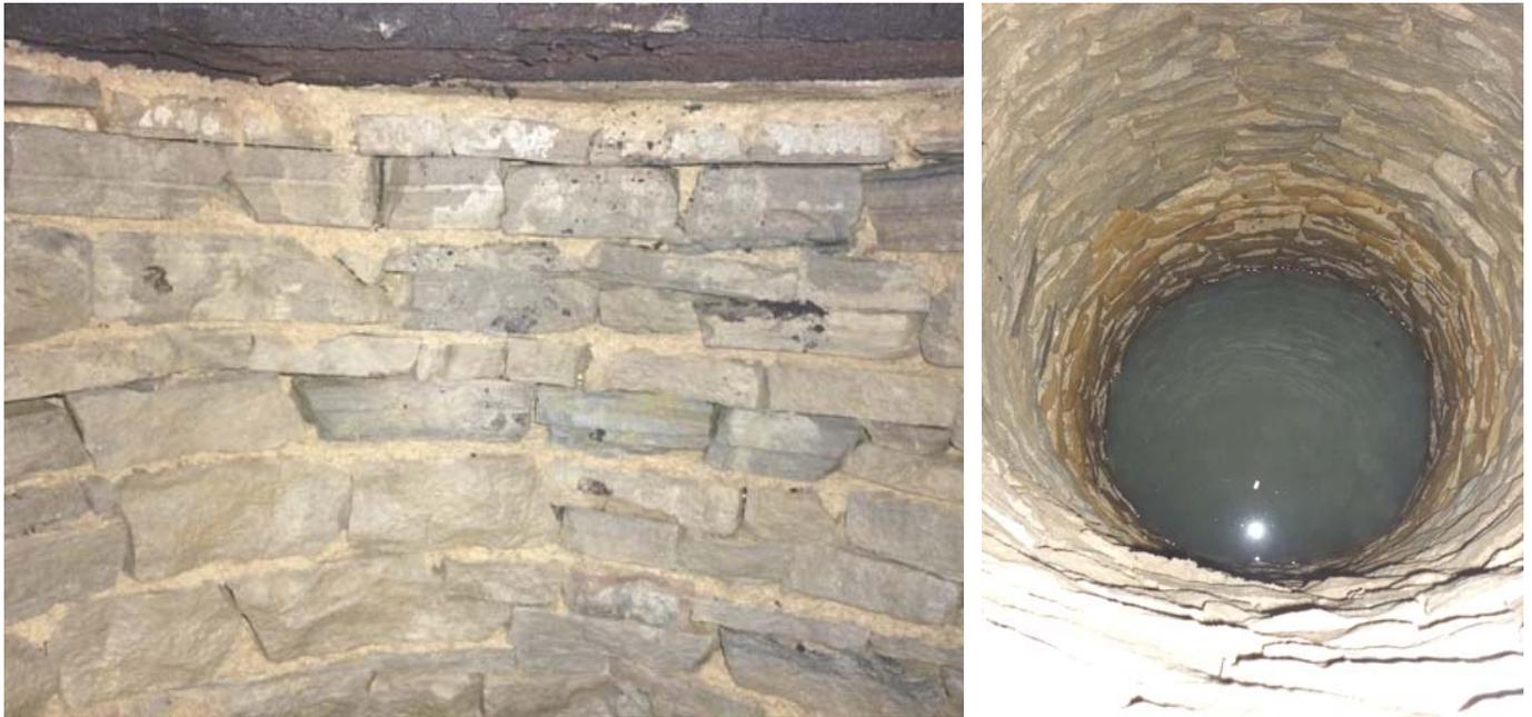
**Plate 20 (left): Internal construction detail of the well**
