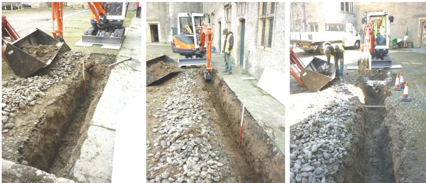
**Plate 12 (left): Trench section at the west end of the courtyard**
