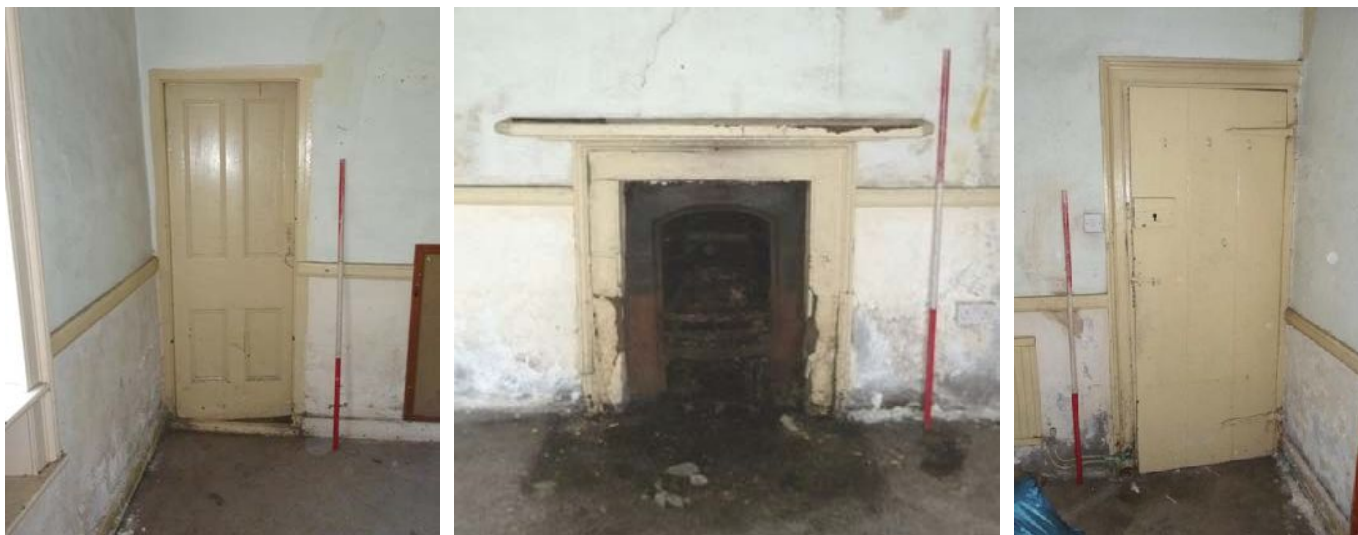
Plate 28 (left): Door in the east elevation of Ground Floor Room 2
