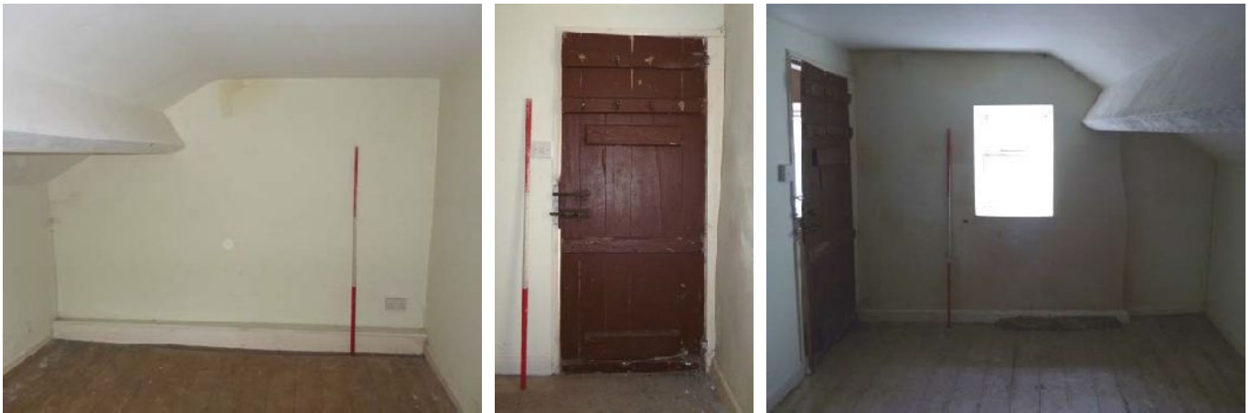
Plate 64 (left): East end of First Floor Room 1
