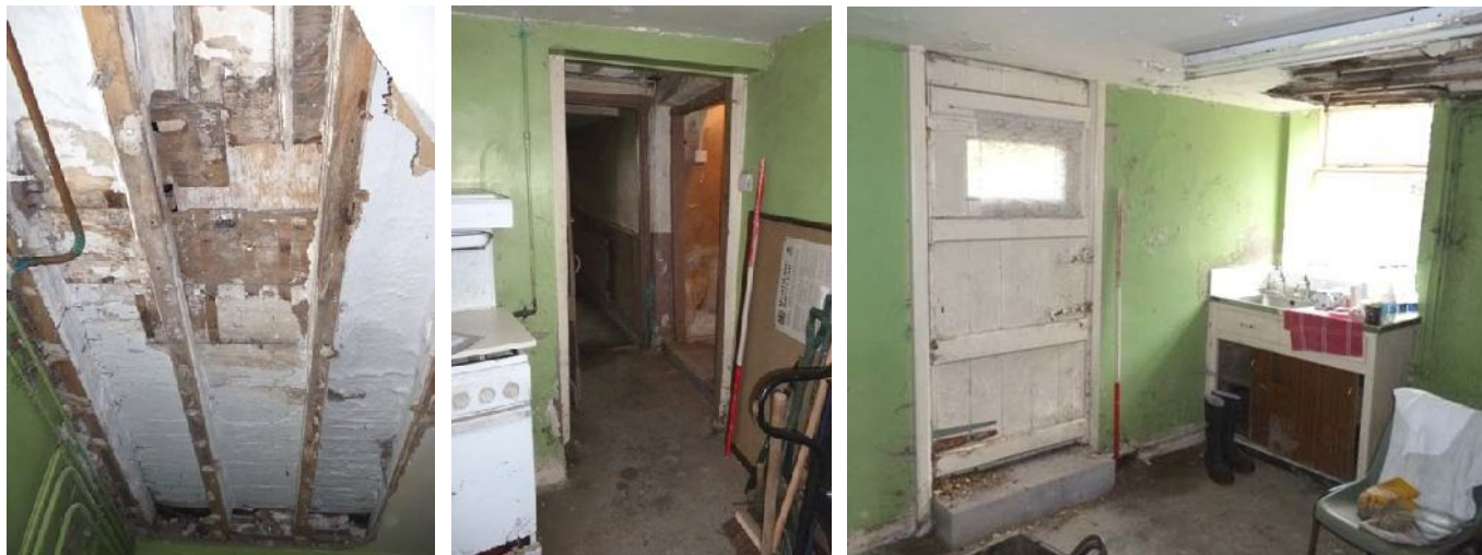
Plate 46 (left): Joists and floorboards for the room above visible from Ground Floor Room 5
