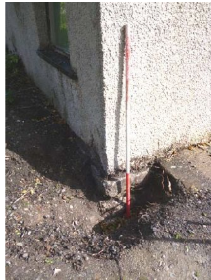
Plate 19 (right): Footings exposed at the south-east corner of the building
