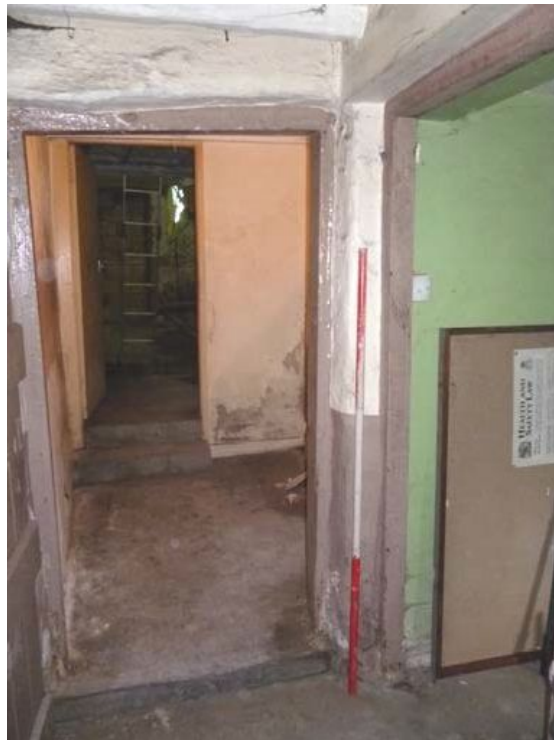
Plate 39: Centre and east end of Ground Floor Room 3
