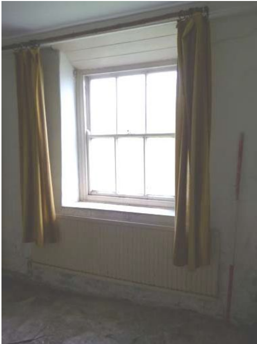
Plate 26 (left): Six-light sash window in Ground Floor Room 1
