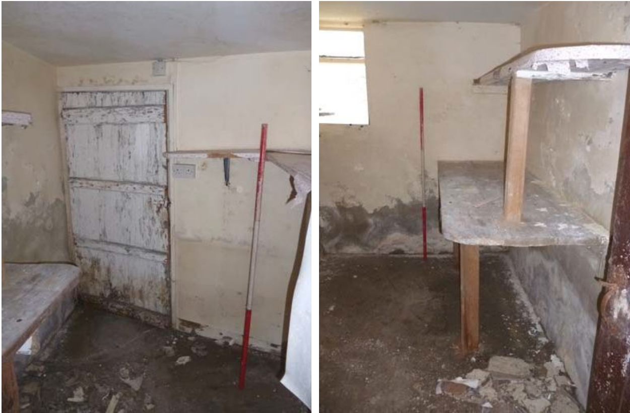
Plate 49 (left): The north elevation of Ground Floor Room 6, showing doorway
