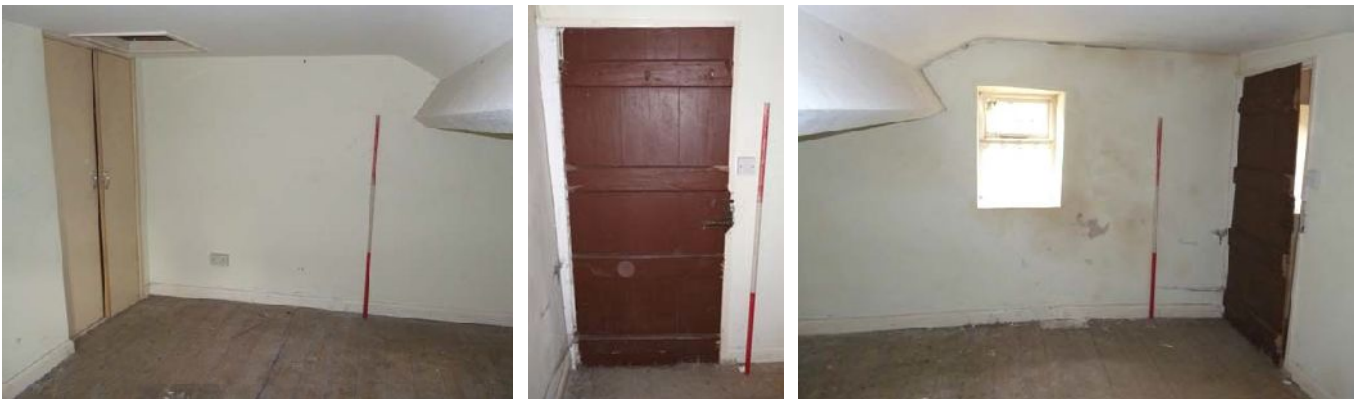
Plate 70 (left): North-east corner of First Floor Room 3
