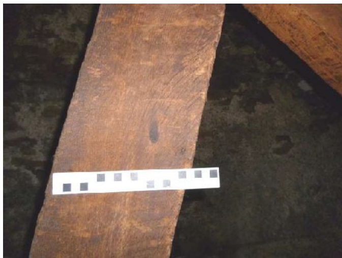
Plate 63 (left): Taper mark on north face of west of centre angled brace, south truss, Room A2
