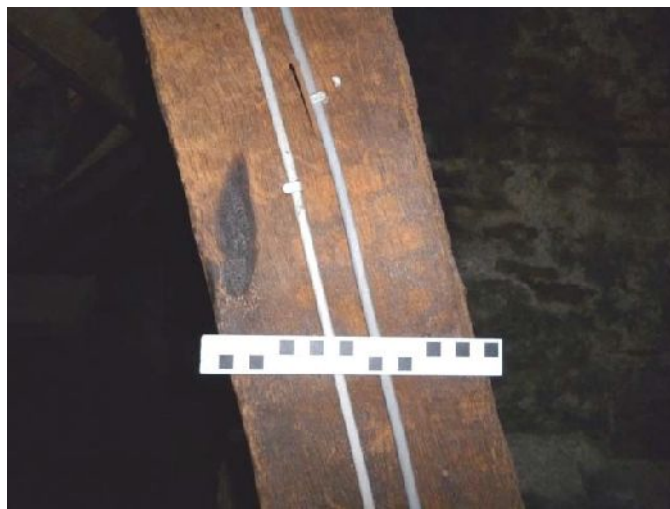
Plate 63 (left): Taper mark on north face of west of centre angled brace, south truss, Room A2
