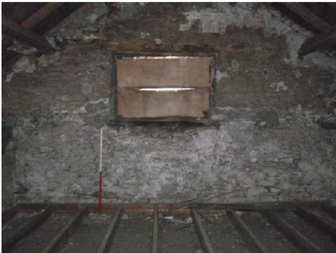
Plate 57 (left): Window in east elevation, Room A1
