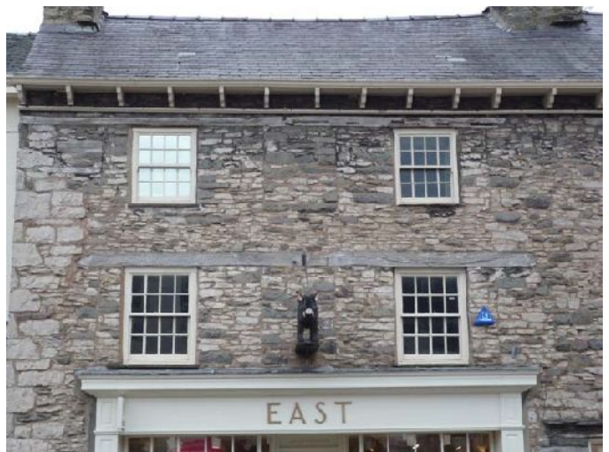
Plate 24 (left): South side of ground floor: window, formerly a doorway, and passage entrance
