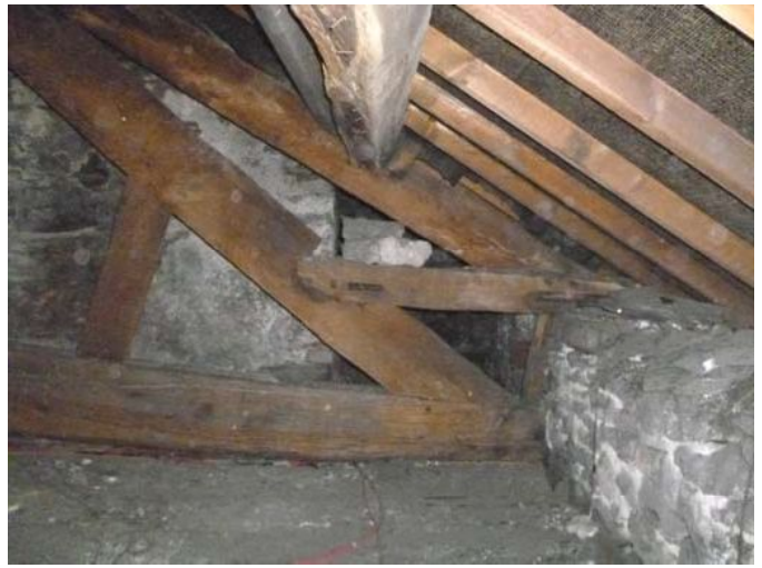
Plate 60 (right): Additional bracing timbers, west end of south truss, Room A2
