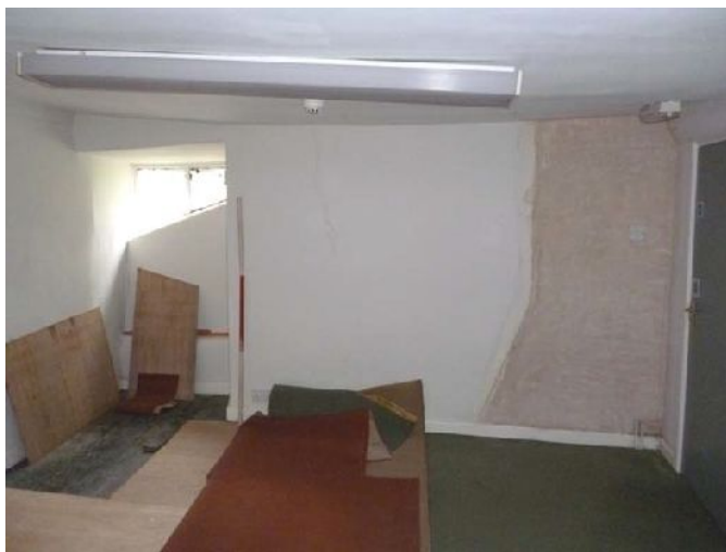
Plate 51 (right): Partially blocked window and blocked aperture, east elevation, Room S4
