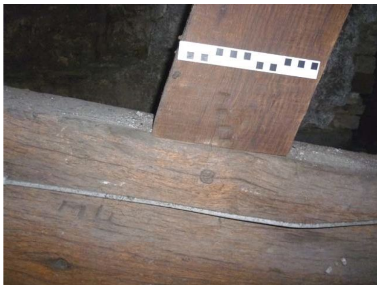
Plate 61 (left): Carpenter's marks 'II', west end, north face of south truss, Room A2
