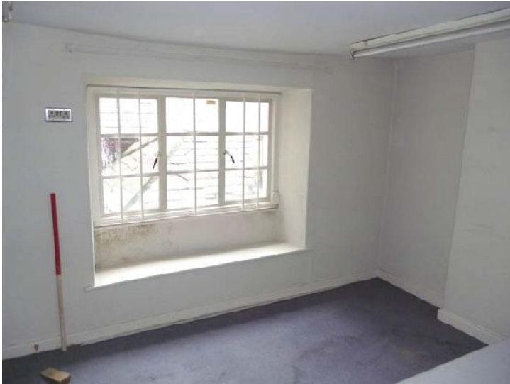
Plate 38 (left): Window, east elevation, Room F6
