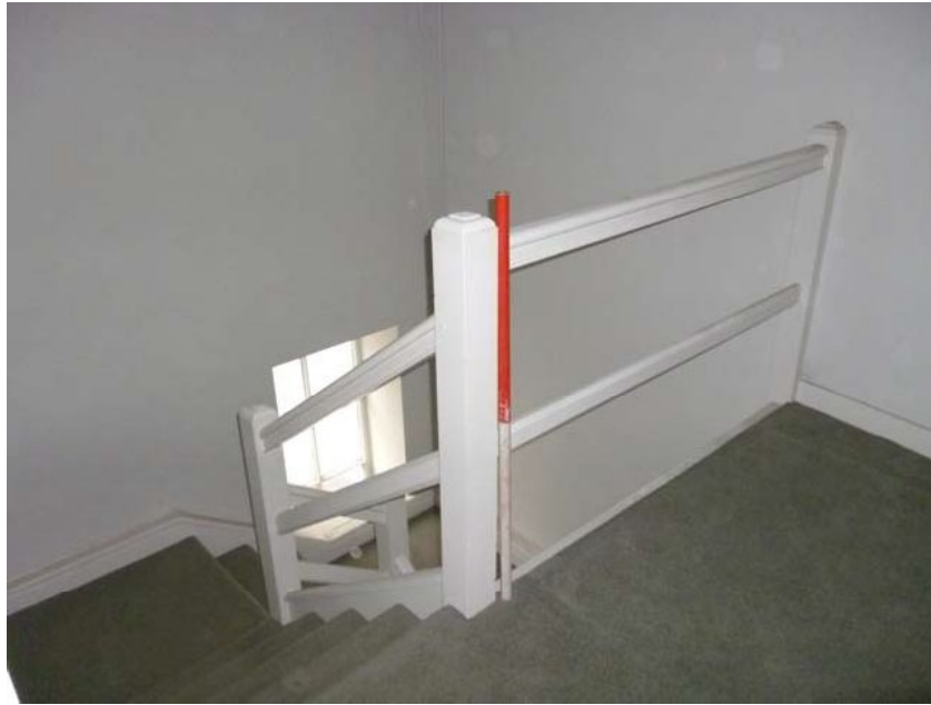
Plate 54: Staircase in Room S6
