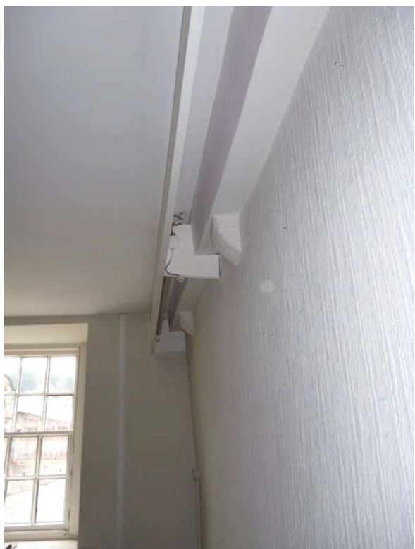
Plate 34 (left): Corbels supporting beam along north elevation, Room F4
