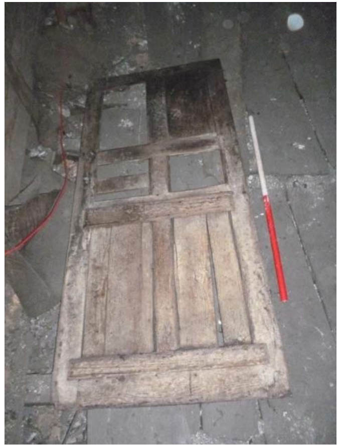
Plate 66 (right): Loose door presumed to be from doorway in north truss, Room A2
