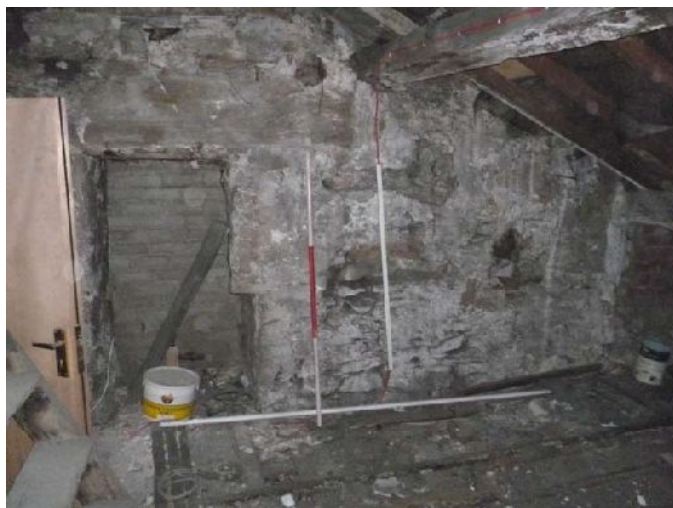
Plate 52 (left): West elevation, Room S5
