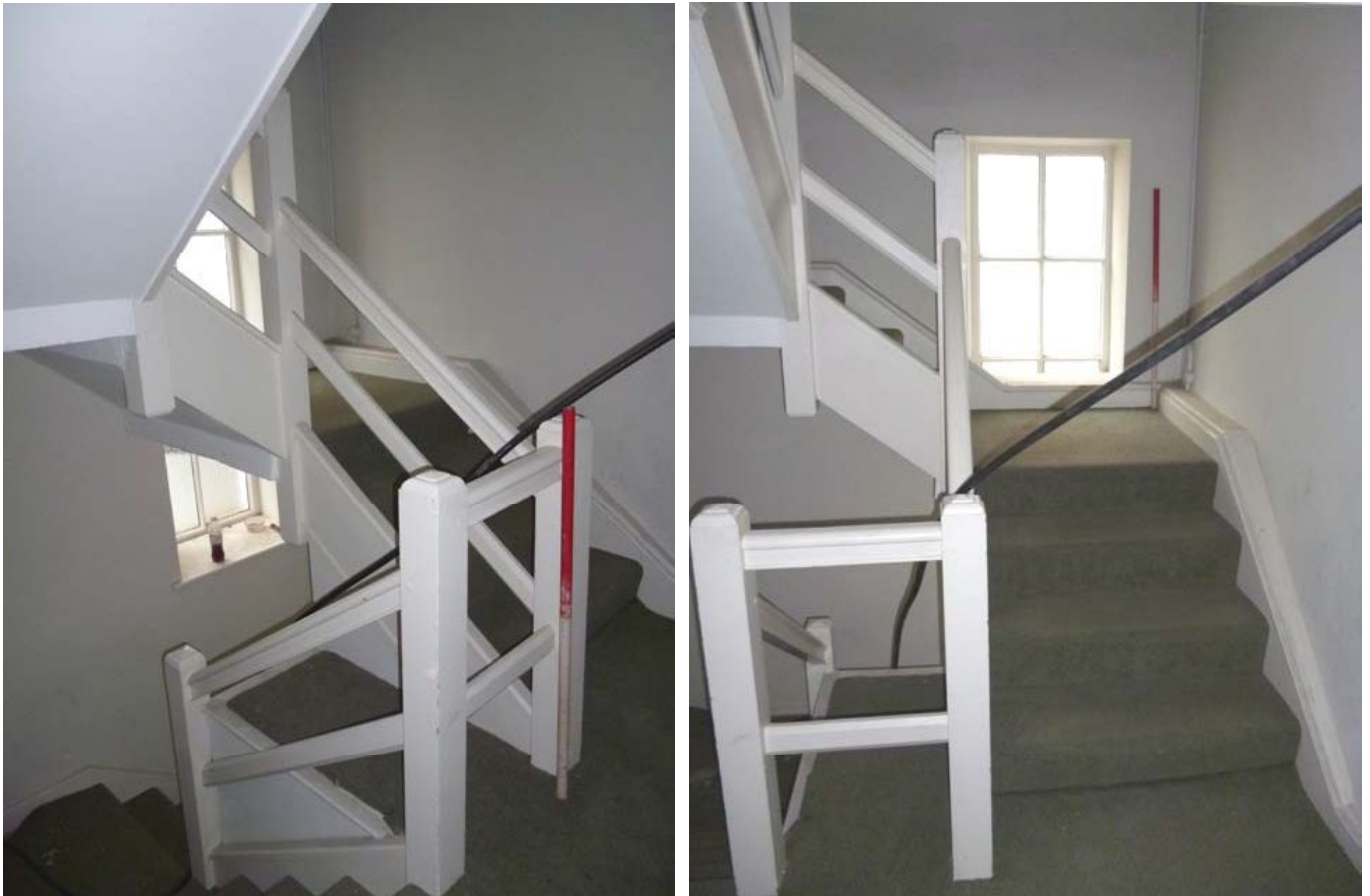
Plate 36 (left): Staircase in Room F5
