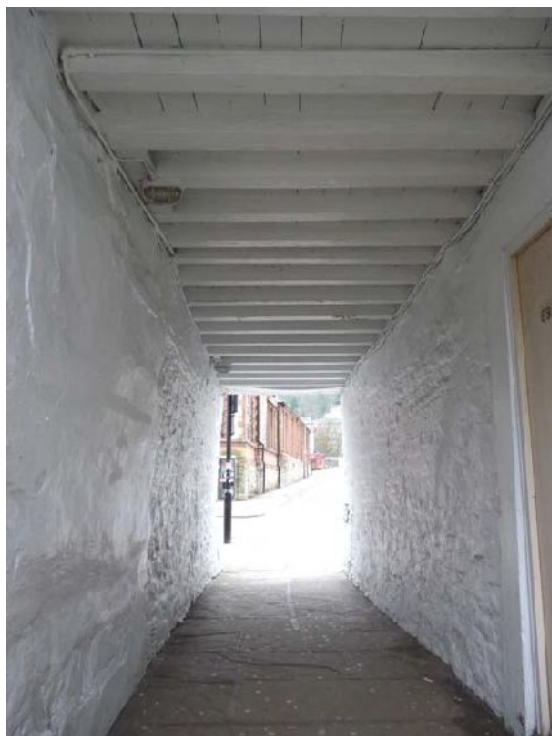
Plate 26 (left): General view of Room G1 showing the ceiling joists
