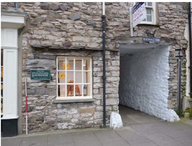
Plate 24 (left): South side of ground floor: window, formerly a doorway, and passage entrance
