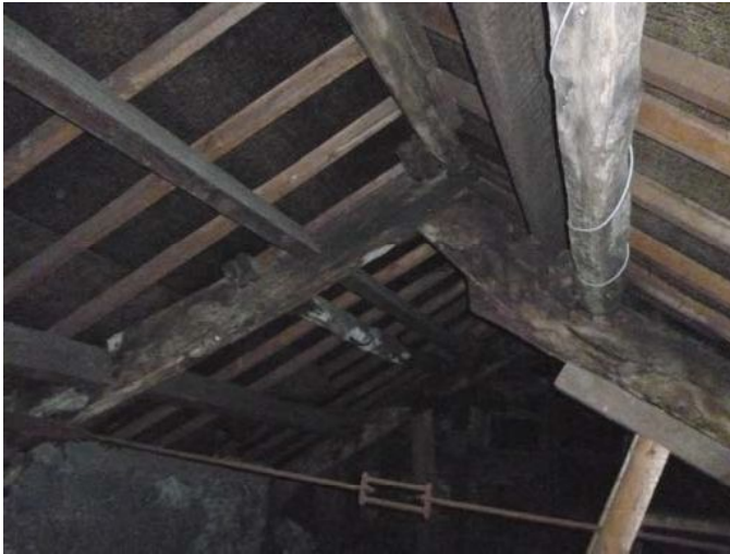
Plate 55 (left): East face of east truss, Room A1
