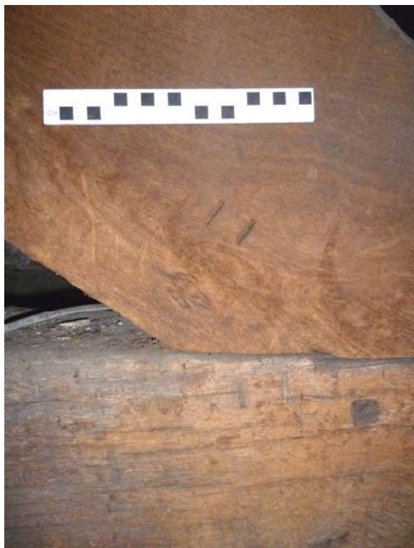
Plate 61 (left): Carpenter's marks 'II', west end, north face of south truss, Room A2
