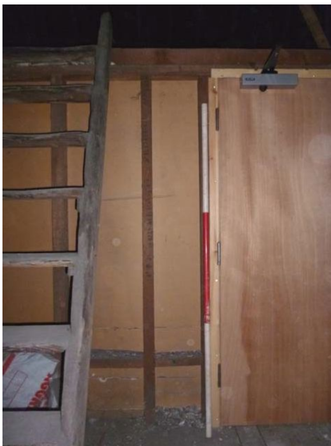
Plate 53 (right): Stud wall with re-used timber, south elevation, Room S5
