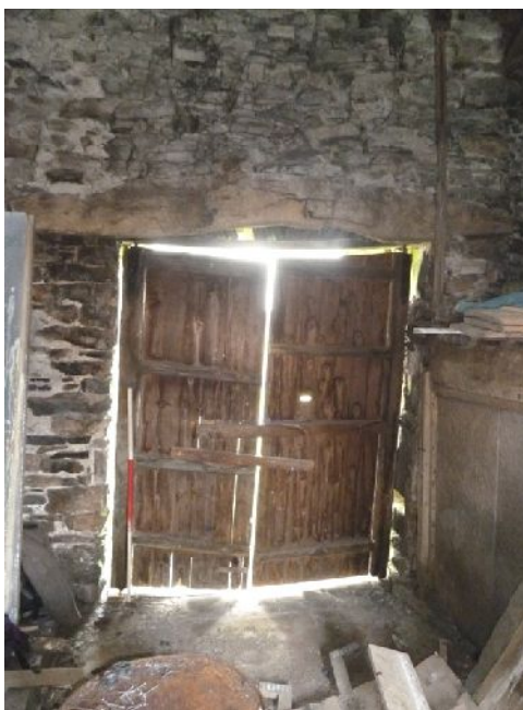
Plate 34: Doorway in the south elevation of Ground Floor Room 4
