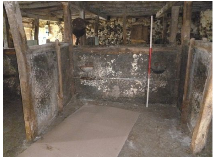
Plate 22 (left): Stall partitions in the Ground Floor Room 3
