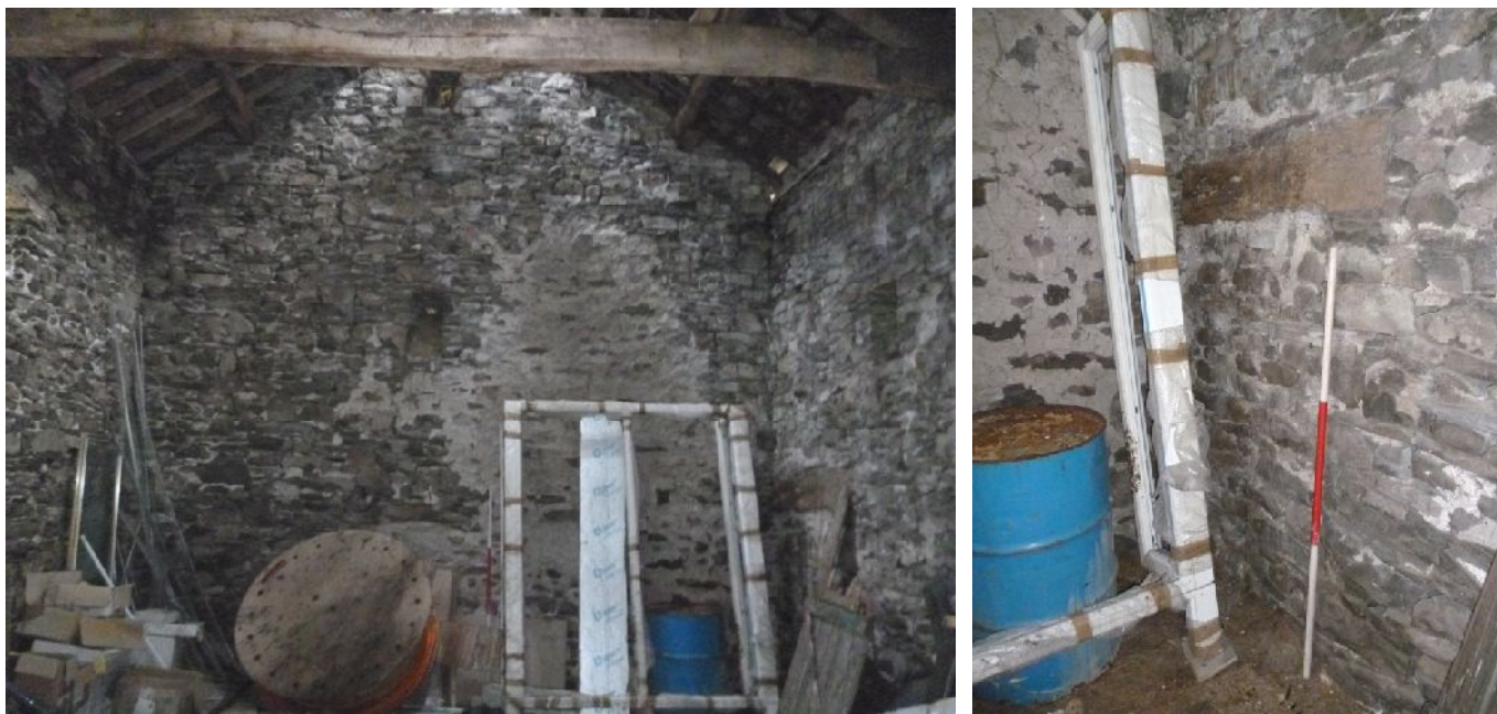
Plate 32 (left): The east elevation of Ground Floor Room 4
