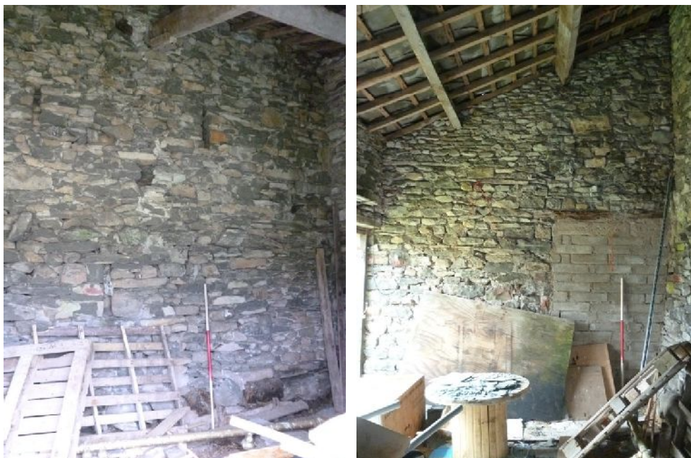
Plate 35 (left): North elevation of Ground Floor Room 5
