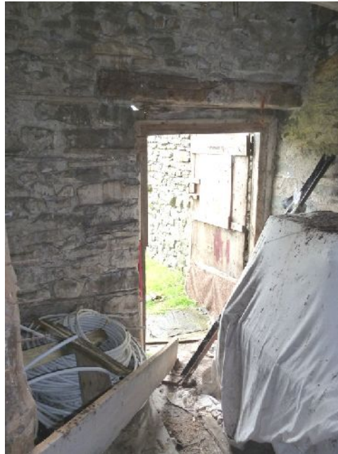
Plate 39: Doorway in the south elevation of Ground Floor Room 6
