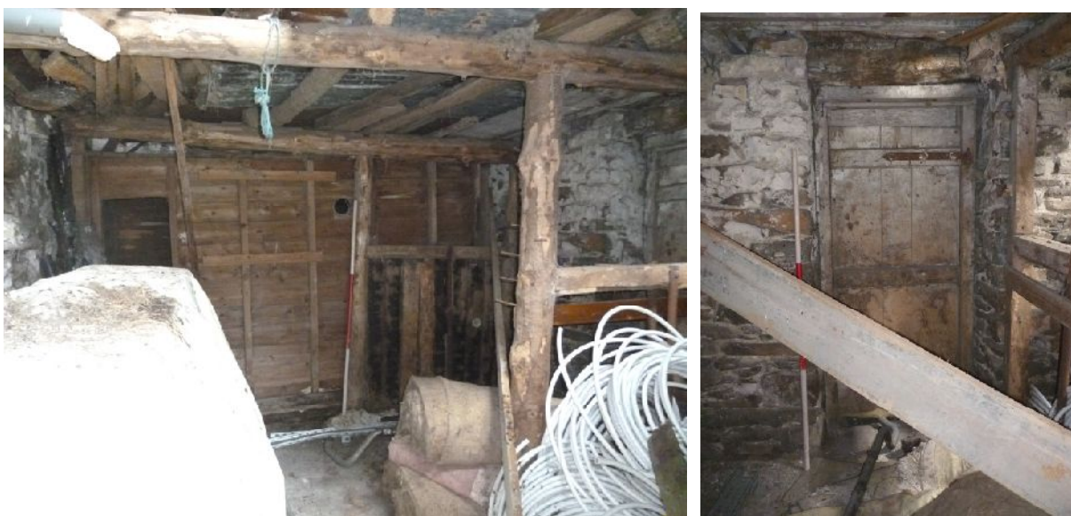
Plate 37 (left): North elevation of Ground Floor Room 6
