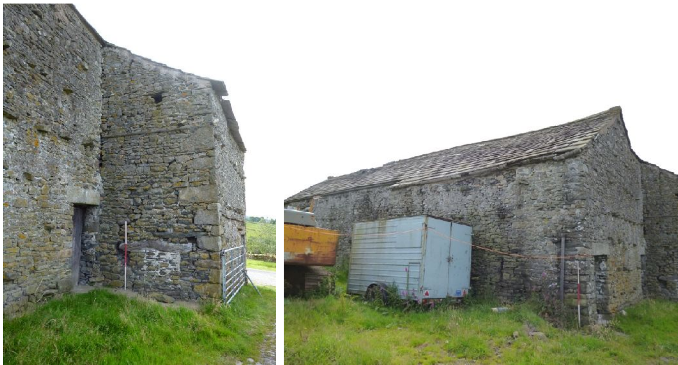
Plate 13 (left): Return in the centre of the west external elevation
