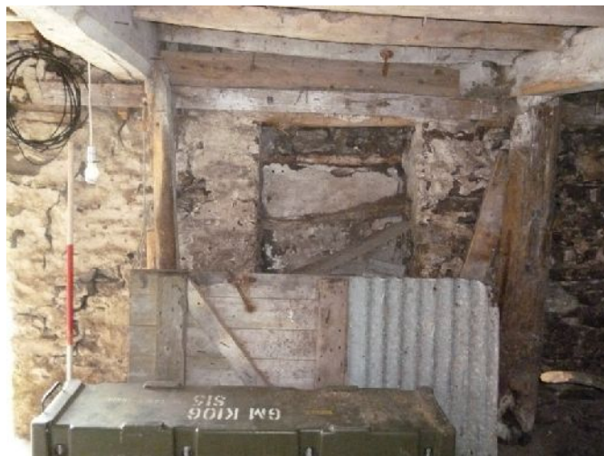
Plate 21: Alcove in the west elevation of Ground Floor Room 1
