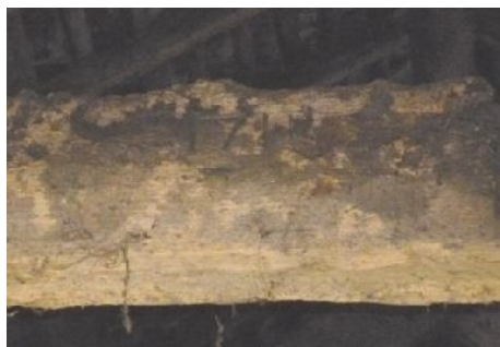
Plate 48: '1711' chiselled into the truss
