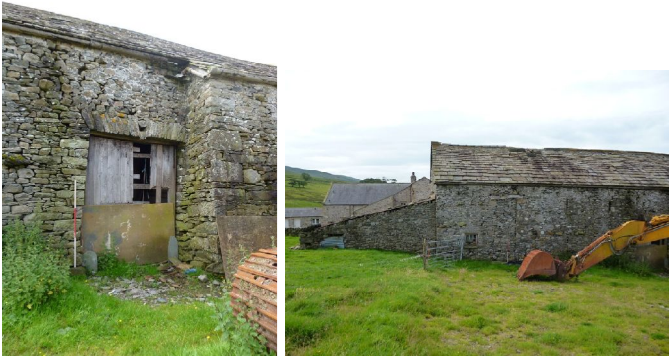
Plate 15 (left): Wagon doorway in the centre of the north external elevation
