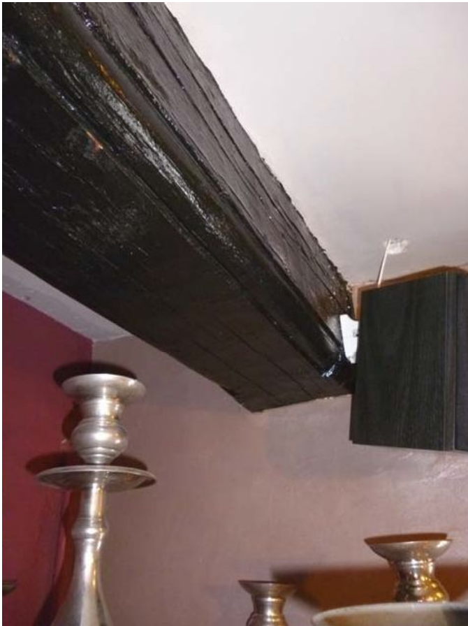
Plate 29 (left): Ovolo-moulded chamfer in Room G1
