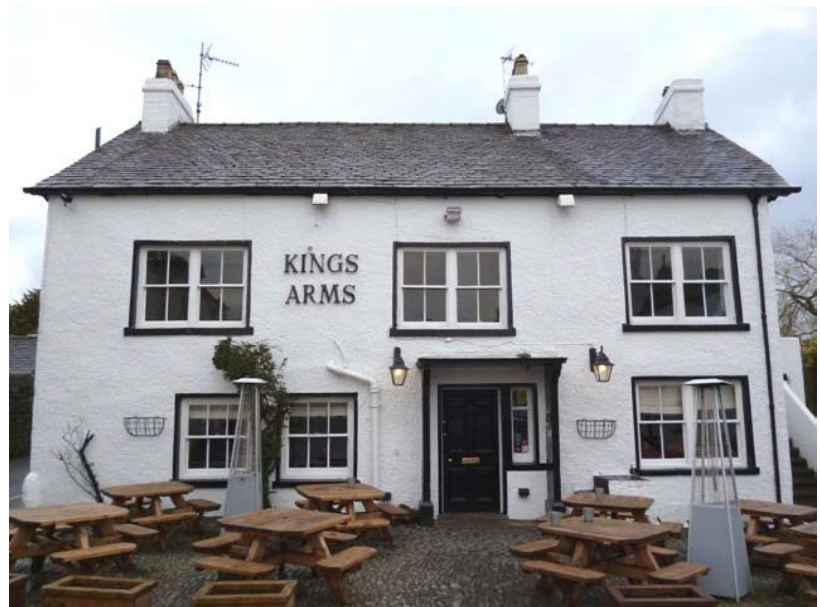
Plate 25 (left): North external elevation
