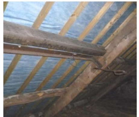
**Plate 72 (right): Iron brace between truss 'I' and 'II'**
