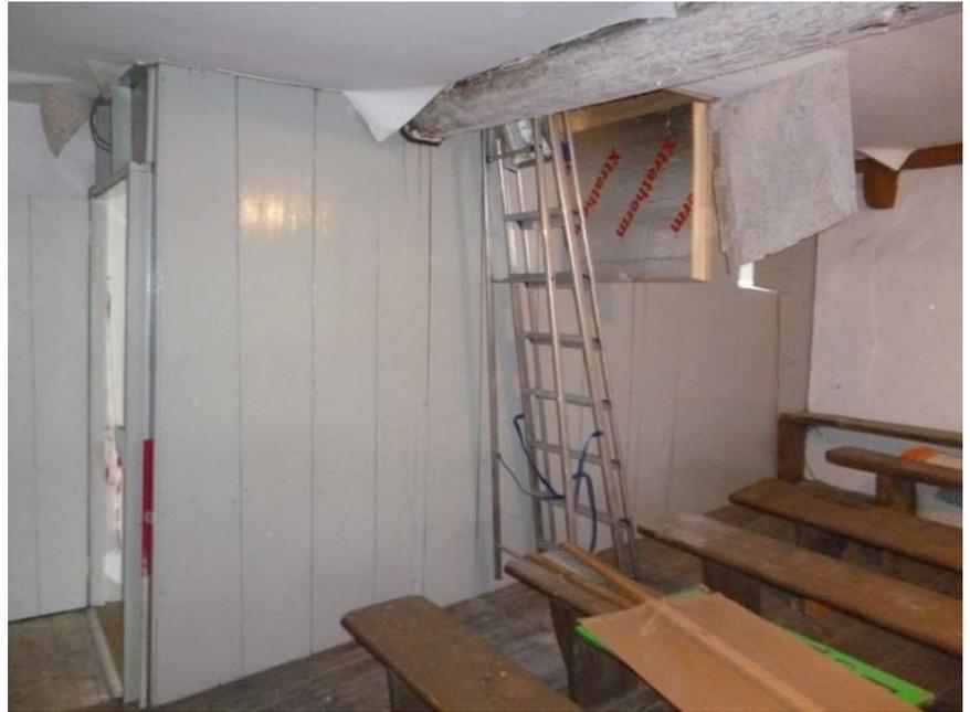
Plate 65 (right): Stud wall along the side of the stairs, viewed from First Floor Room 1
