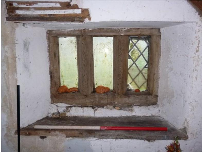
**Plate 42: Timber mullion window beneath the stairs**
