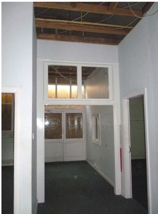
Plate 101 (left): Tops of windows obscured by a suspended ceiling, south-east elevation, Room 19
