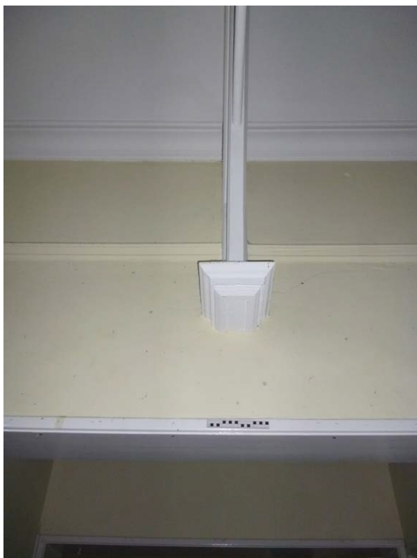
Plate 89 (left): Damaged corbel, north-west end of truss, Room 16
