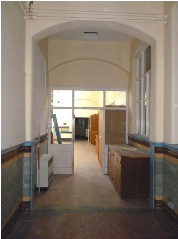
Plate 105 (left): North-east end of Room 21, showing the divided opening and higher arch over the doorway into Room 12
