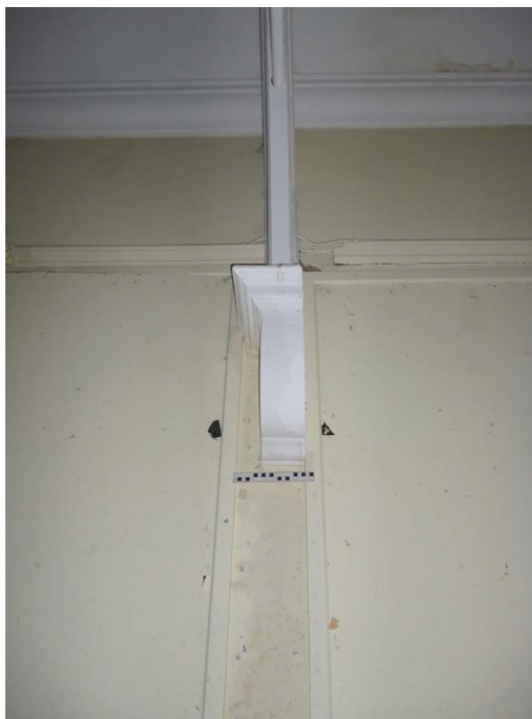
Plate 89 (left): Damaged corbel, north-west end of truss, Room 16
