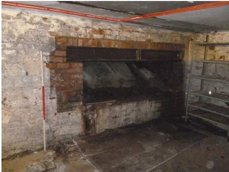
Plate 115: Coal chute in the north-east elevation of the north-east room of the basement
