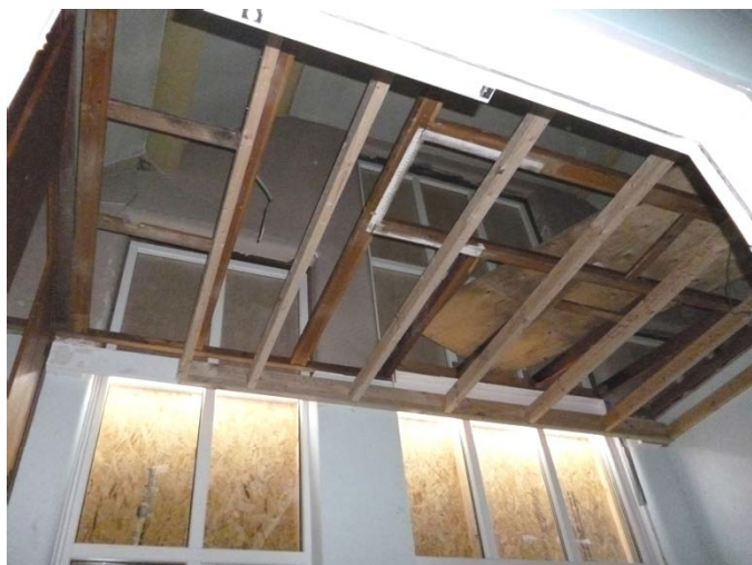
Plate 101 (left): Tops of windows obscured by a suspended ceiling, south-east elevation, Room 19
