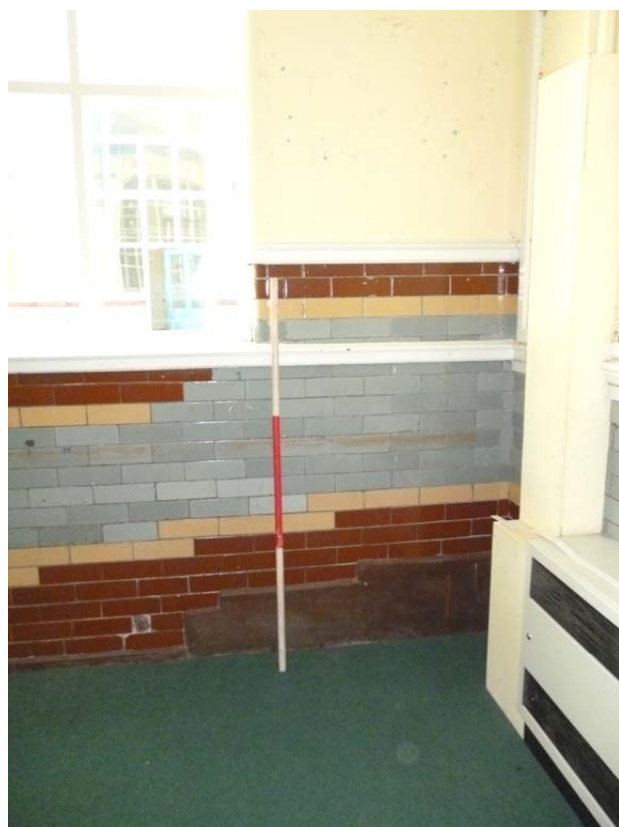
Plate 83 (left): Stepped bricks and concrete, south-east side, north-east elevation, Room 14
