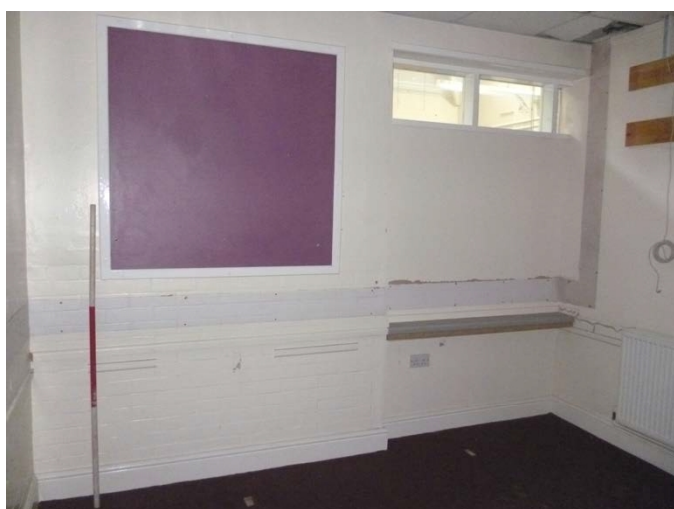
Plate 57 (left): High-level windows in north-east elevation within blocked doorway
