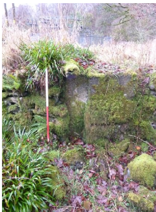
Plate 17 (left): Concrete rebate for a sluice gate on the east side of the north arm of the mill race ( Element 04 )
