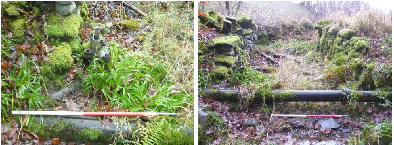
Plate 19 (left): Valve ( Element 05 ) and associated pipe ( Element 06 )
