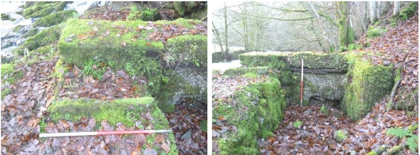
Plate 13 (left): Detail of the north side of the sluice ( Element 03 )
