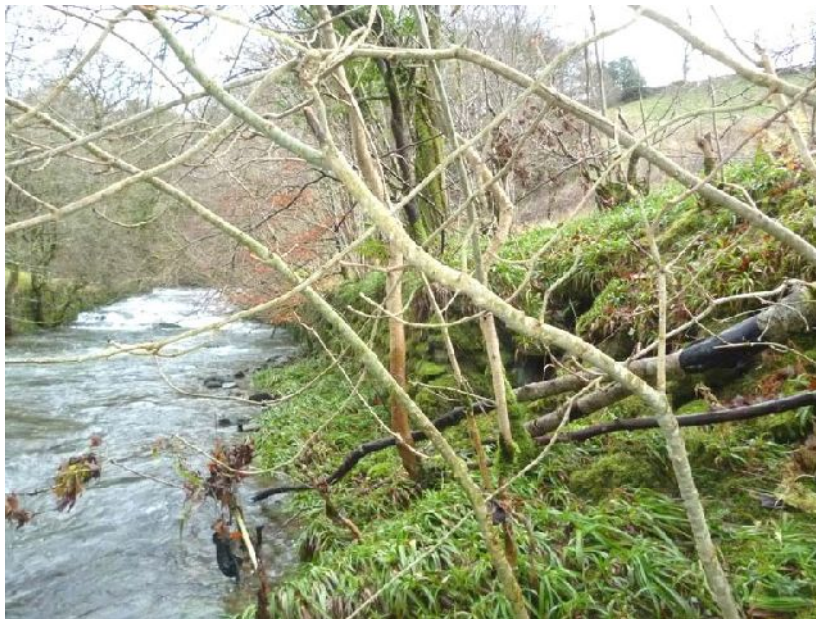
Plate 21: Retaining wall ( Element 07 ) alongside the Trout Beck
