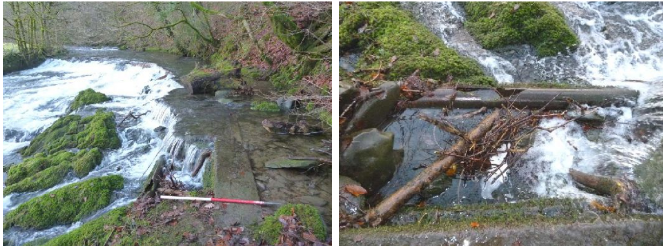
Plate 10 (left): General view of the weir ( Element 01 )
