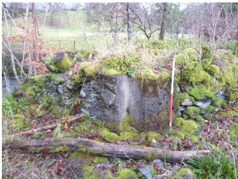
Plate 17 (left): Concrete rebate for a sluice gate on the east side of the north arm of the mill race ( Element 04 )
