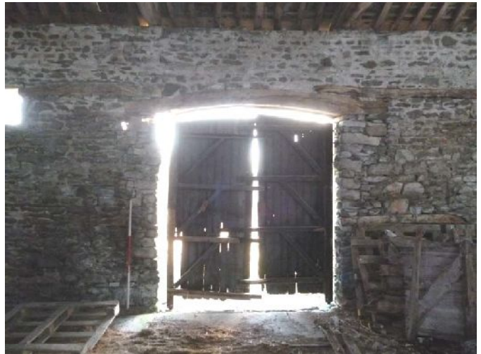
Plate 48 (left): North-eastern pitching or winnowing doorway, south-east elevation, Room F1
