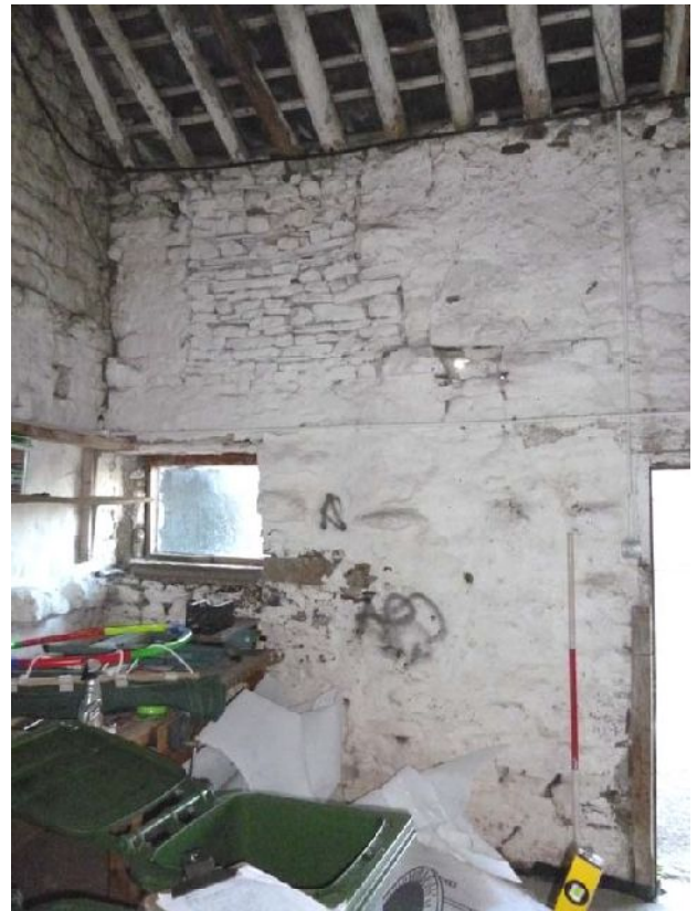
Plate 26 (left): South elevation, Room G3, showing the junction between the outshut and the main barn
