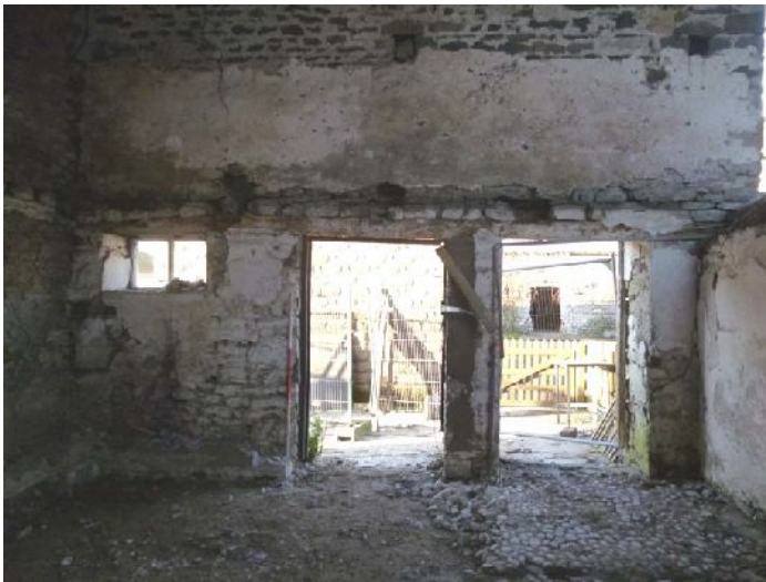
Plate 40 (left): Doorways and window sharing a single piece of re-used timber as a lintel, north-west elevation, Room G7
