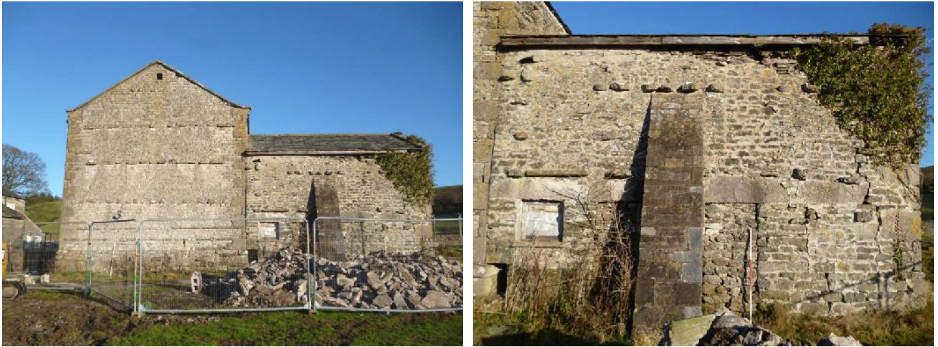
Plate 12 (left): The central and south-east part of the south-west elevation
