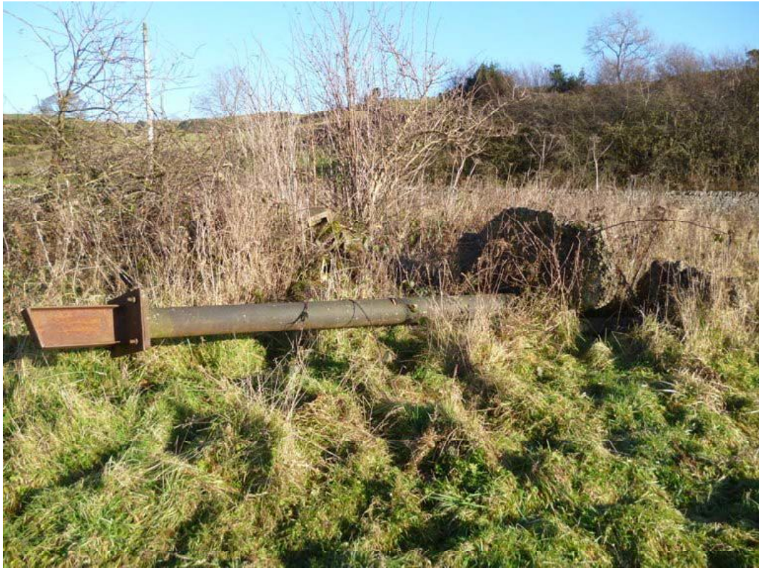
Plate 21: Iron columns lying loose to the south-east of the barn
