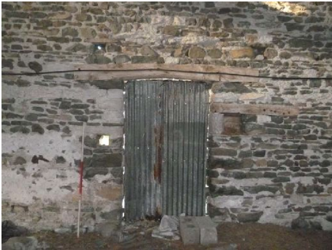
Plate 48 (left): North-eastern pitching or winnowing doorway, south-east elevation, Room F1
