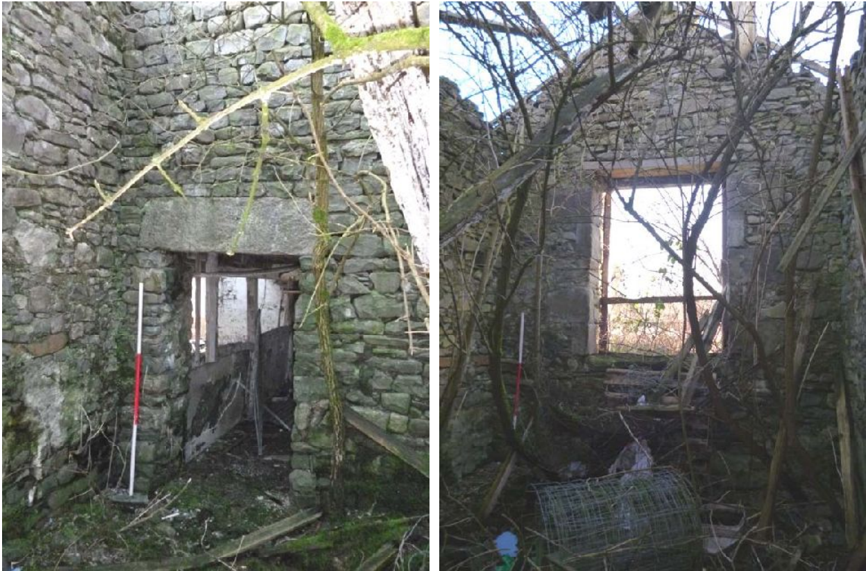
Plate 44 (left): Doorway in the north-west elevation, Room G9
