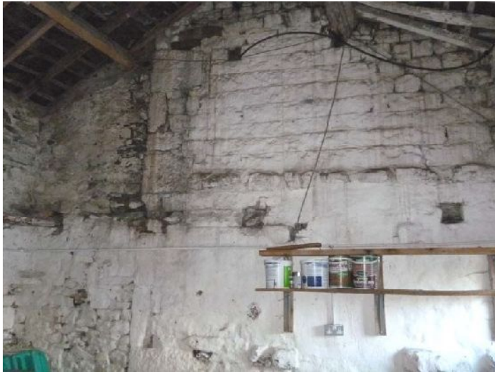
Plate 26 (left): South elevation, Room G3, showing the junction between the outshut and the main barn
