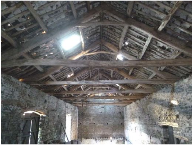
Plate 46 (left): Trusses in Room F1
