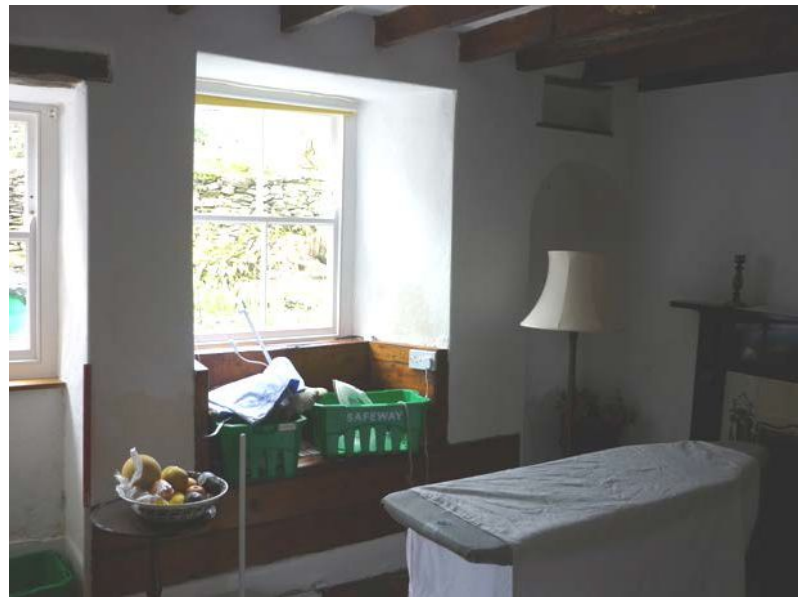
Plate 23 (left): Window, original a doorway, on the north side of the east elevation of Room 4
