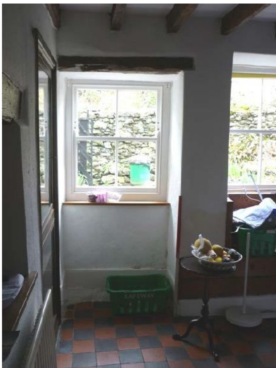
Plate 23 (left): Window, original a doorway, on the north side of the east elevation of Room 4
