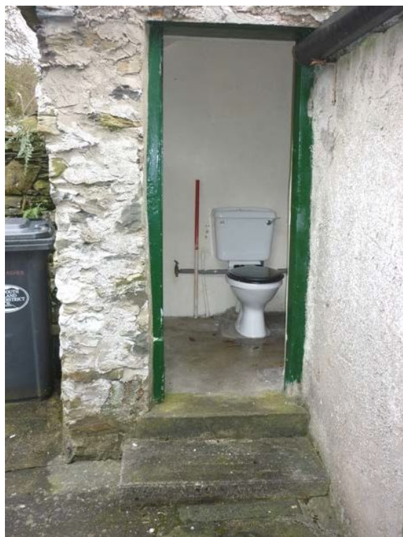
Plate 27 (left): East elevation of Room 8, showing roughcast render
