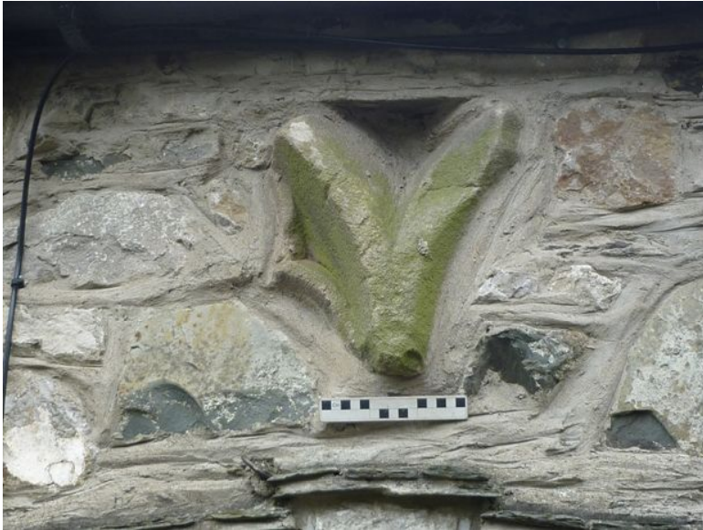
Plate 10 (left): Re-used medieval masonry above the southern window at the north end of the east external elevation, probably a piece of window tracery
