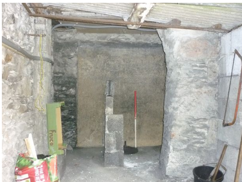
Plate 27 (left): East elevation of Room 8, showing roughcast render
