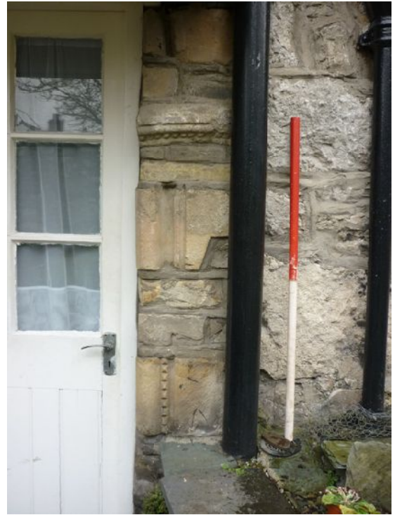
Plate 10 (left): Re-used medieval masonry above the southern window at the north end of the east external elevation, probably a piece of window tracery
