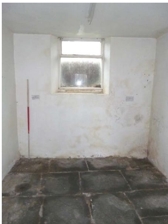
Plate 135 (left): North-west end of Room G2, showing flag floor
