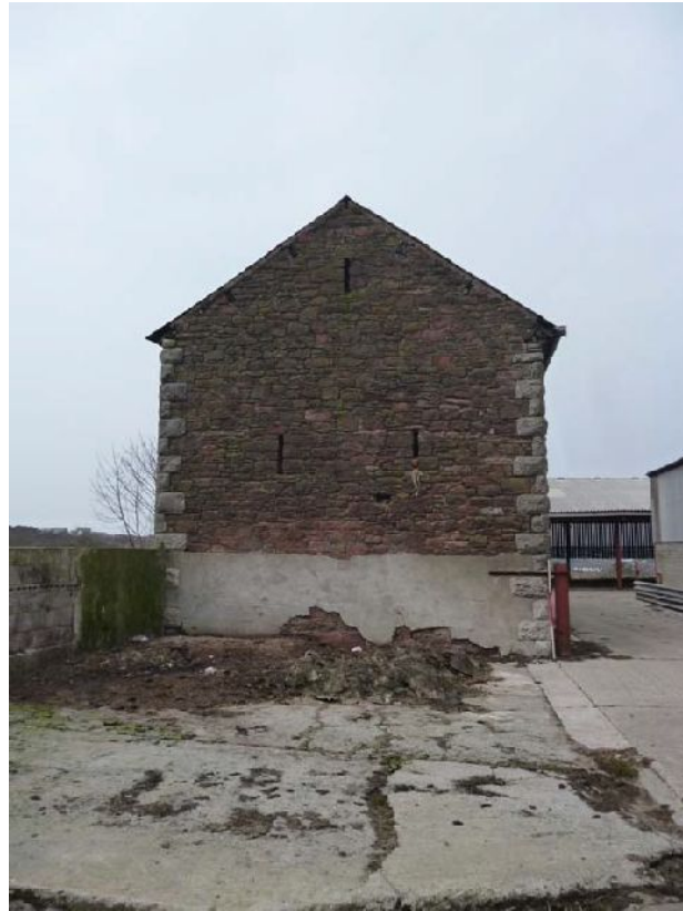
Plate 14: South-east external elevation, Building 1
