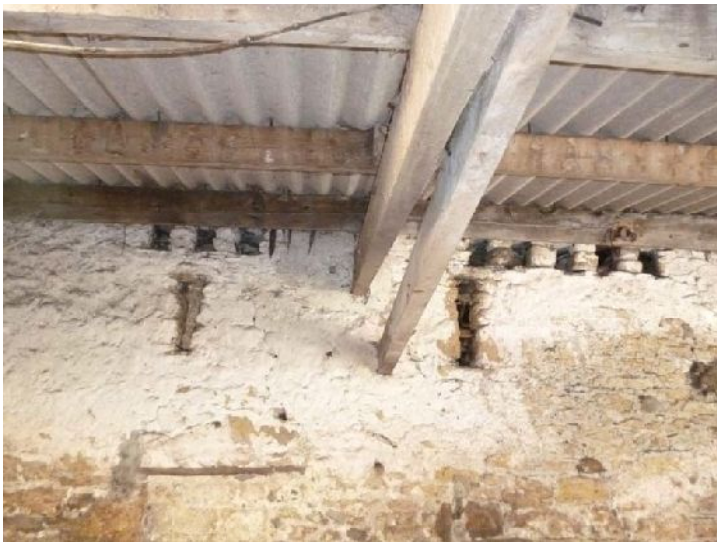
Plate 80 (left): Ventilation slots and holes forming a probable dove cote, south-east elevation, Room 5, Building 3
