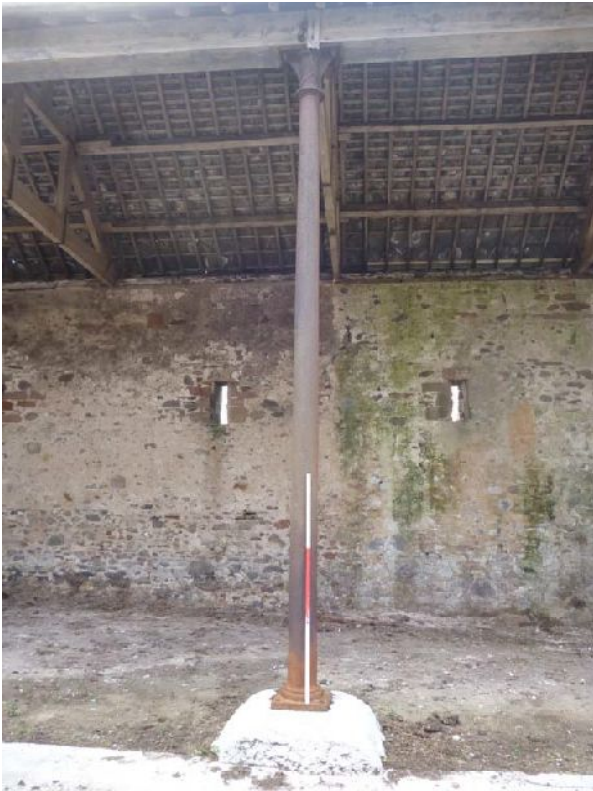
Plate 10 (left): Detail of iron column supporting roof, north-east external elevation, Building 1
