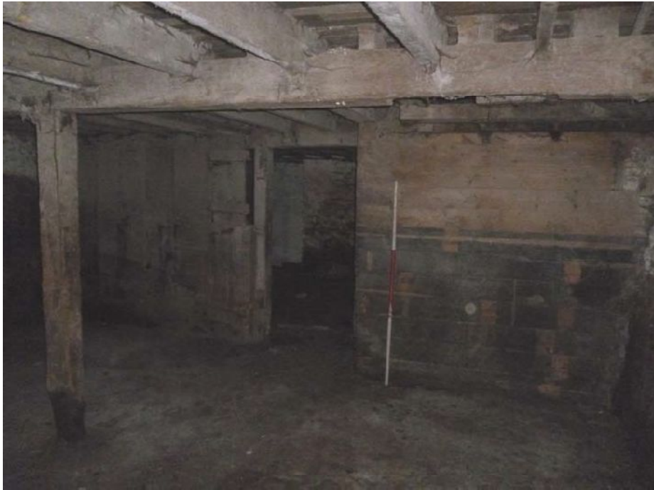
Plate 71: Timber walls below the inserted floor, Room 4, Building 3
