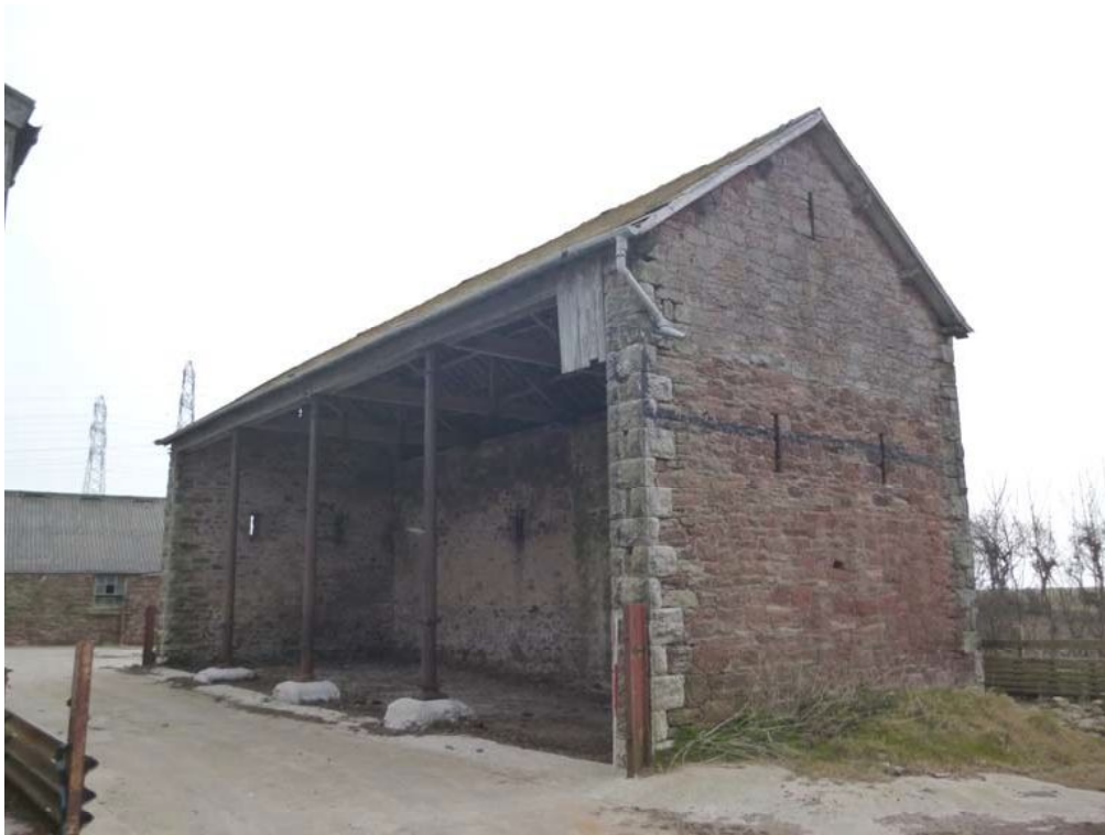
Plate 9: The north-east and north-west external elevations, Building 1
