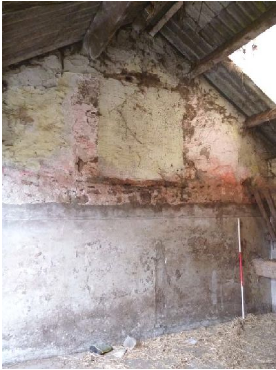
Plate 99 (left): Blocked window in north-west elevation, Room 1, Building 4
