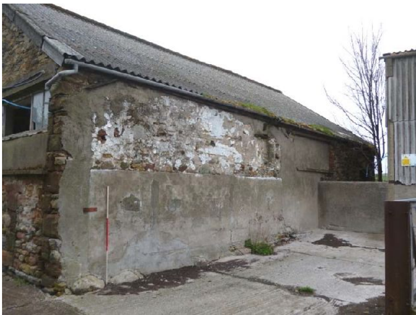
Plate 46: North-east end of the south-east external elevation, Building 6
