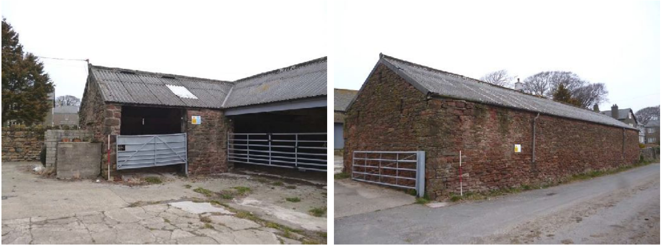
Plate 30 (left): North-west side of the south-west external elevation, Building 4
