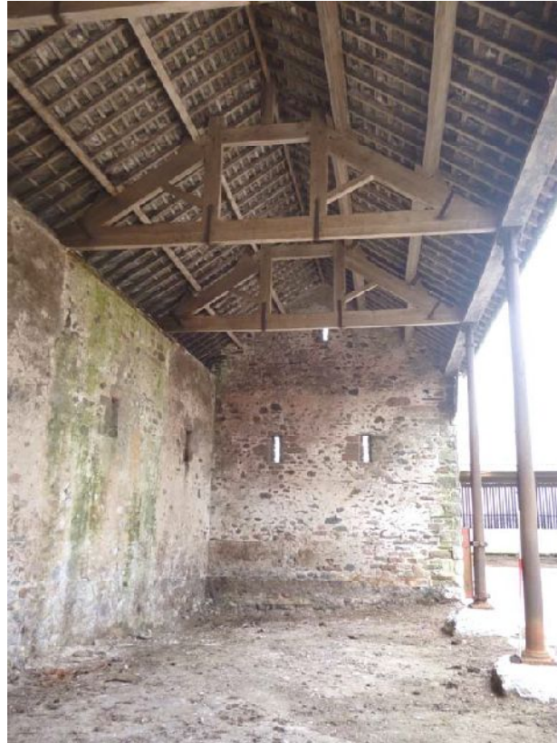
Plate 53: Trusses in Building 1
