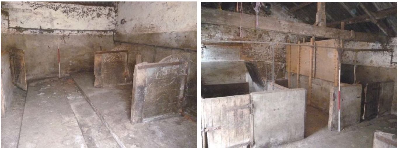
Plate 103 (left): Dung channel and south-west stall, Room 3, Building 4
