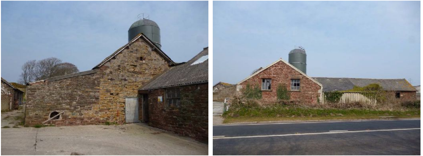
Plate 24 (left): North-west side of the south-west external elevation, Building 3
