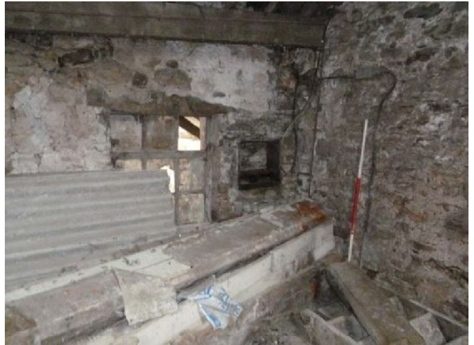
Plate 74 (left): Truss incorporated in the north-east elevation, Room 4, Building 3
