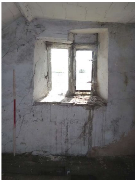
Plate 164 (left): Mullion window in south-east end of Room A2
