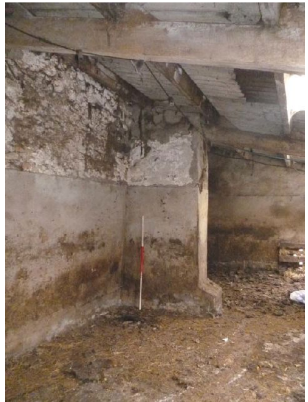
Plate 80 (left): Ventilation slots and holes forming a probable dove cote, south-east elevation, Room 5, Building 3
