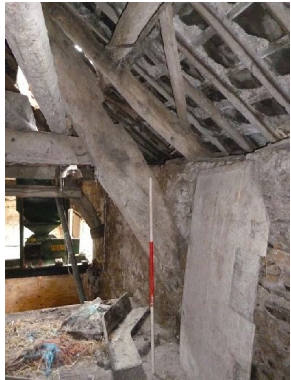
Plate 72 (left): Detail of truss end showing packing piece and wind brace, Room 4, Building 3
