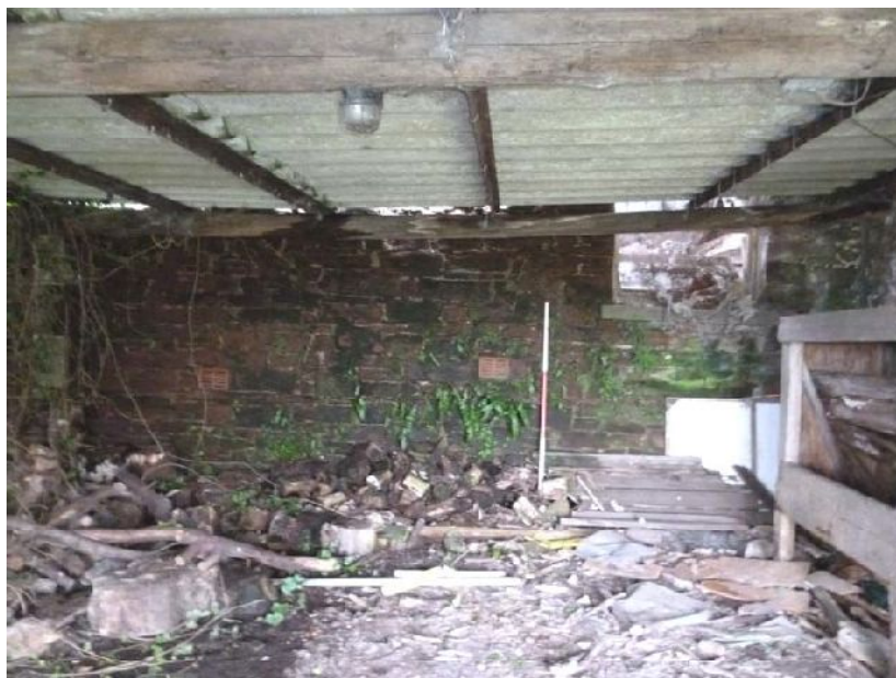
Plate 98: North-west elevation, Room 9, Building 3
