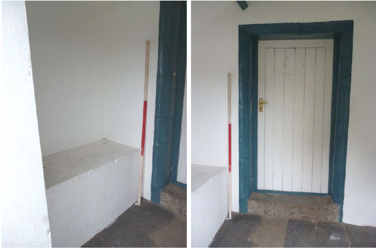
Plate 149 (left): Stone bench, north-west side of Room G8
