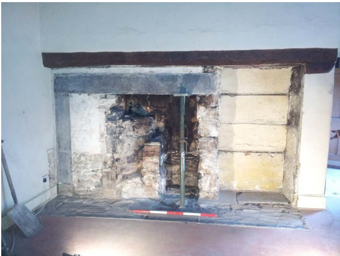
Plate 5: Remodelled fireplace set within blocking (photograph by Dale Rennard)
