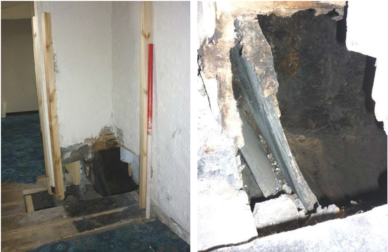
Plate 8 (left): Exposed smoke hood in Room F3
