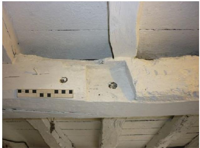
Plate 36 (right): Re-used cruck in Ground floor Room 4
