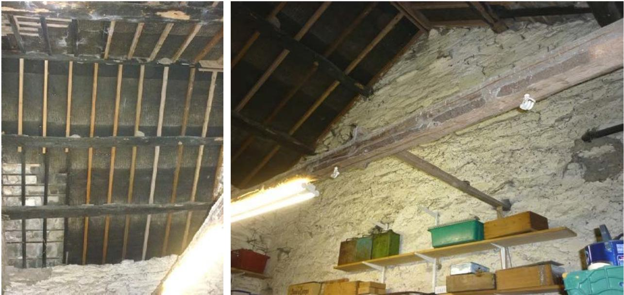
**Plate 28 (left): Fire damage in the roof above Ground floor Room 3**
