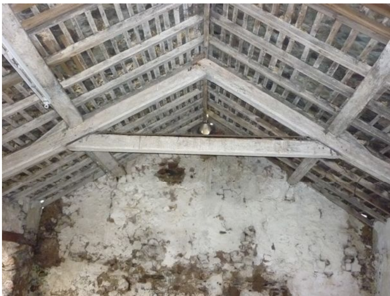
Plate 9: Truss in Room 1, north-west face
