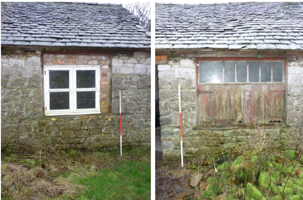
Plate 6 (left): North-west window, north-east external elevation
