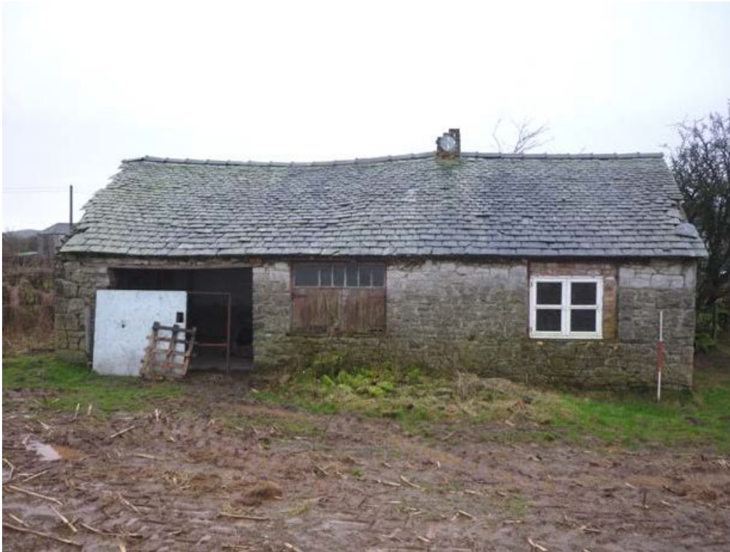
Plate 5: North-east external elevation
