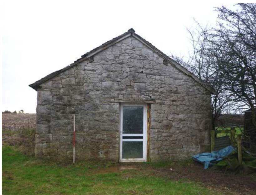
Plate 4: North-west external elevation
