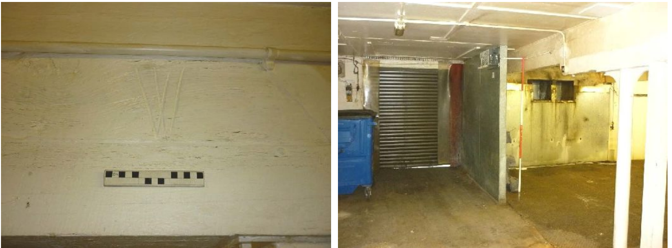
Plate 36 (left): Baltic timber mark in the beam south of the north wall in Room G5
