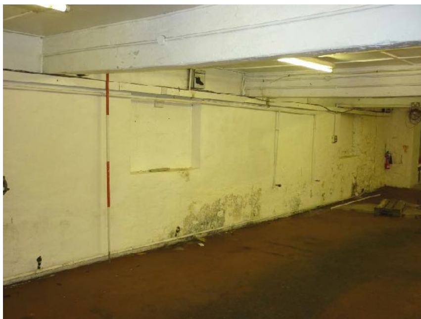
Plate 33: Blocked windows in the west elevation of Room G4
