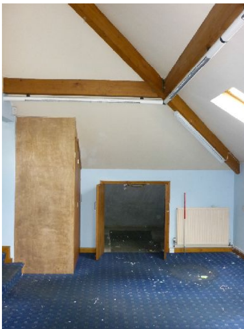
Plate 49: West elevation of Room F1
