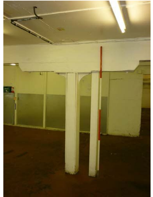
Plate 28 (right): Boxed column and square section girder beneath the beams in Room G4
