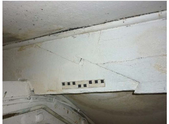
Plate 65 (left): Baltic marks on truss in Attic Room 2
