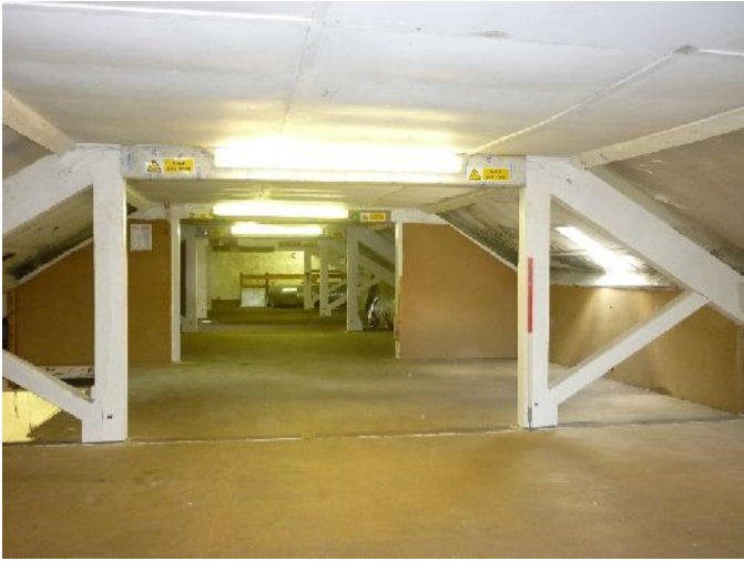
Plate 63 (left): Lower part of the trusses in Attic Room 2
