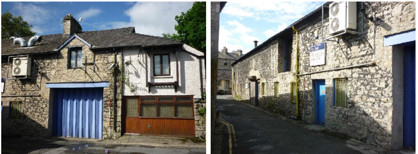
Plate 12 (left): The north end of the east external elevation
