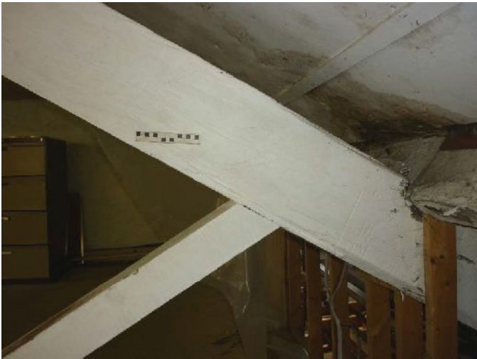
Plate 65 (left): Baltic marks on truss in Attic Room 2
