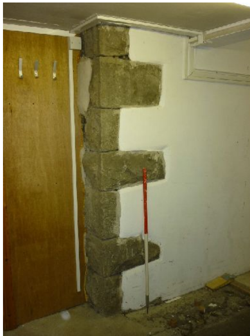
Plate 21: Original external wall of the 'cottage' visible in Room G1
