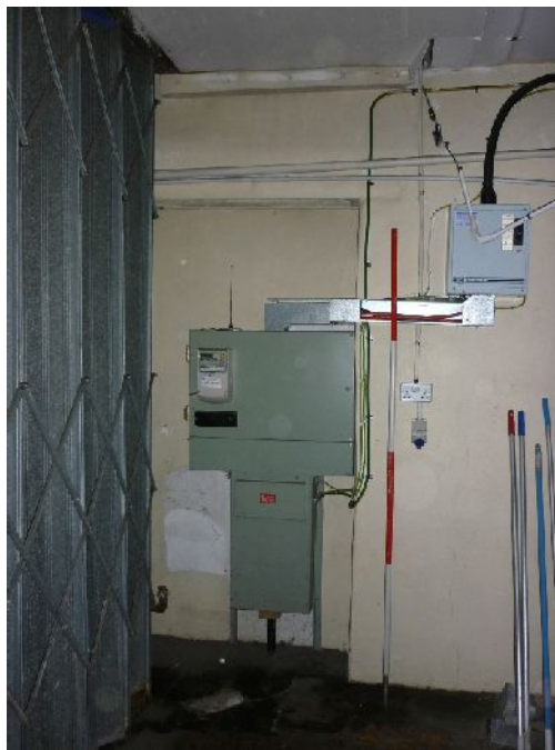
Plate 24: South elevation of Room G2
