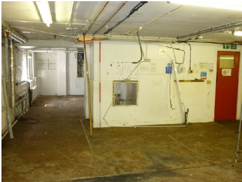
Plate 58: South end of the west elevation of Room F5
