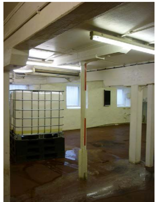
Plate 28 (right): Boxed column and square section girder beneath the beams in Room G4
