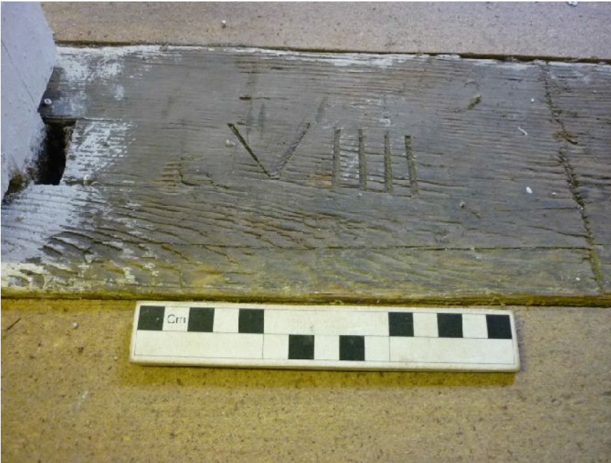
Plate 67 (left): Carpenter's marks in Attic Room 2
