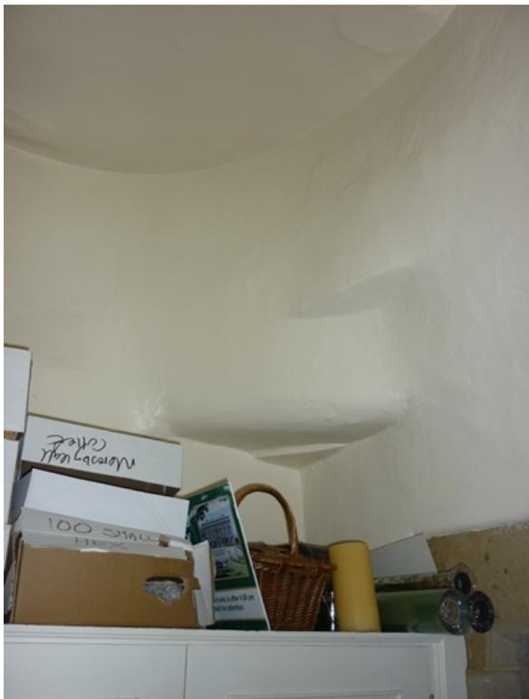
**Plate 75 (left): Corbelled remnants of spiral stair in east wing behind south section**
