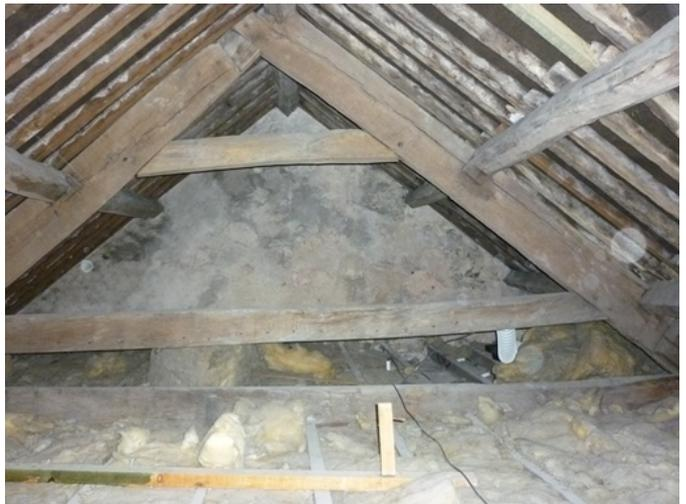
**Plate 80 (right): Roof truss with collar on the west side of the south section of the hall**
