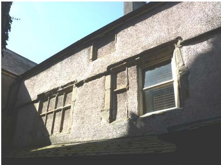
**Plate 81 (left): Mullion and transom windows with hood moulds on the north side of the courtyard**
