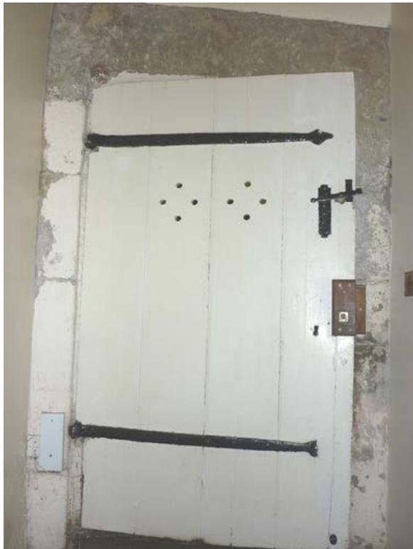
**Plate 74 (right): Early plank door with long strap hinges leading east**
