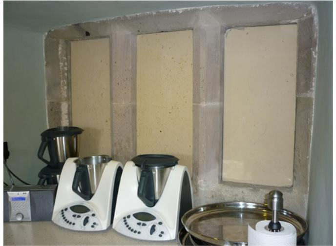
**Plate 70 (right): Blocked mullion window in the west wing behind the south section**
