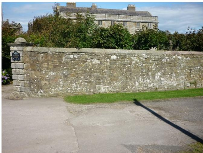
**Plate 89 (left): Blocked gateway in the centre of the south boundary wall**
