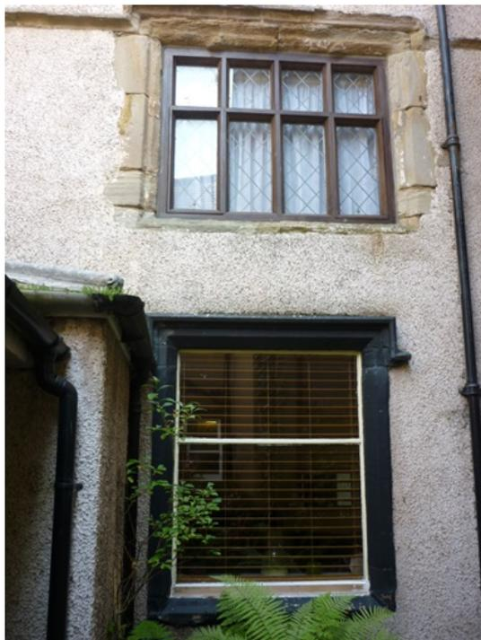
**Plate 82 (right): Windows with hood moulds on the east side of the courtyard**
