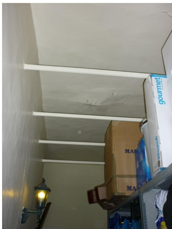
**Plate 76 (right): Iron bars in ceiling of room to east**
