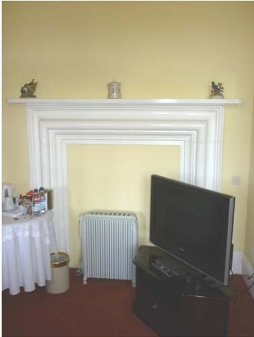
**Plate 77 (left): Bolection moulded fireplace on first floor**
