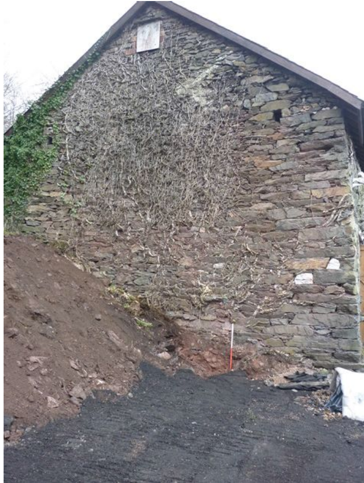
Plate 7: Haematite deposit staining the end of the charcoal barn, viewed from the south
