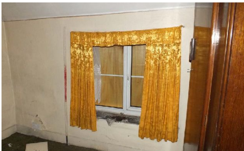
Plate 70: Window in the south-west elevation, Room F6, viewed from the north
