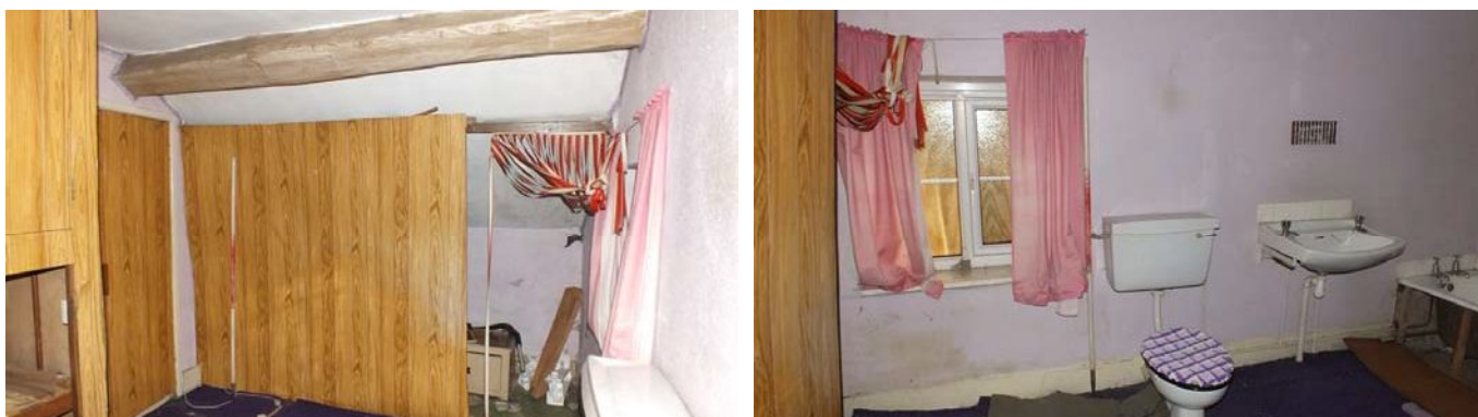
Plate 82 (left): General view of Room F10, viewed from the south-west
