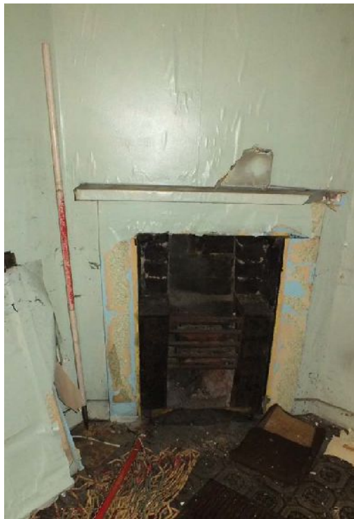
Plate 42: Fireplace in the north-west elevation, Room G7, viewed from the south
