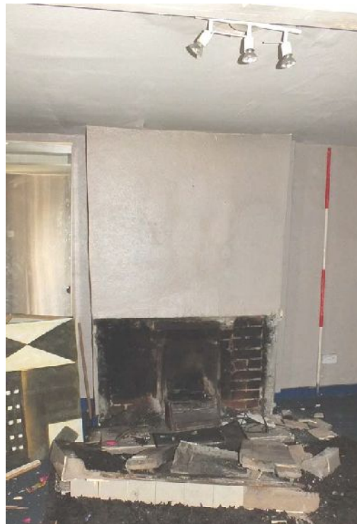
Plate 25: Fireplace in the north-west elevation, Room G2, viewed from the south-east
