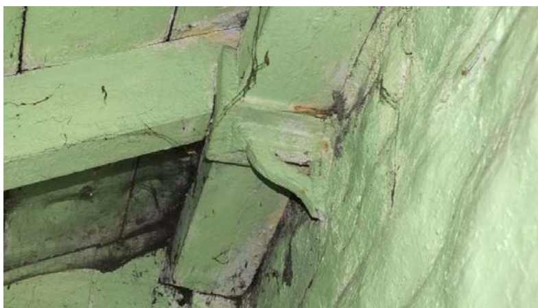
Plate 48 (left): Bracket supporting the beam against the north-west elevation, Room G9, viewed from the north-east
