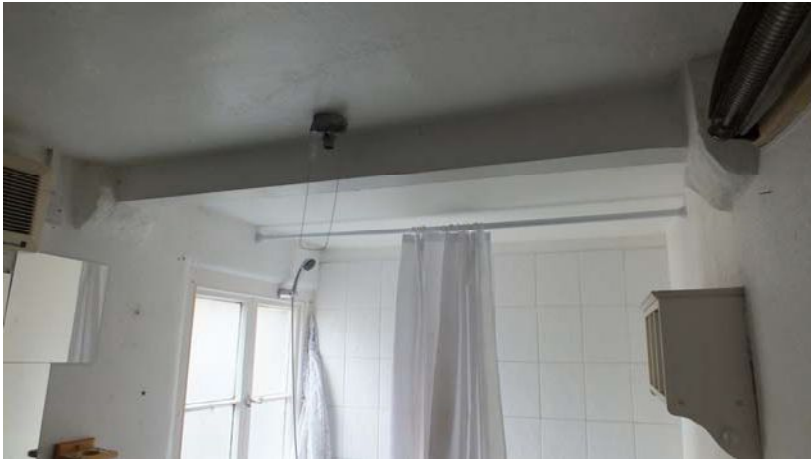
Plate 32 (left): Beam and corbels supporting the ceiling of Room G5, viewed from the west
