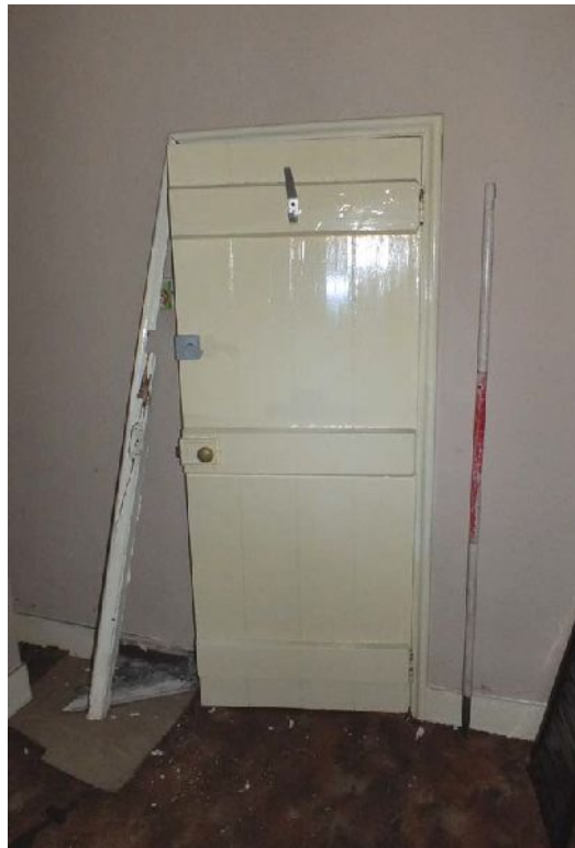
Plate 67: Door in the south-west elevation, Room F5, viewed from the north-east
