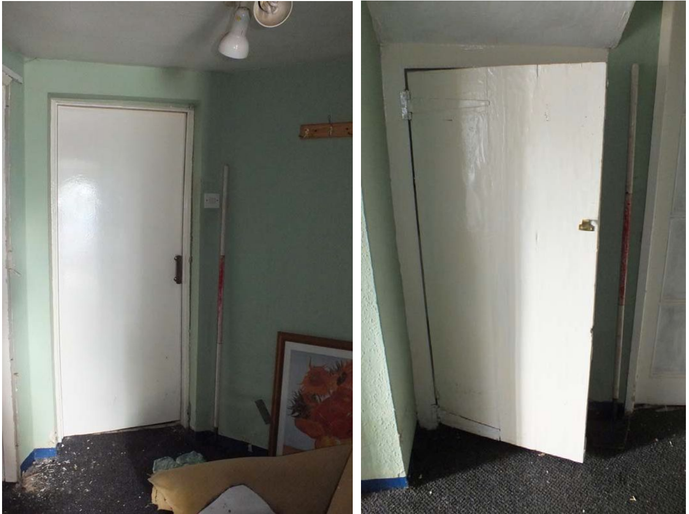
Plate 29 (left): North-east elevation, Room G4, viewed from the south-west
