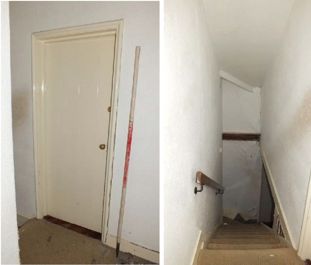
Plate 63 (left): Door to the north-east, Room F4, viewed from the south
