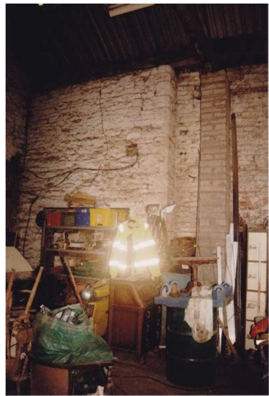
Plate 54 (right): West end of the north elevation of Room G3
