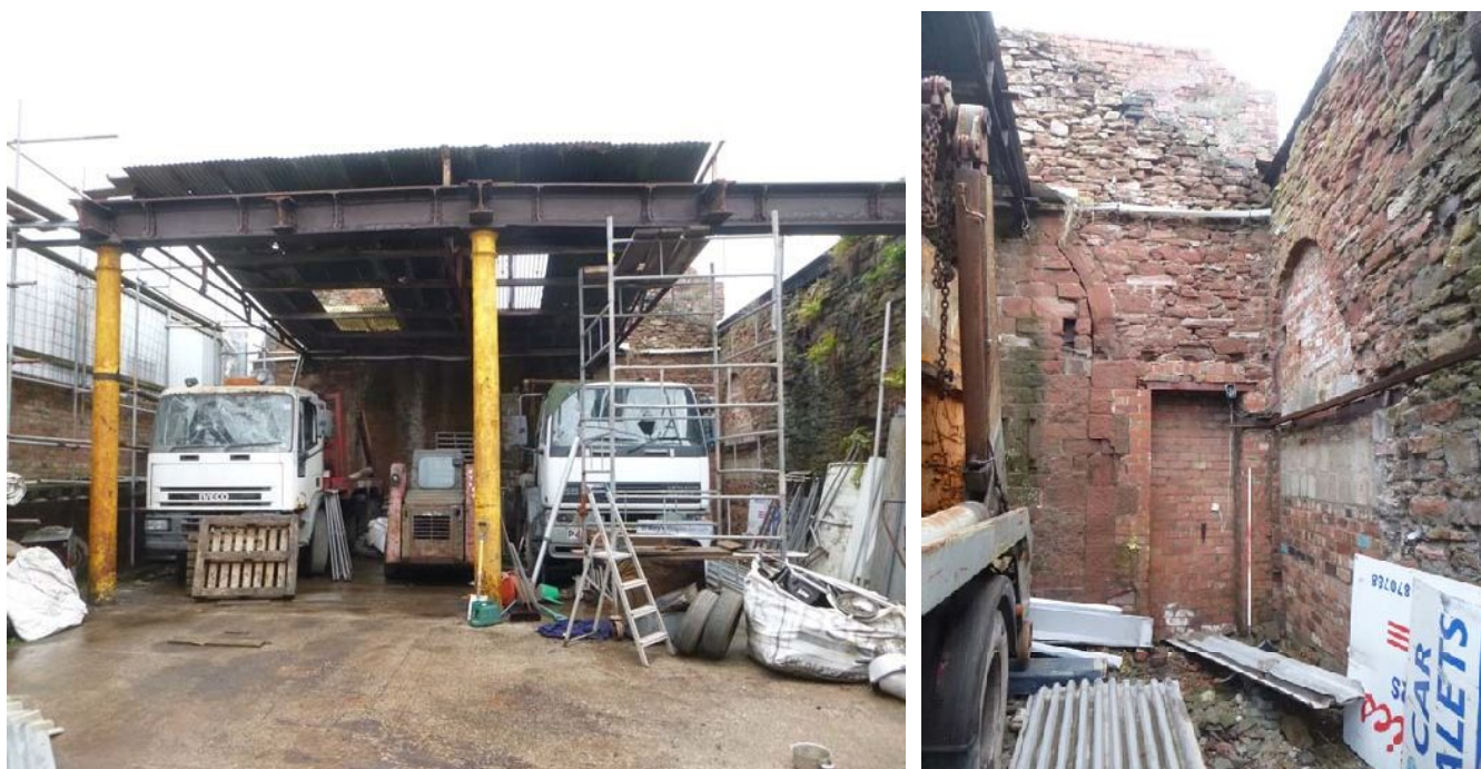
Plate 35 (left): North end of the east elevation of Room G1
