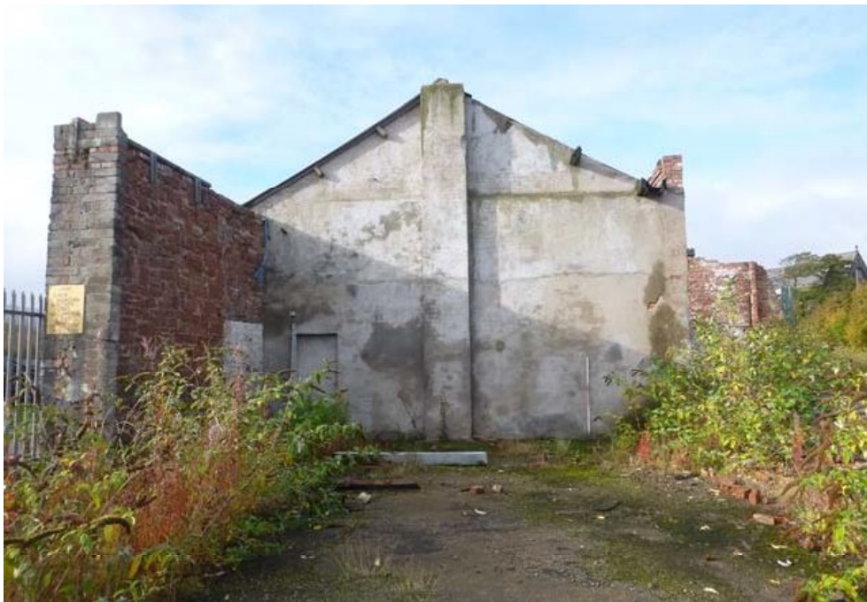
Plate 22: South end of the east external elevation
