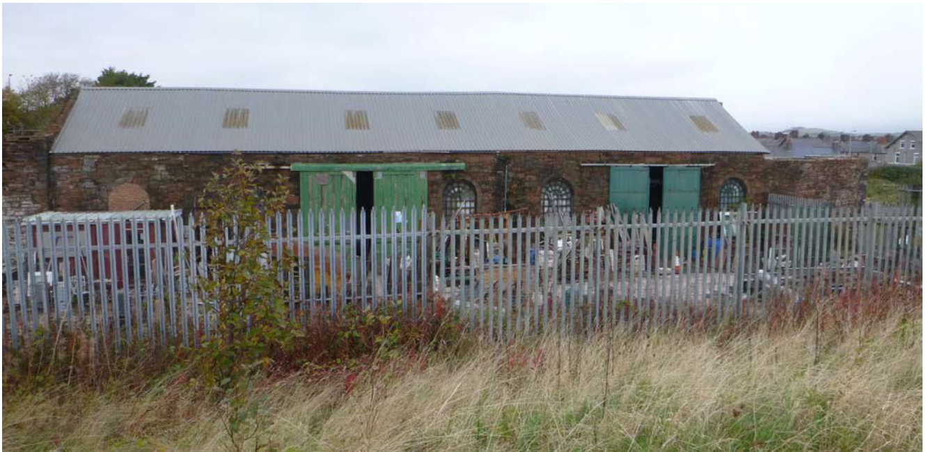
Plate 26: East end of the external south elevation
