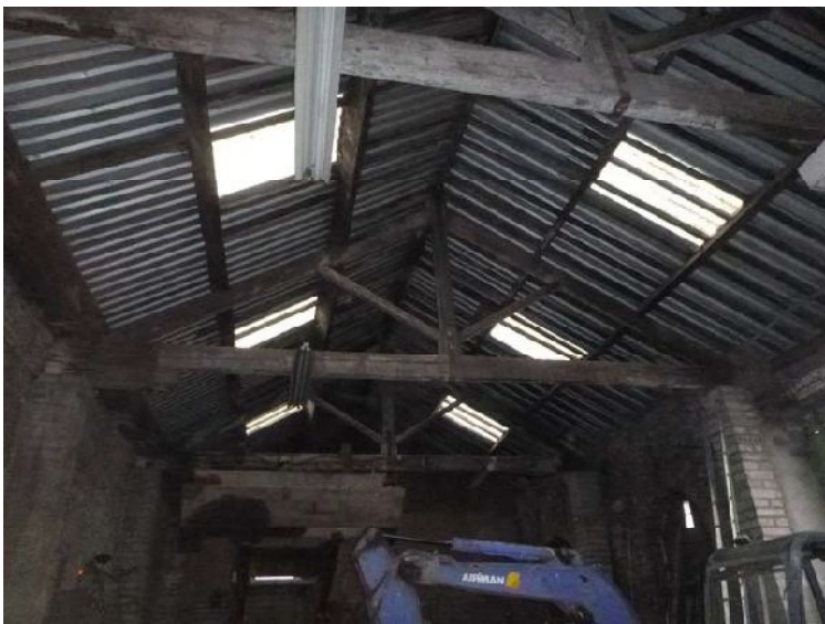
Plate 53 (left): Trusses in Room G3
