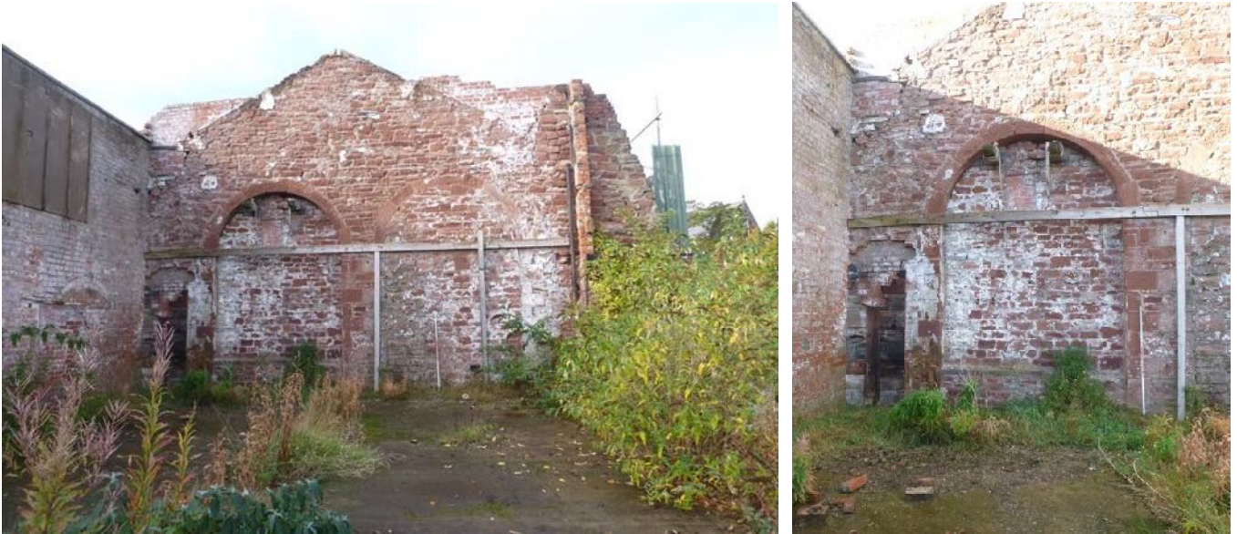
Plate 23 (left): North end of the east external elevation
