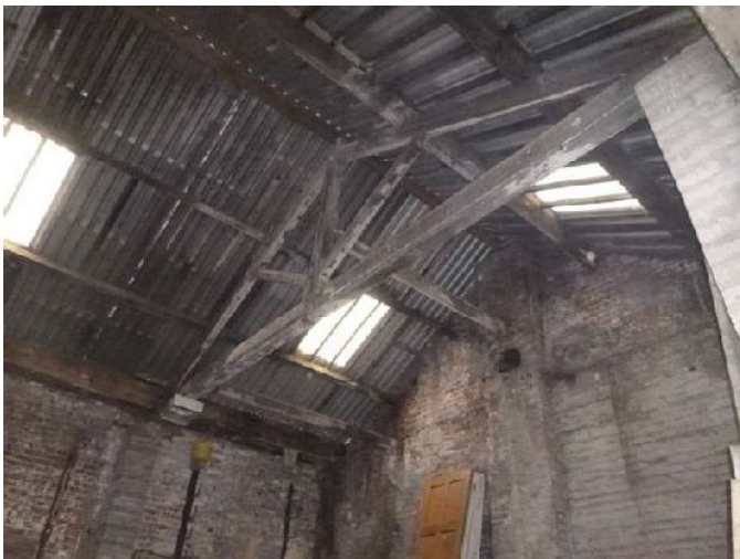
Plate 61 (left): Truss in Room G4
