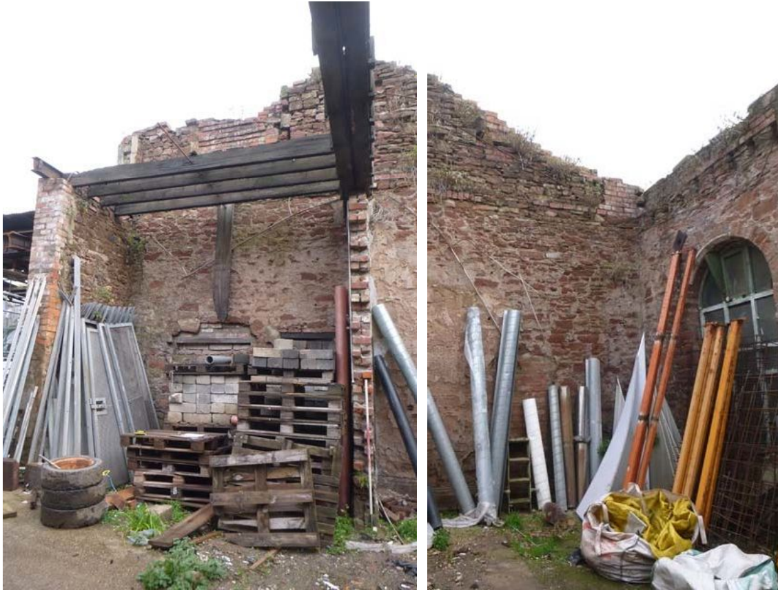
Plate 39 (left): South end of the east elevation of Room G1
