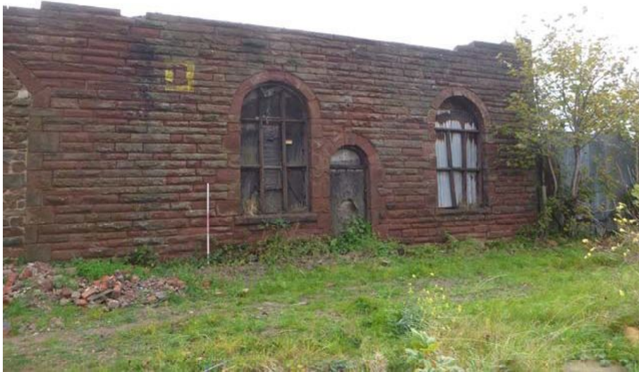
Plate 21: South end of the west external elevation
