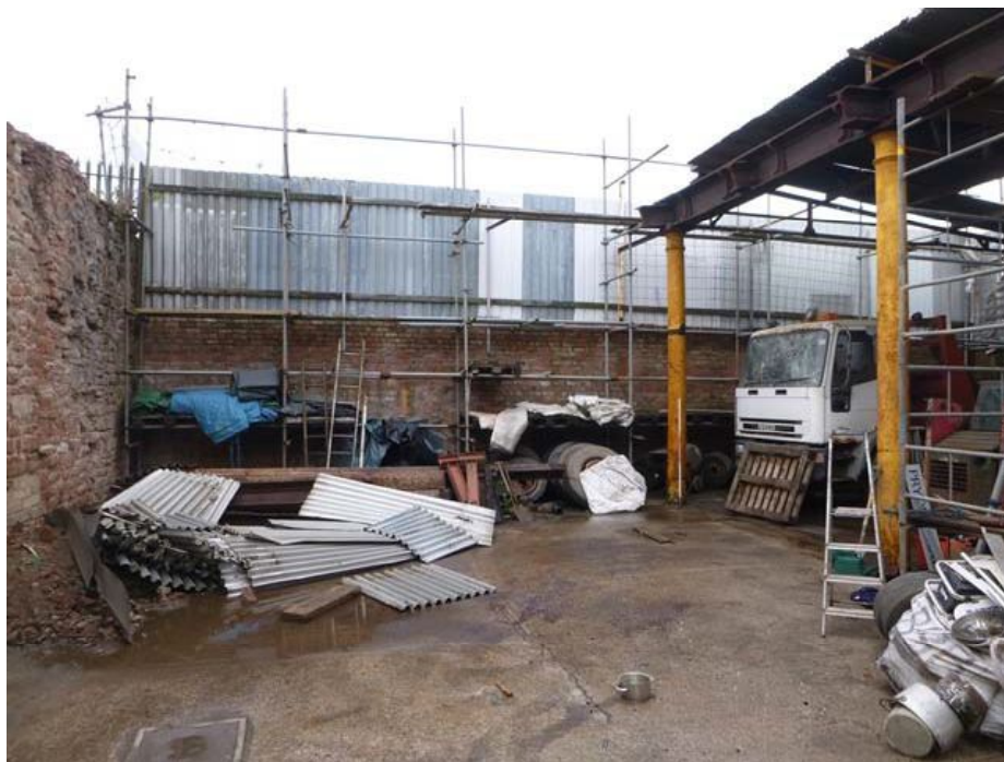
Plate 34: North elevation of Room G1
