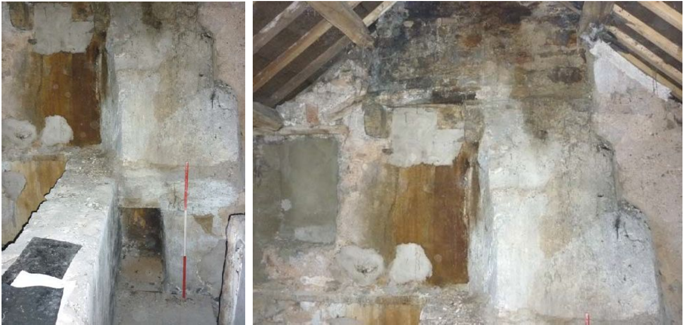
Plate 65 (left): Chimney breast to the north of the 'spine' wall
