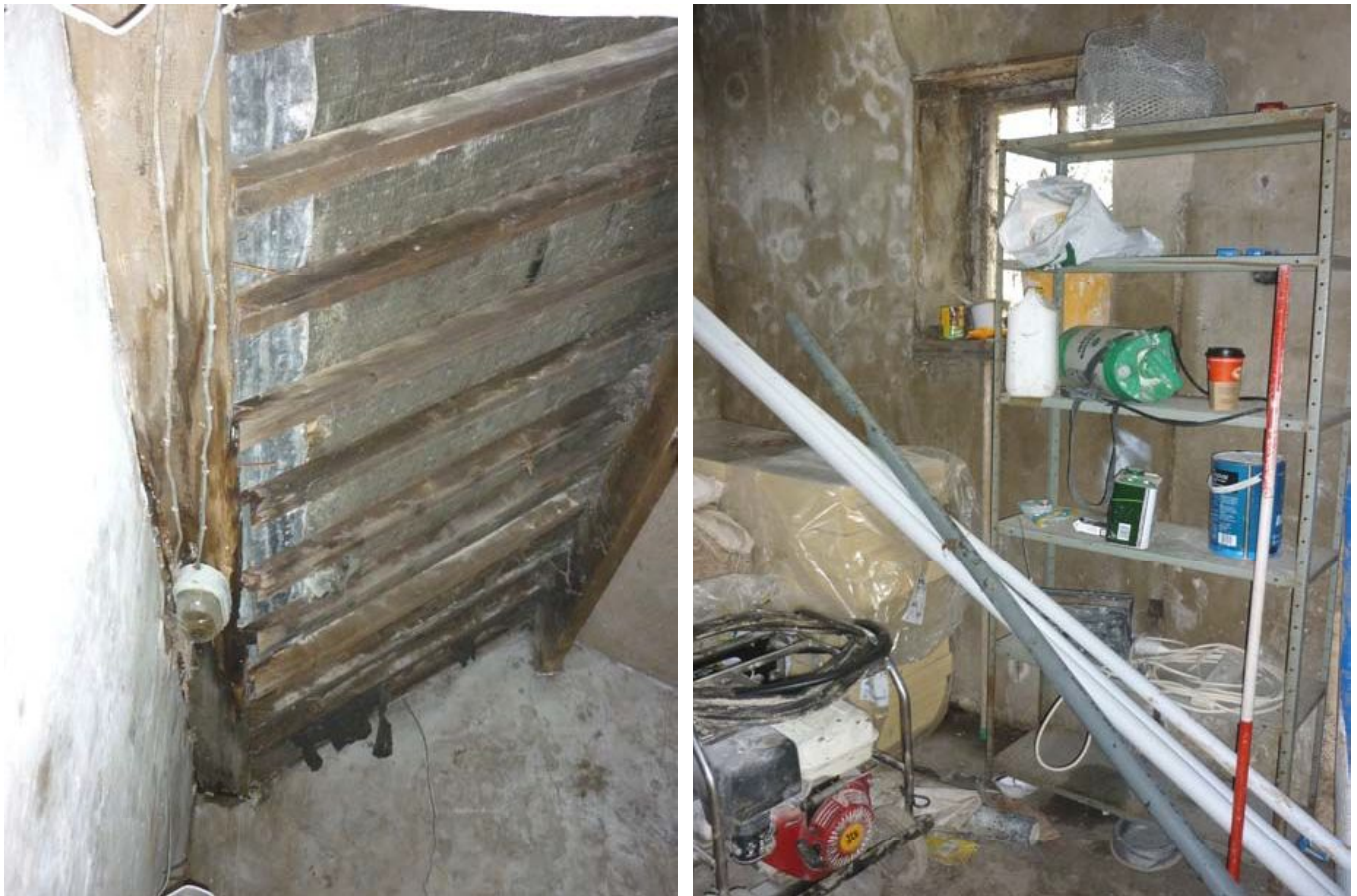
Plate 20 (left): Machine cut rafters along the south wall of Ground Floor Room 1
