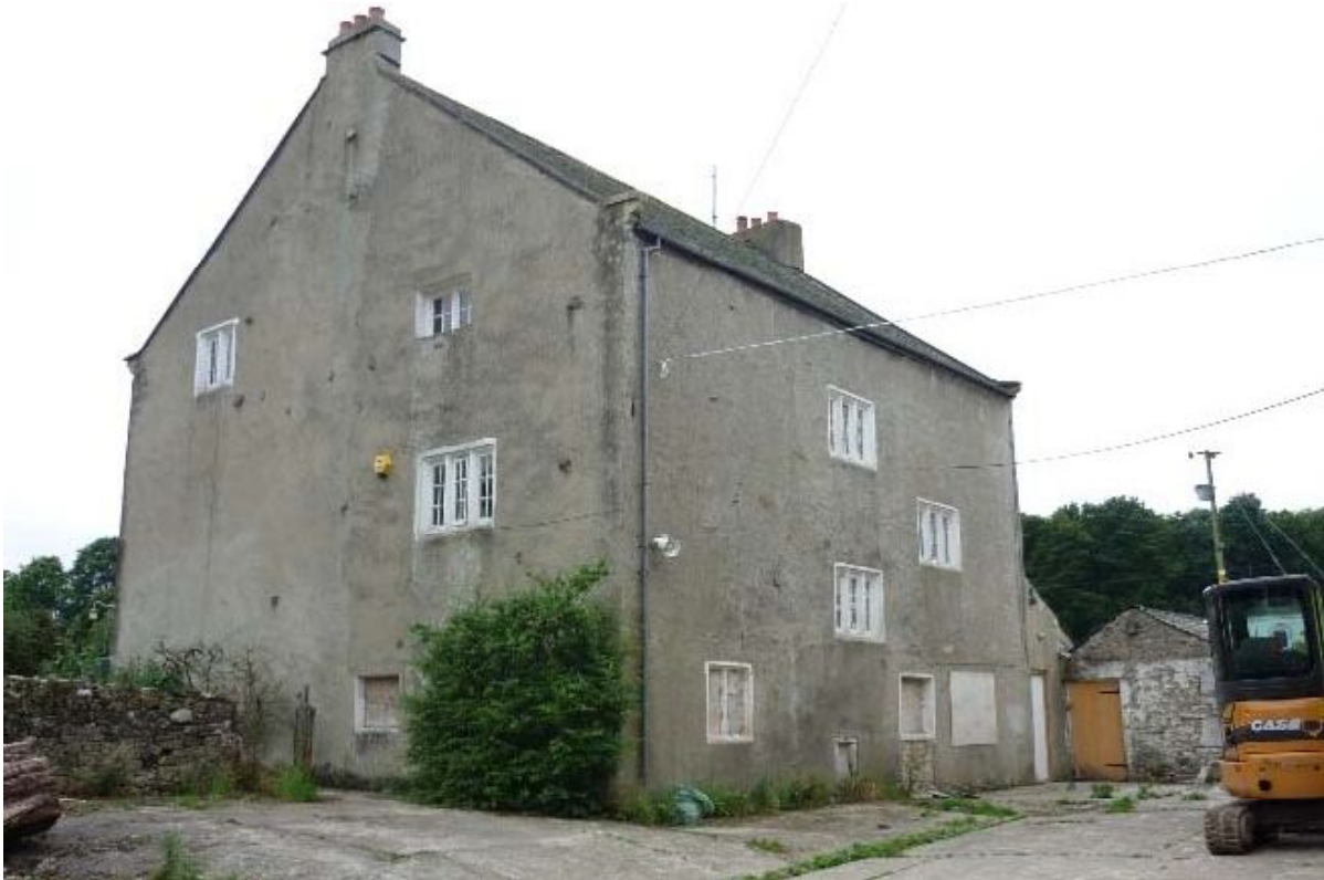
Plate 5: North and east external elevations of the house and outshuts
