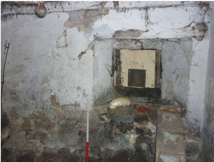
Plate 16 (left): North elevation of the cellar
