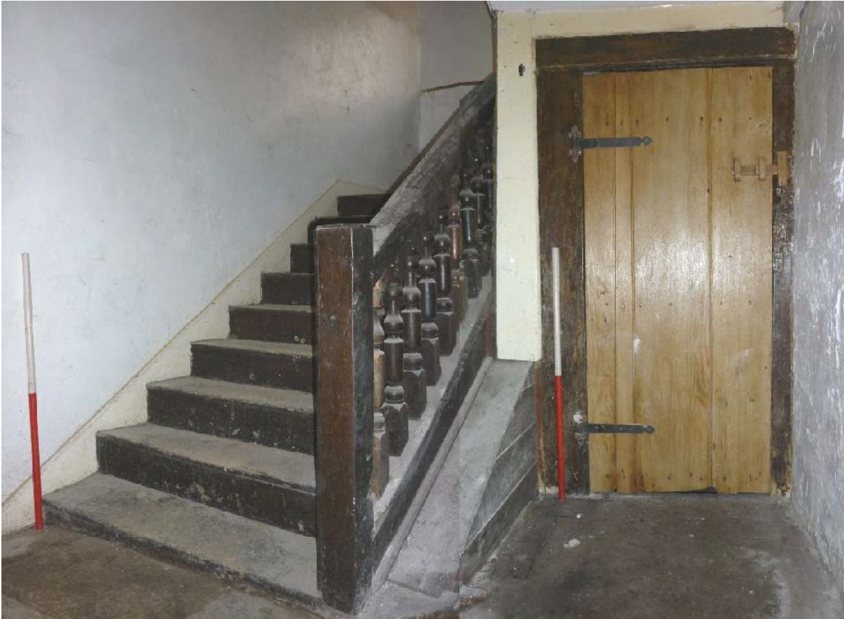
Plate 32: Composite photograph of the stairs, viewed from the ground floor
