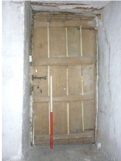
Plate 57: Door in the north elevation of Second Floor Room 2
