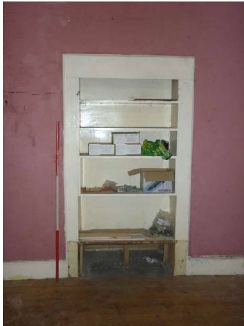
Plate 36: Cupboards on the west elevation of Ground Floor Room 6
