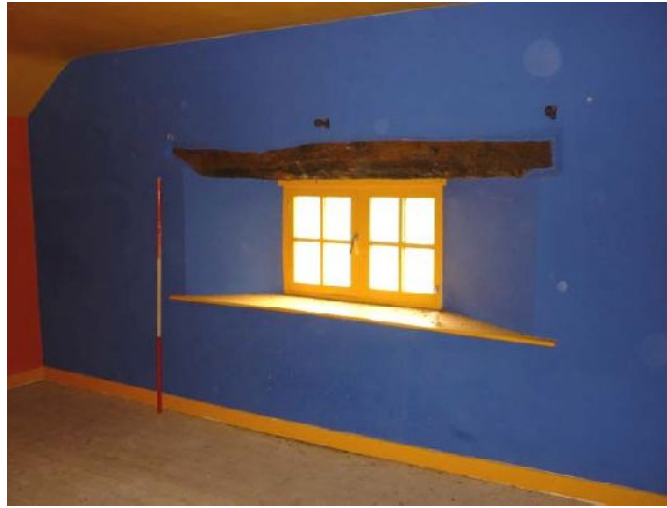
Plate 62: East elevation of Second Floor Room 5
