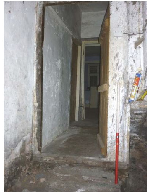
Plate 17 (right): Doorway in the south elevation of the cellar
