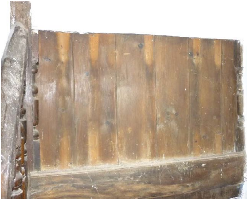
Plate 58 (left): Tongue and groove beaded planks to the west side of the stairs viewed from
