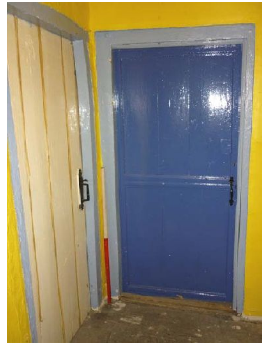
Plate 58 (left): Tongue and groove beaded planks to the west side of the stairs viewed from
