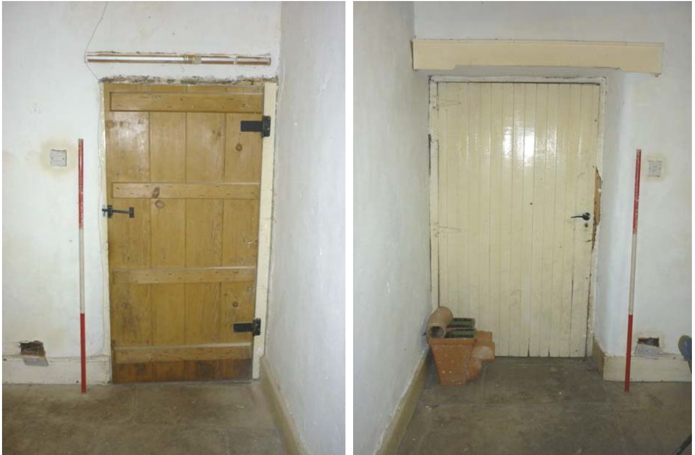
Plate 28 (left): Doorway in the north elevation of Ground Floor Room 4
