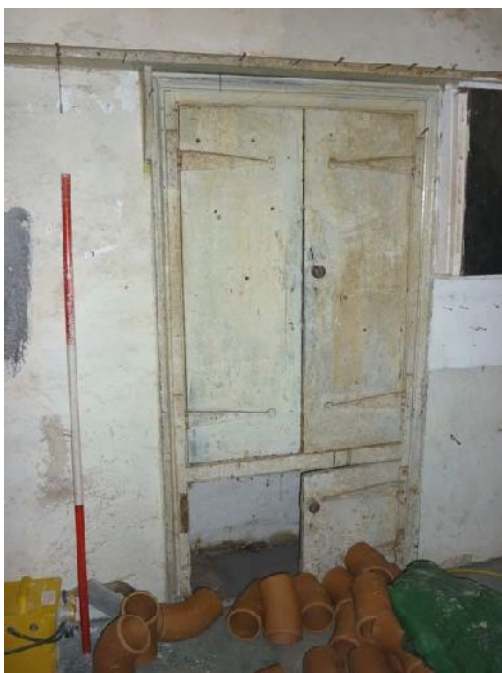
Plate 39: Cupboard in the west elevation of Ground Floor Room 7
