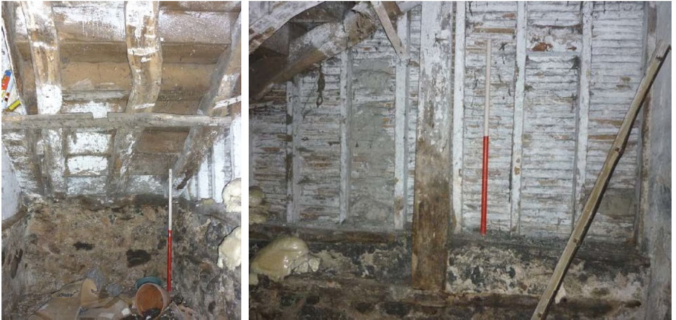
Plate 18 (left): Underside of the stairs from in the cellar
