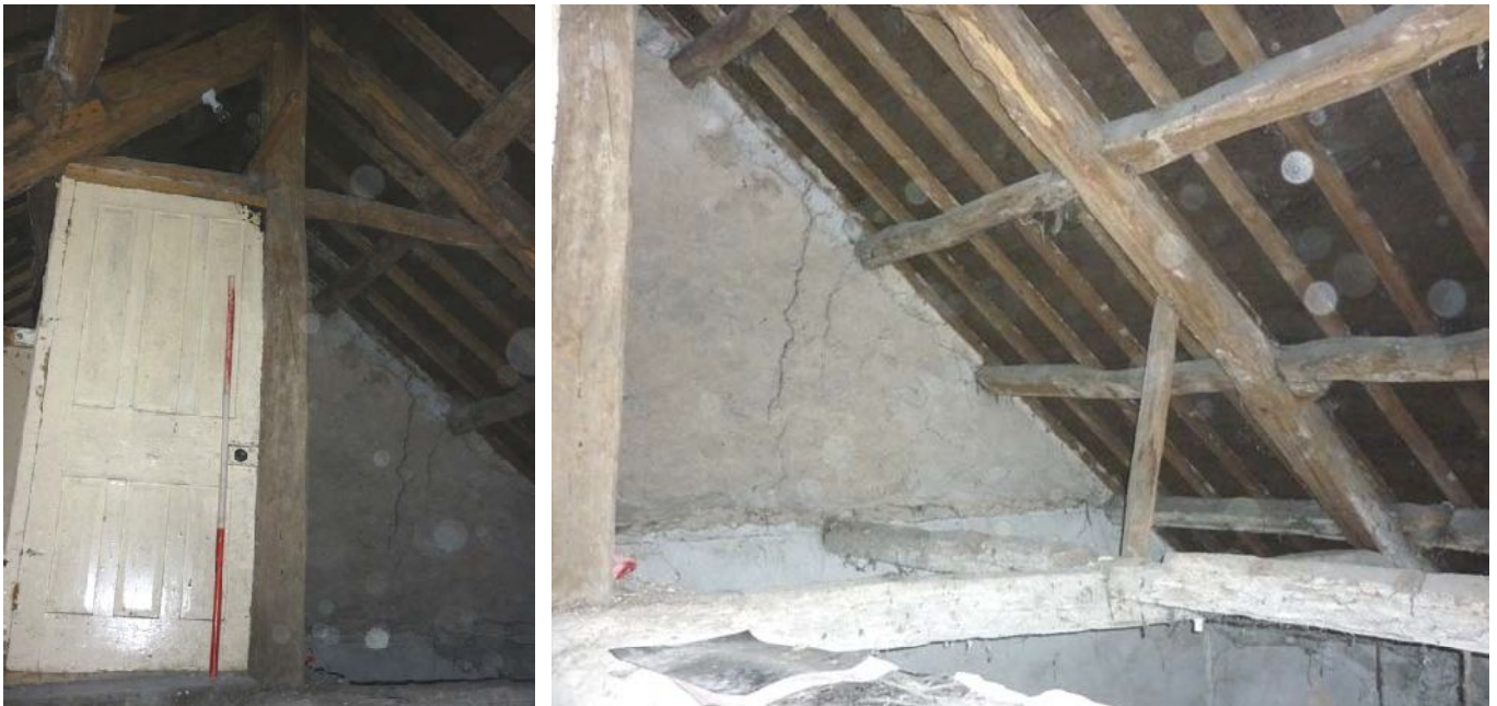
Plate 63 (left): King post truss and upper collar
