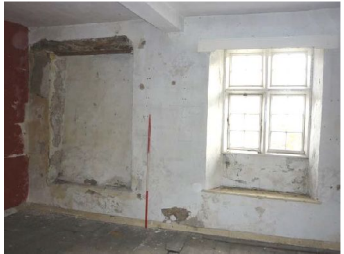
Plate 50 (left): Fireplace in the east elevation of First Floor Room 5
